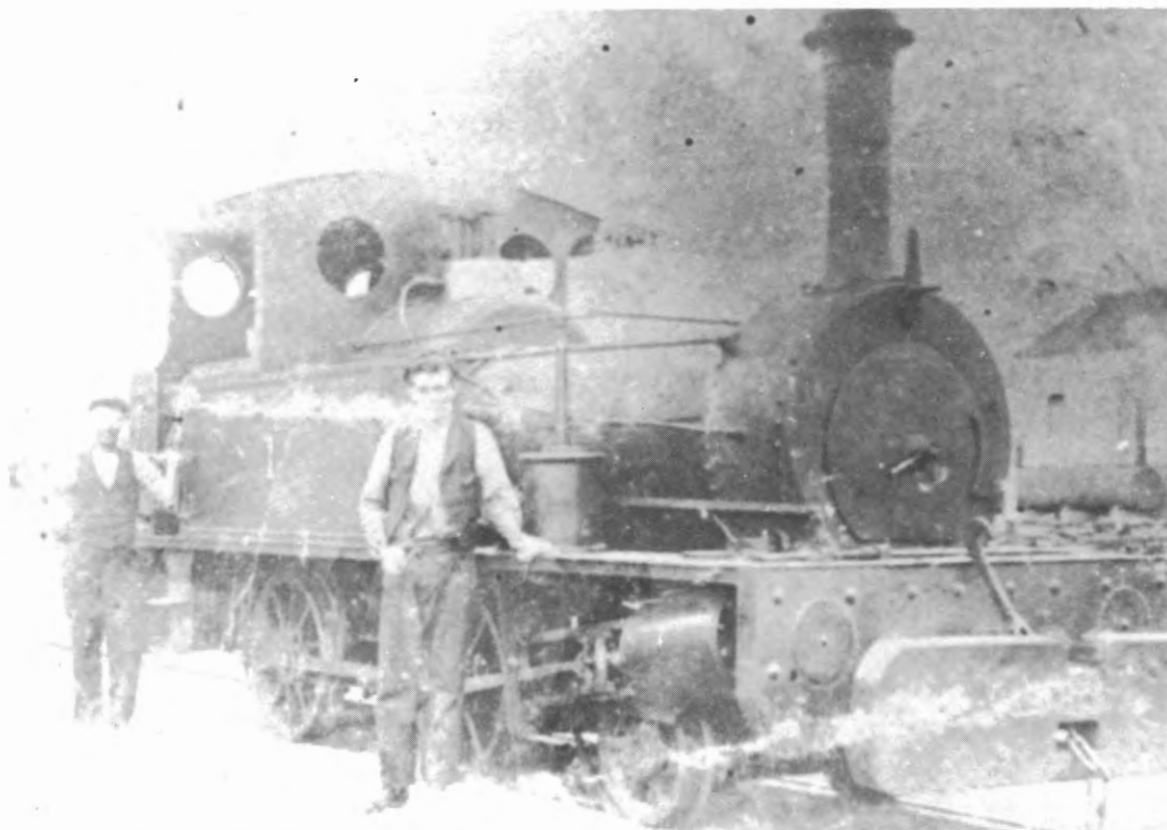
Above The Moonta Dubs rebuilt to 3ft 6in gauge and fitted with a Hudswell Clarke boiler.
