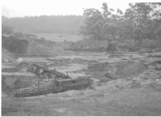
Jerry Platt was on hand to photograph the archaeological dig at the old Mittagong Ironworks site during the open day on 5 November 2005. A large T-shaped structure dominates the remnants. At the top of the Tee is the deep pit wherein sat the flywheel of the rolling mill engine. The foundations of the rolling mill stands are at the leg of the Tee. The flywheel pit foundations were very deep and made of massive blocks of sandstone laid across one another. North of the flywheel pit is another 'hole', wherein sat the helve hammer for knocking puddles blooms into shape and also for forge welding smaller billets into larger ones.
