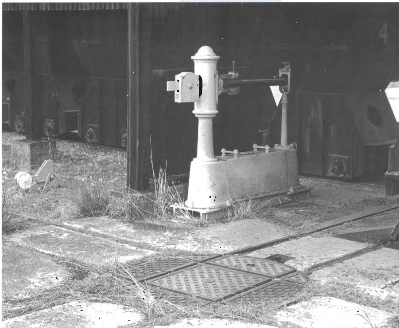
A view of the weighbridge and turntable at the western end of the Skip Truck Shelter, Acid Section, 1972.
