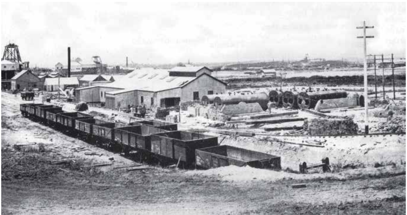
State Coal Mine Power House under construction in 1911. The bricks for its construction came from the State Brickworks. In this scene the brick foundations for the boilers are well underway. The 2ft gauge tramway that carried bricks to the site can be seen in the middle of the scene with a bogie truck ready to be unloaded.
