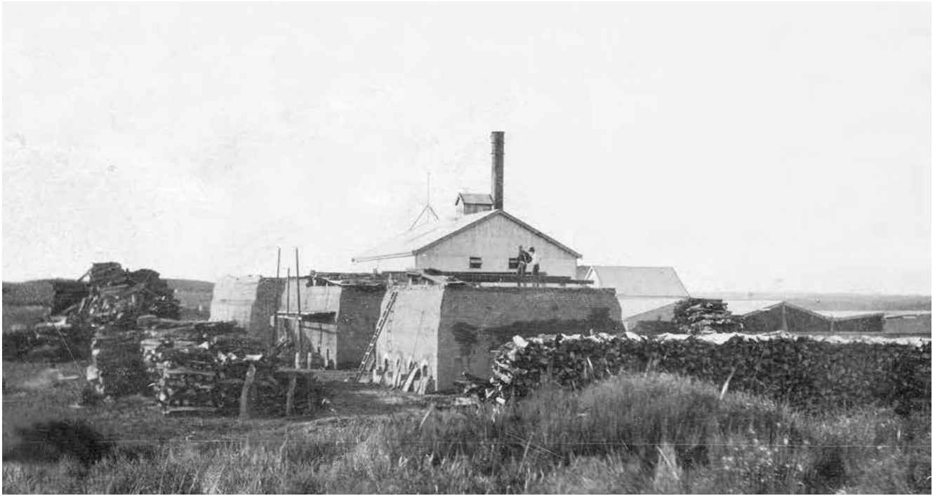
The Scotch kilns around August 1911 viewed from the west. The closest structure was a single kiln while the two further away comprised two kilns in each structure. The move from using the local coal to firewood has happened Photo: Wonthaggi Historical Society
