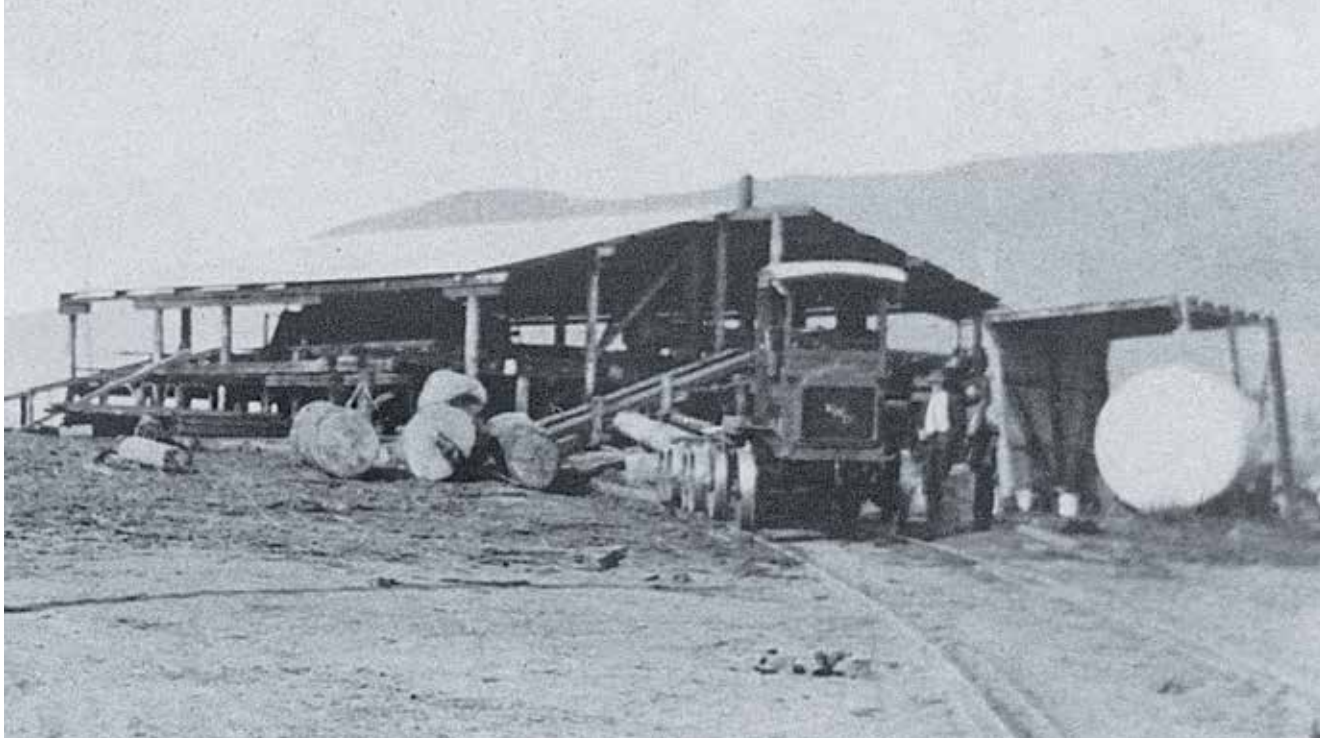
The Rhodes Timber Company's standard-gauge FWD rail lorry on the log siding in front of the company's first sawmill at Mount George. The American-made four wheel drive successfully hauled logs to the mill over the lightly-graded Woolshed Creek line between 1921 and 1925. When the logging tramway was extended up Knodingbul Ridge in 1925 the FWD did not have enough tractive effort to cope with the 1:10 and 1:7½ grades and was replaced by Nattrass Rail Tractors. Photo: ARHS Photo 931
