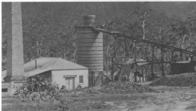
Among the early photographs of the Eskbank Ironworks located in the Powerhouse Museum collection is this 1877 scene of the blast furnace being rebuilt. The brick wall for the new heating stove is evident at the base of the blast furnace, while a crude 'lean to' protects the winding apparatus that operated the wagon on the inclined charging tramway. The engine house and chimneystack are on the left.
