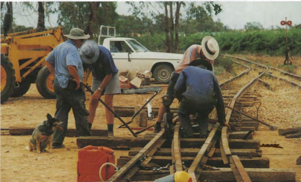
Volunteer workers install a sleeper at the Cobdogla steam railway. The 'site manager', Cody the dog, keeps a watchful eye on the proceedings. Note the SAR switch stand on the right. Photo: Brian Grayson
