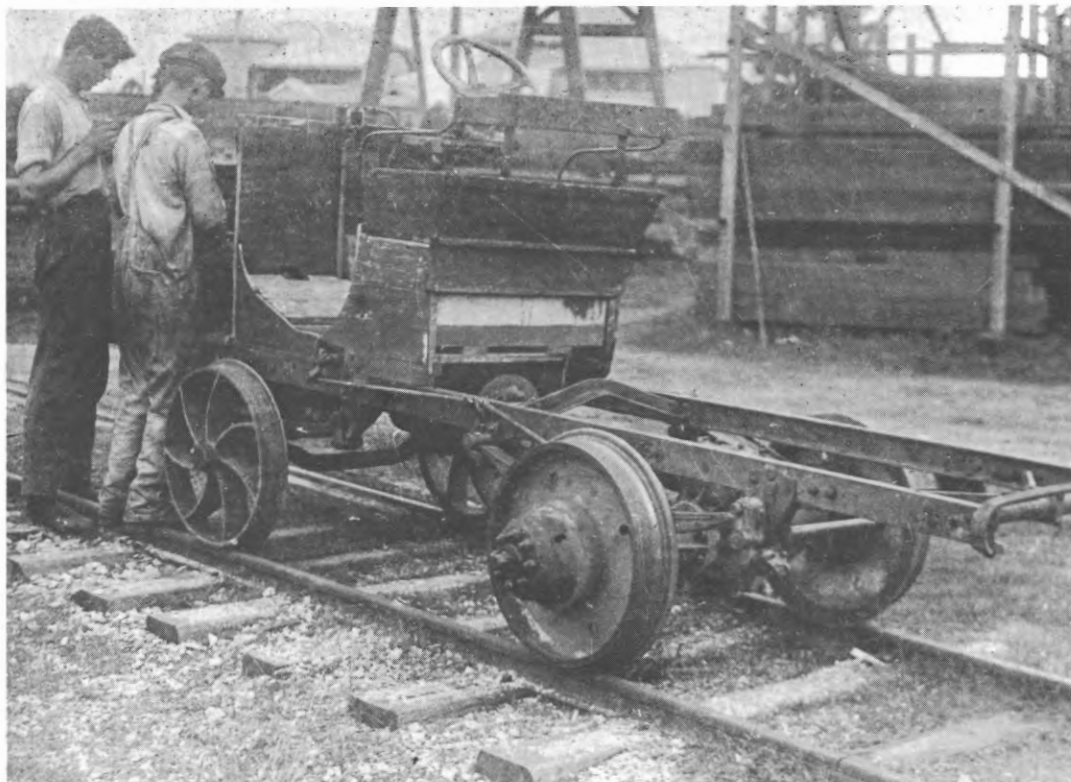
Two views of the railcar which had been converted from an old Commer truck.
