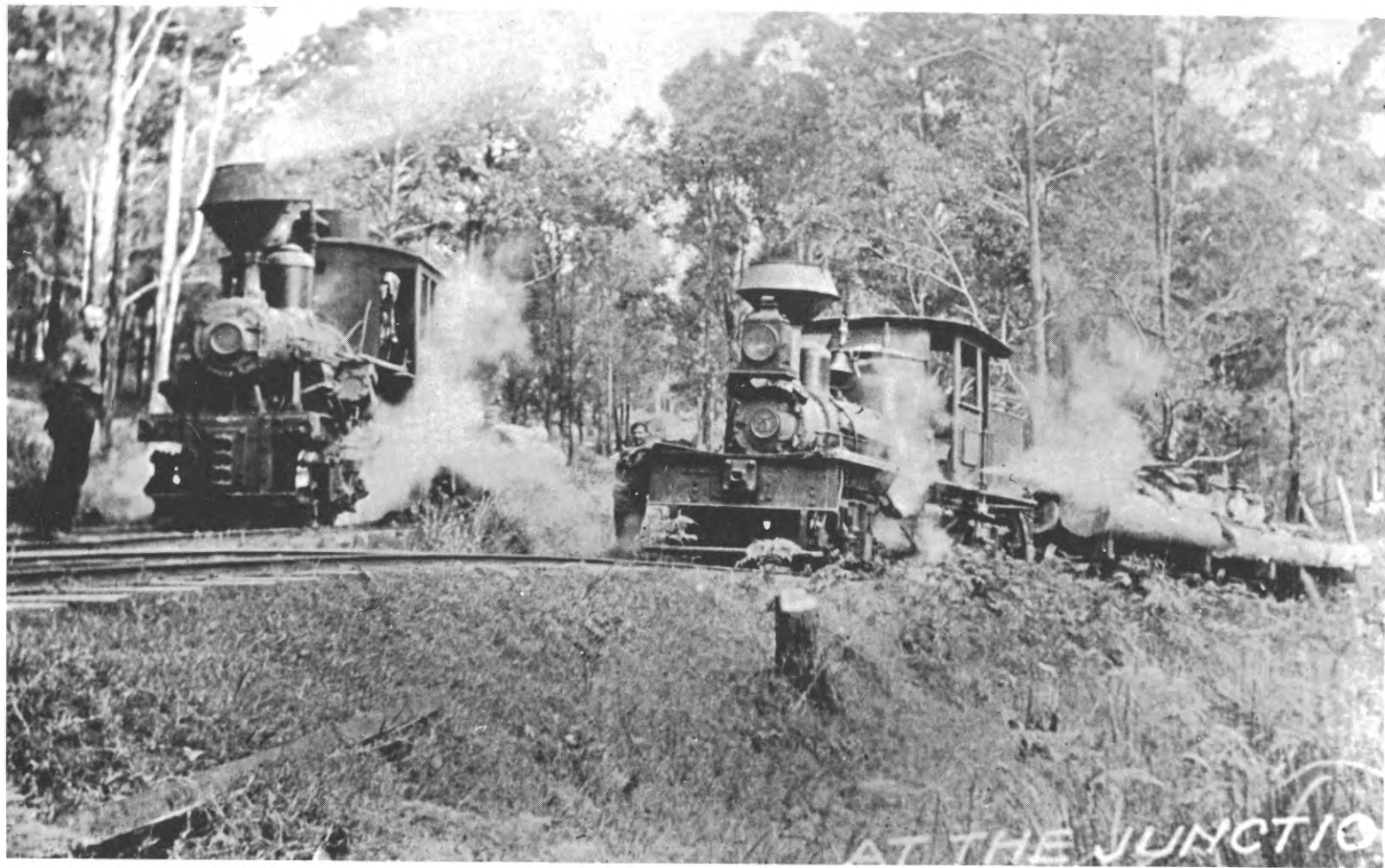
The Climax and ex-North Mount Lyell Shay (still with its bell and headlamp) meet at one of the junctions on Lahey's tramway.
