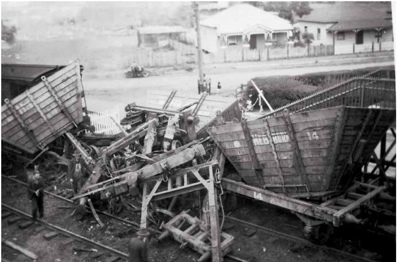
'Self Destruction'. Wooden coal hoppers certainly came to grief in a spectacular manner. This is the 1942 accident referred to in the text. The photo, taken from the High Street Station footbridge, Maitland, includes the wreckage of seven Hebburn coal hoppers and a van. Photo: John Parker Collection
