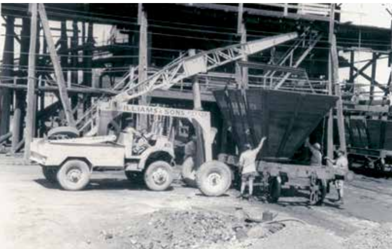
Left: "Saturday Shift". With the advent of the Dyke ship loader, the Railways Department required that all waggon brake levers be on the same side. Here at Maitland Main Colliery, one Saturday in 1969, the two waggon repairers, the carpenter and the shunter, spend an overtime shift turning waggons. One more job to keep the Department at bay. Photo: Author
