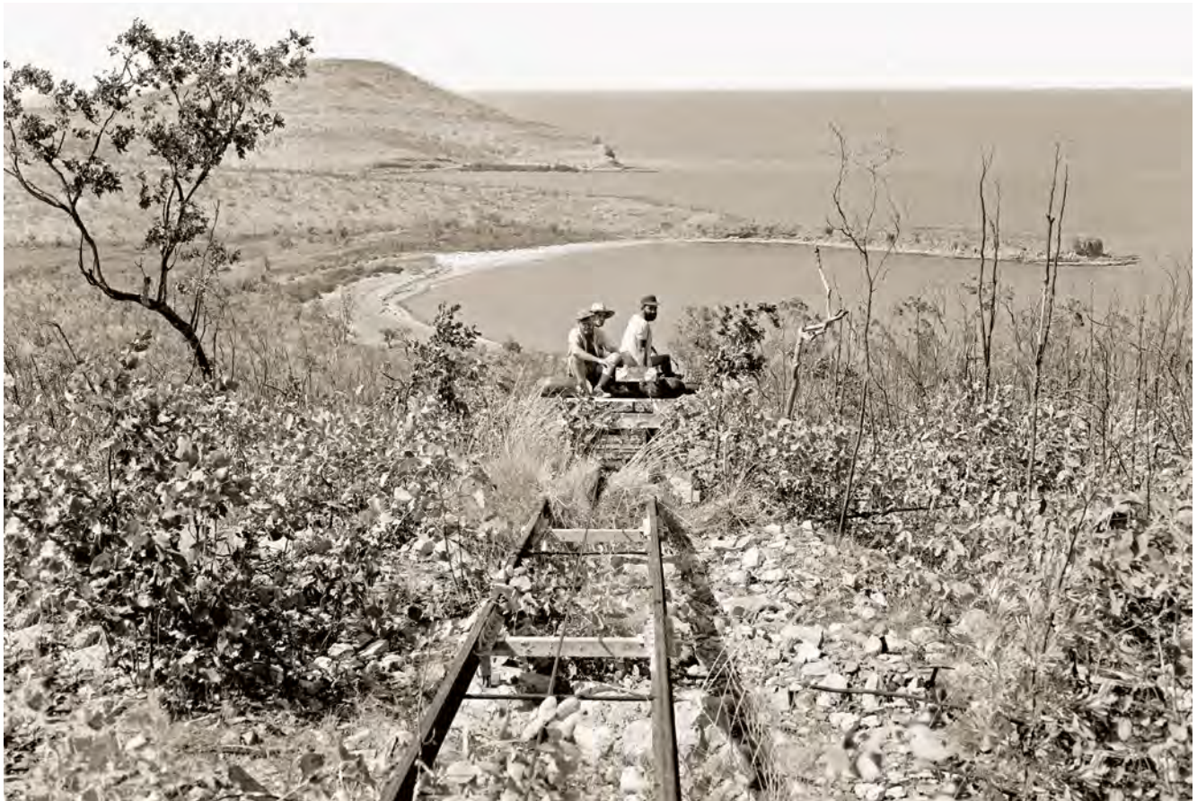
The winch driver's view, looking s-s-e from the top of the incline as the loaded trolley comes into view and nears the last cable roller between the rails. Turtle Bay is the nearest of the two bays. In the far distance is the coast line on the eastern side of Cambridge Gulf. Dated 1963, the re-growth of grasses in the three years since the line was built is apparent as is the scrubby tree cover and rocky nature of the ground. The MV Cape Don is out of picture, to the right, off Turtle Bay.
