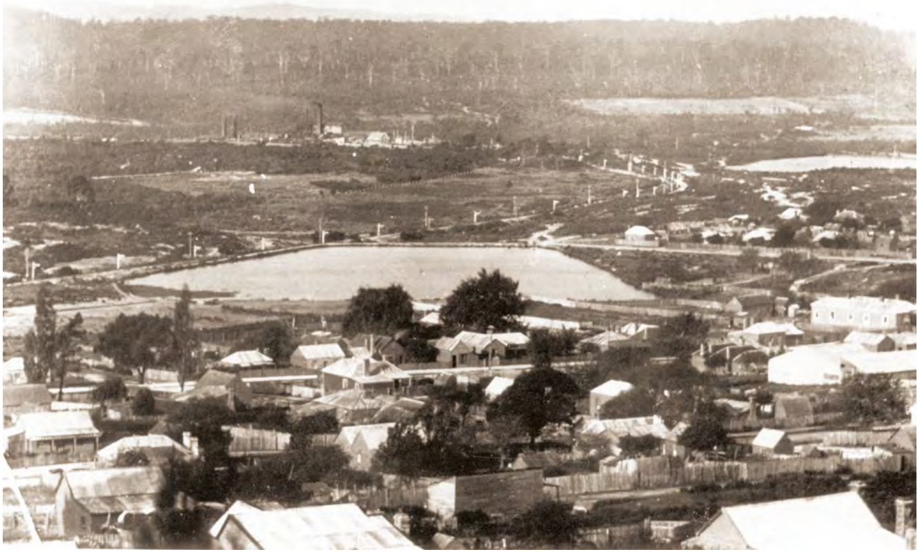
Above: Undated view of the route of the overhead wire electric railway marked by the bright white painted support posts. Photo: Beaconsfield Mine & Heritage Centre collection. Left: Piece of rail recovered from the site of the gold mine battery, so quite possibly from the tramway. The rail measures 1\frac{3}{4} in high x 1 in wide across the head x 2in wide across the bottom flange which would equate to roughly 12-14 lb/yd. The black and white squares measure 10 mm x 10 mm each. Photo: Beaconsfield Mine & Heritage Centre collection. Below: Robert Hudson Ltd V skip and V skip frame on display at the Beaconsfield Mine & Heritage Centre. Photo: Beaconsfield Mine & Heritage Centre collection.
