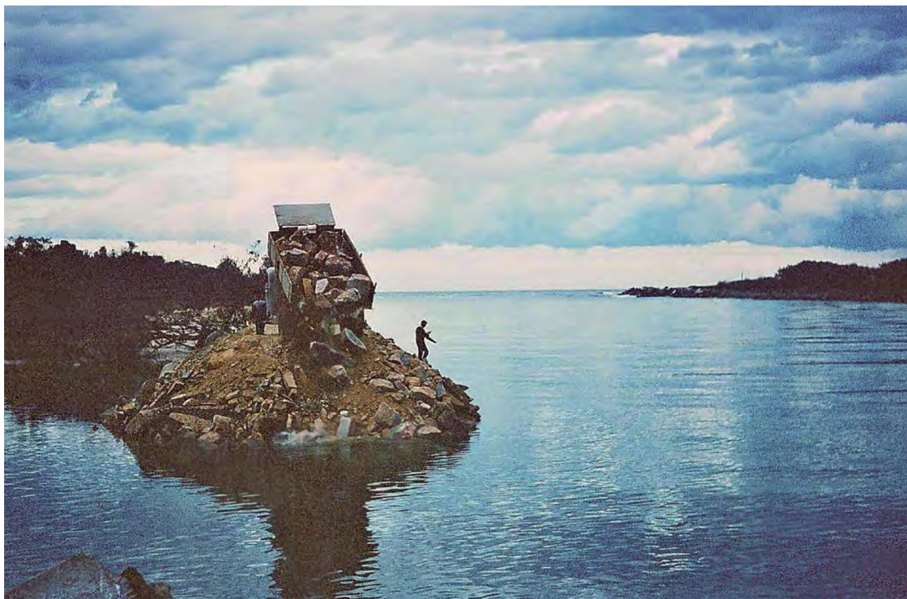
The North Training Wall was extended a short distance upriver when the ocean breakwaters were constructed between 1968 and 1972. Laurieton Quarry was re-opened to supply stone but this time road trucks were used to haul and dump stone. The south breakwater at the river entrance can be seen in the distance.
