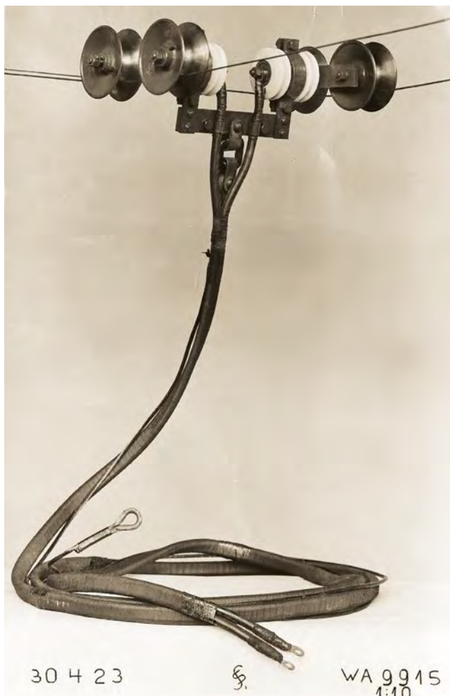
The electrical collector running along the overhead wires, and flexible lead, supplying electric power to the locomotive possibly looked something like the above. Photo: Wolfgang collection
