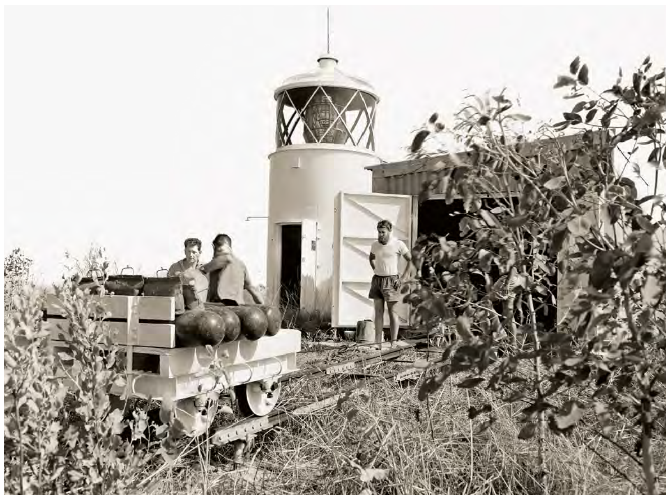
The trolley at the top. Four heavy cylinders of acetylene gas and other supplies need to be unloaded. Four men were usually required to manhandle each cylinder into the light tower. The 45 lb/yd rail is in ten-foot sections between vertical supports, with two steel tie rods in each section of track. The heavy 6-hole fishplates seem rather excessive for the task. Photo: National Archives of Australia A1200, L45685
