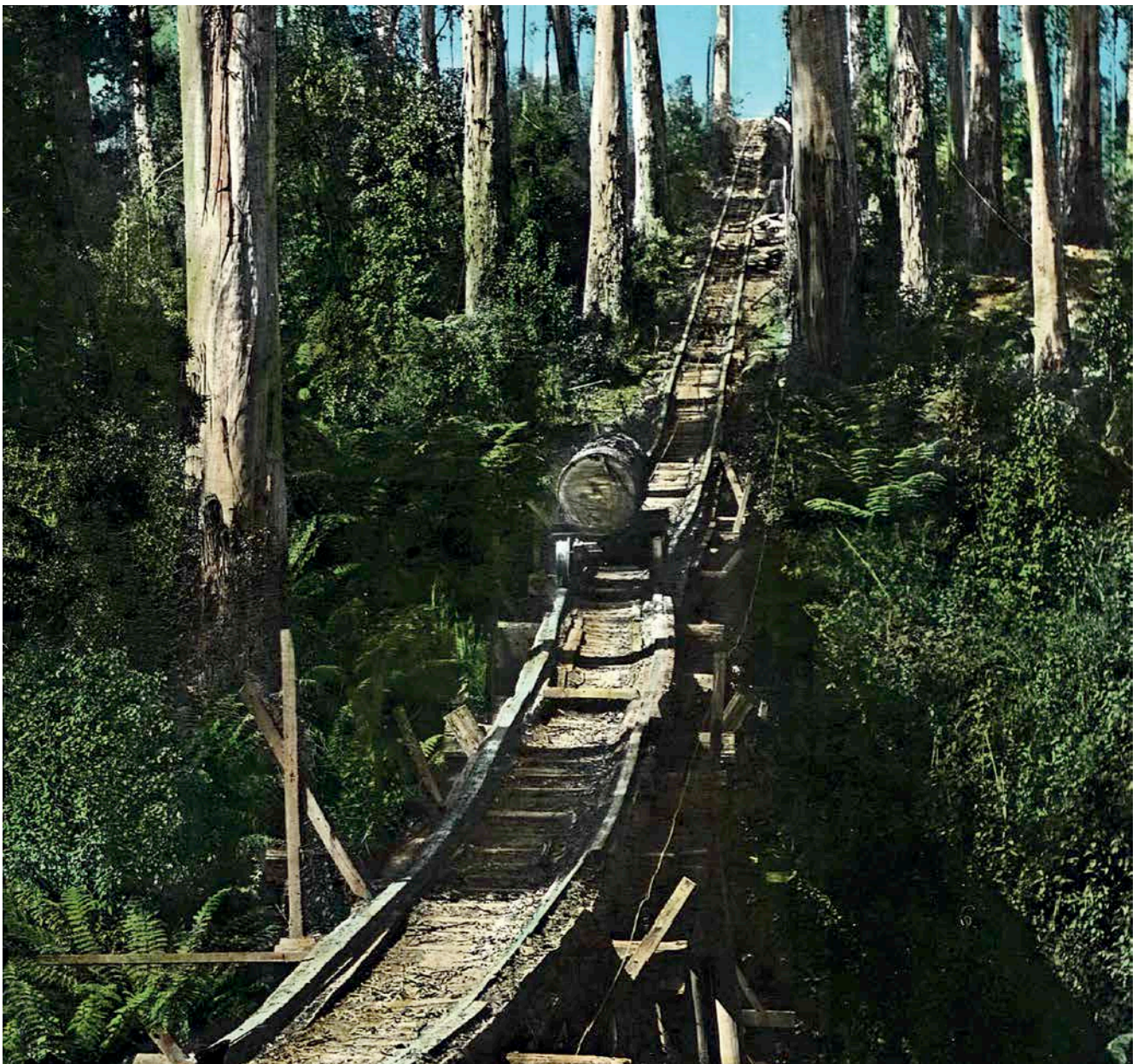
Above: Hauling a log up to the Elliott River mill. Note that the tinter has omitted the very top of the incline and turned it into sky! The bridge over the Elliott River has incurred a sideways kink when compared with earlier photographs (see Sawdust and Steam , Norman Houghton, 2010). Both timber and steel strap rails seems to be in evidence. Note towards the bottom left of the bridge the wooden upright which has been attached - this was probably to keep the cable in place when going round the curve. And on the right hand side of the bridge is either a telephone line or whistle rope to communicate between the bottom and top of the incline. Photo: National Library of Australia obj-142426403
