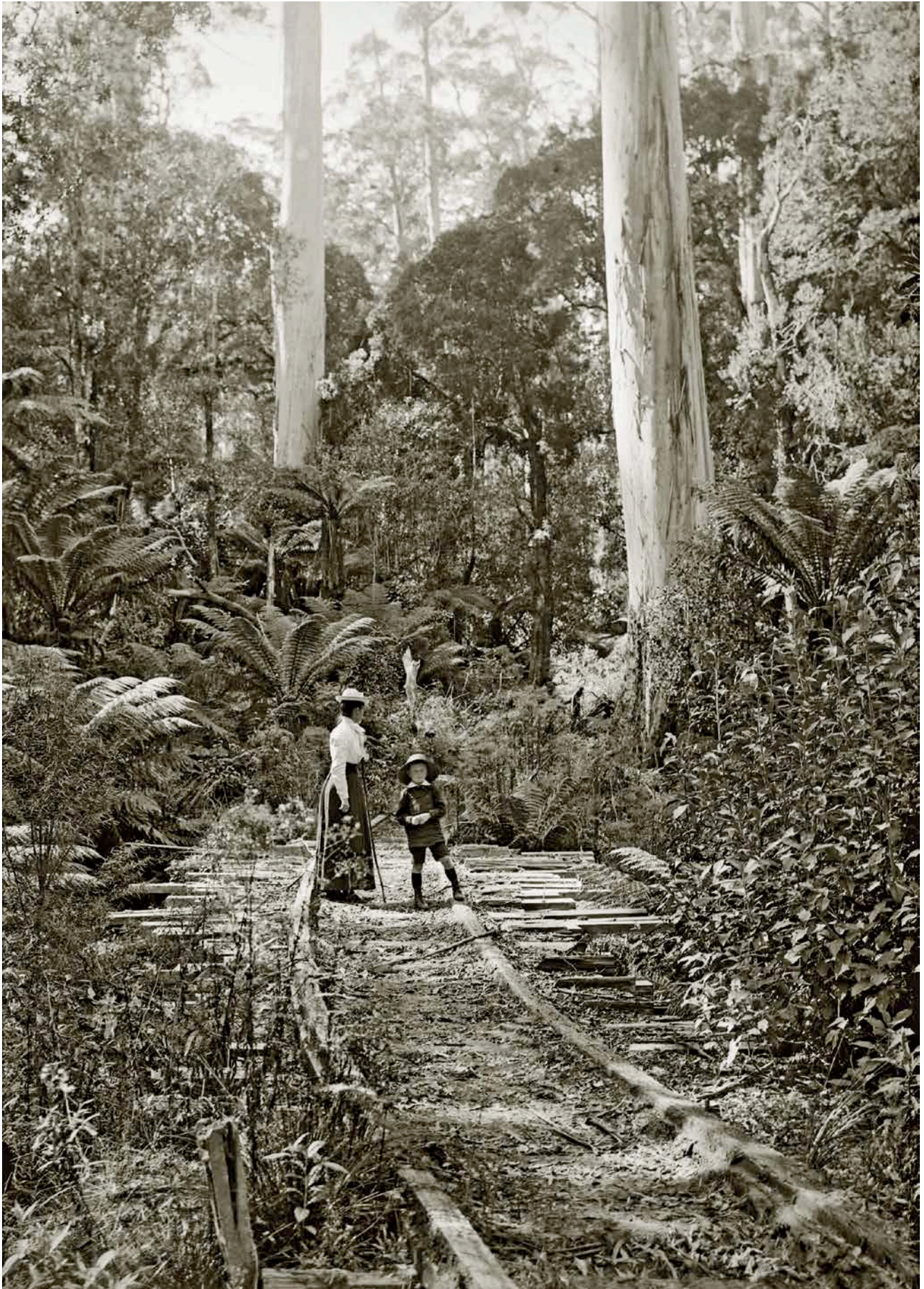
Above: A disused logging tramway. Various owners of the Elliott mill invested much capital, trying to make it a 'goer'. The last of them, in 1907, was Henry Teesdale Smith (not as sometimes said, Millars' Karri & Jarrah Company – Smith had 'retired' from that company). Despite employing well-known sawmiller Alexander Clark Mackay as manager, Teesdale Smith also failed to make the venture profitable. Photo: State Library of Victoria H2011.40/16
