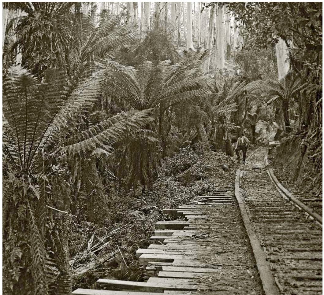
Right: 'On the Saw Mill Tram, Apollo Bay' is the title Harvey assigned to this carefully composed photo. Judging by the well-used tram track it is the main tramway from the jetty at Apollo Bay to the Elliott River mill. The camera has been set up on a fully decked bridge in a well-shaded gully. The actual rails seem to have been recently re-laid and the bridge re-decked. Photo: State Library of Victoria H90.161/52
