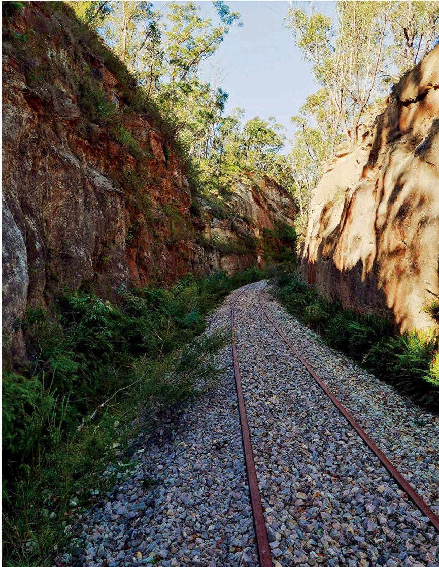
The restored line between Clarence station and Newnes Junction. The line passes through several deep cuttings and makes for a spectacular journey to where it stops just short of the road to the mine at Newnes Junction.
