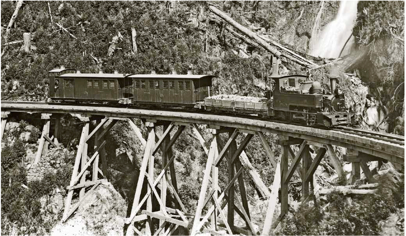
Part of a much larger John W Beattie glass lantern slide (one of two near-identical pictures taken a few minutes apart – cf. Tasmanian Mail , 10 Aug 1901), showing a Sharp Stewart 0-4-2T G-class on a short mixed train heading to Zeehan and the smelters, circa 1900. The original (damaged) print includes the full height of Montezuma Falls – all 340 ft. The 10-span Montezuma bridge was on a two-chain curve and a 1:43 grade. The train consist comprises open wagon AA3 containing bulk ore, AB2 – a 1st/2nd passenger car, and AD1 – a combined 1st-class/guards van. Photo: State Library of Victoria H92.350/164
