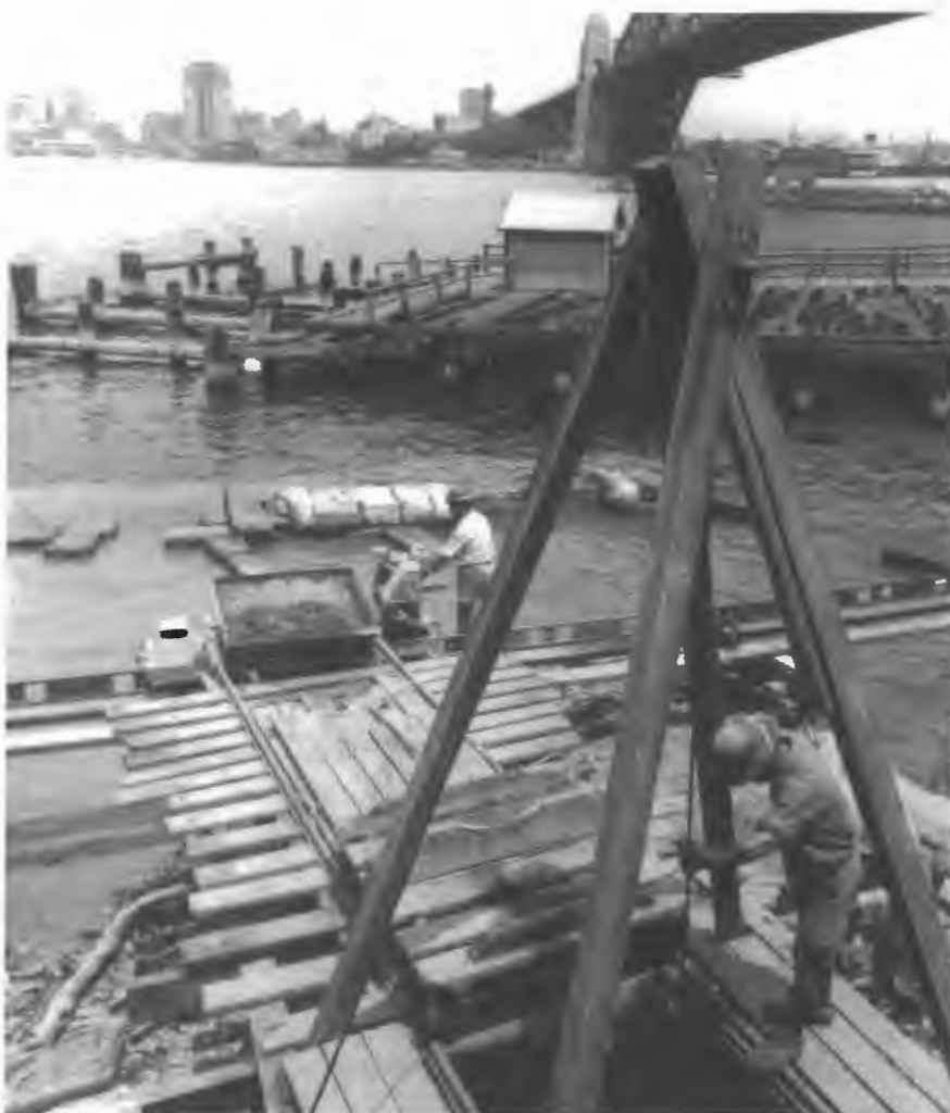
Monorail system at Jeffrey Street wharf, 1965, helping build a new sewer tunnel. The kibbles of spoil are being shunted on a short length of track, then emptied into the monorail transporter. Photo: Sydney Water Board
