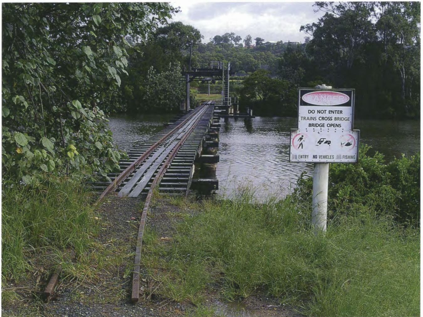
The Maroochy River bridge remains intact, 3 May 2005.
