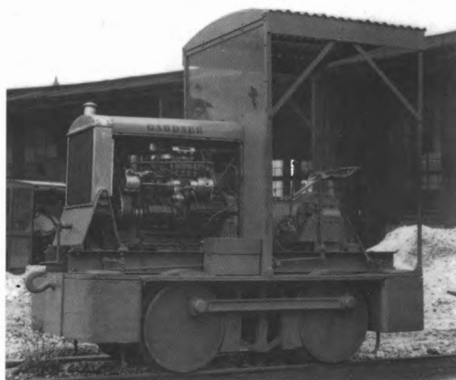
The photograph provided to Andrew Forbes of the 0-4-0DM at the Hobart roundhouse. It is believed to have been taken by CM Plane after fitting of the Gardner 4LK engine in 1950.
