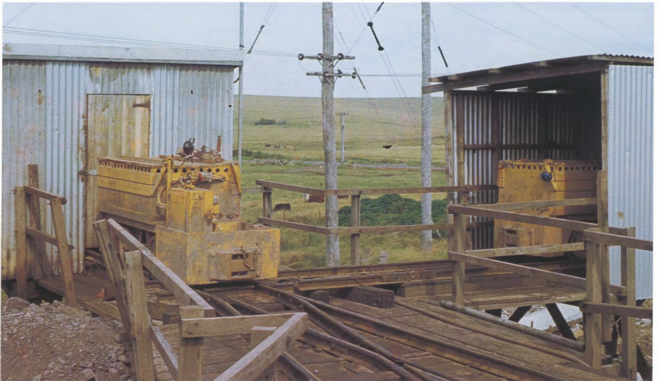
Anti-clockwise, from above: Haulers 78, on the loading dock, and 85, in the charge house, at the Oak Flats Sub-Main Construction, Shell Harbour. Note the small turntable to allow the locomotives to be manoeuvred. 17 April 1976. Photo: John Browning □ Hauler 79 after conversion to 760mm gauge, with battery box 95, in the battery charging room at the Springwood tunnel portal. The batteries to either side are for the shuttle cars, December 1990. Photo: MWSE&DB. □ 4wBE Trammer 98 at the Oak Flats Sub-Main Construction, Shell Harbour, 10 May 1977. Photo: John Browning □ 0-4-0BE Trammers 57 & 61 in store at the Plant Maintenance Depot, Birrong, 10 May 1977. Photo: John Browning
