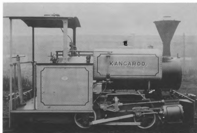
The photograph provided to Andrew Forbes of the 0-4-0DM at the Hobart roundhouse. It is believed to have been taken by CM Plane after fitting of the Gardner 4LK engine in 1950.
