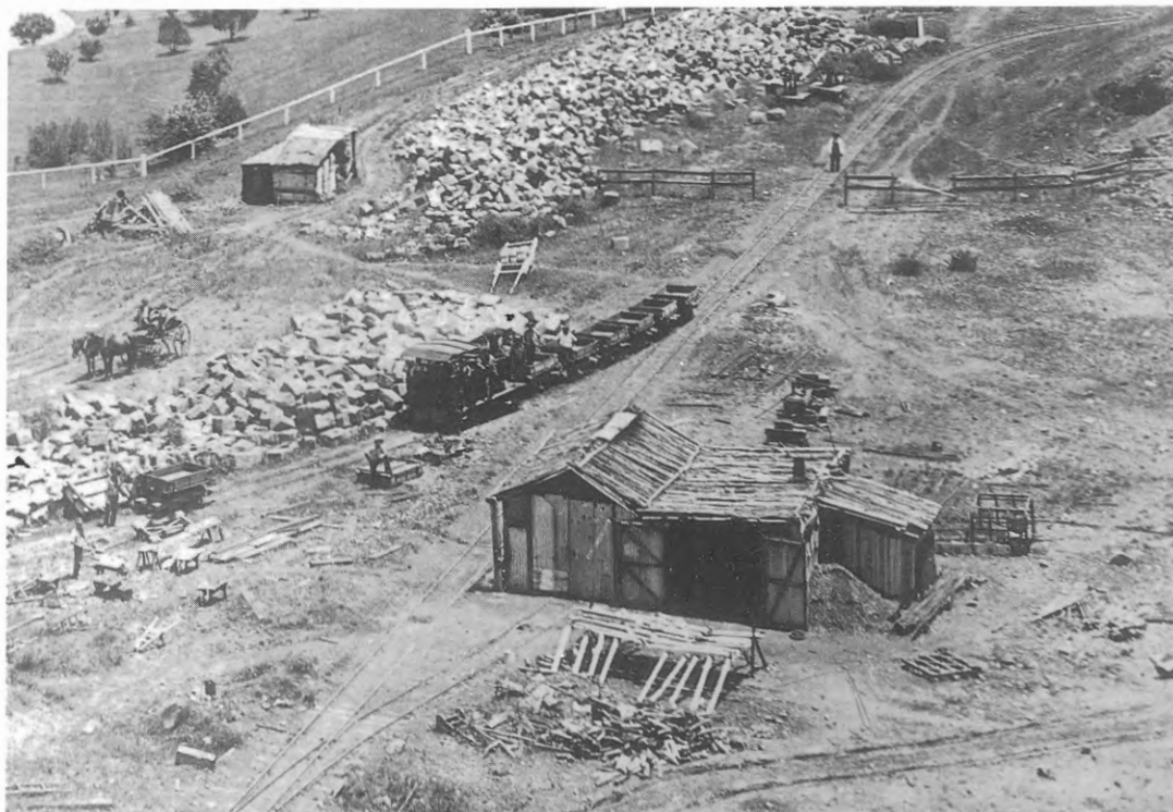
Prospect Reservoir 2 ft 6 in gauge system during stabilisation works on dam wall.
