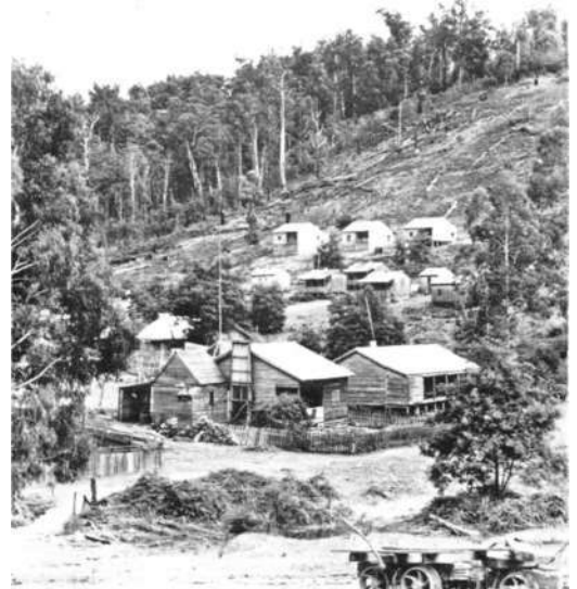
Mill houses at Morgan's on the Western Tyers River. The houses in the background belong to Ingram, those in the foreground to Morgan.
