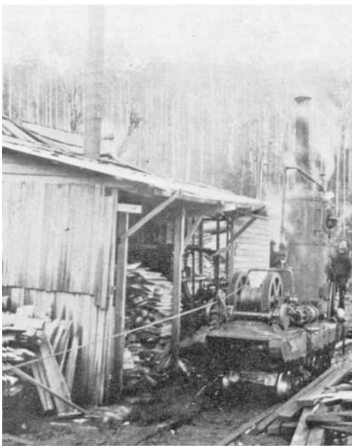
Christensen and Saxton's tram construction winch, c1930. W. Saxton
