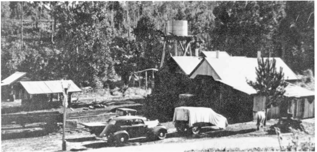
The FCV locomotive depot at Tyers Junction in 1927. Note the ballast truck constructed from two timber bogies. J. Westcott
