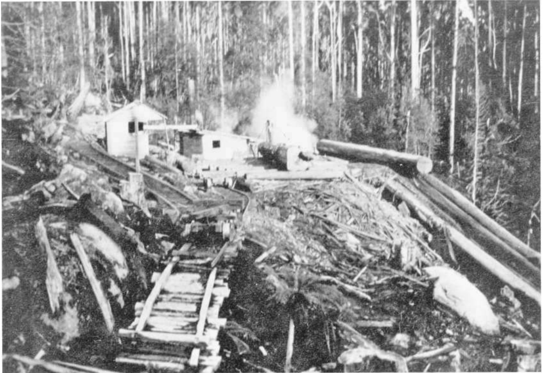
Log winch at the top of the first stage of Christensen and Saxton's second incline, c. 1930. W. Saxton
