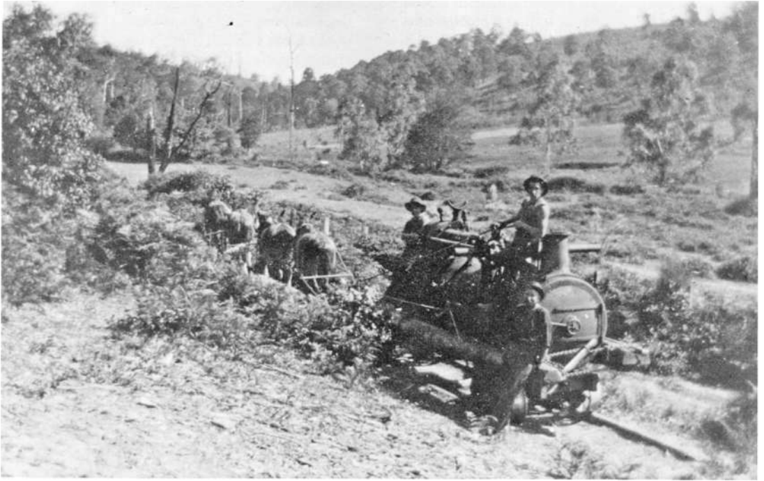
Shifting one of the two boilers at Henry Collins' mill to the new site on the Middle Tyers River in 1923. M. Collins
