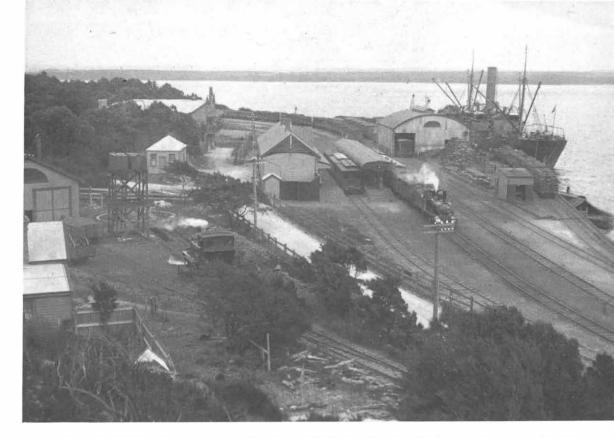
Above Regatta Point station. A Tasmanian Government Railways train from Zeehan can be seen in the right hand platform, with a 2-6-0 tender locomotive. On the left is a Mount Lyell Mining & Railway Company 0-4-2 Abt Rack locomotive, while the Mount Lyell Company's train waits in the left hand platform. On the right copper concentrate from Queenstown is being loaded on board the ship.
