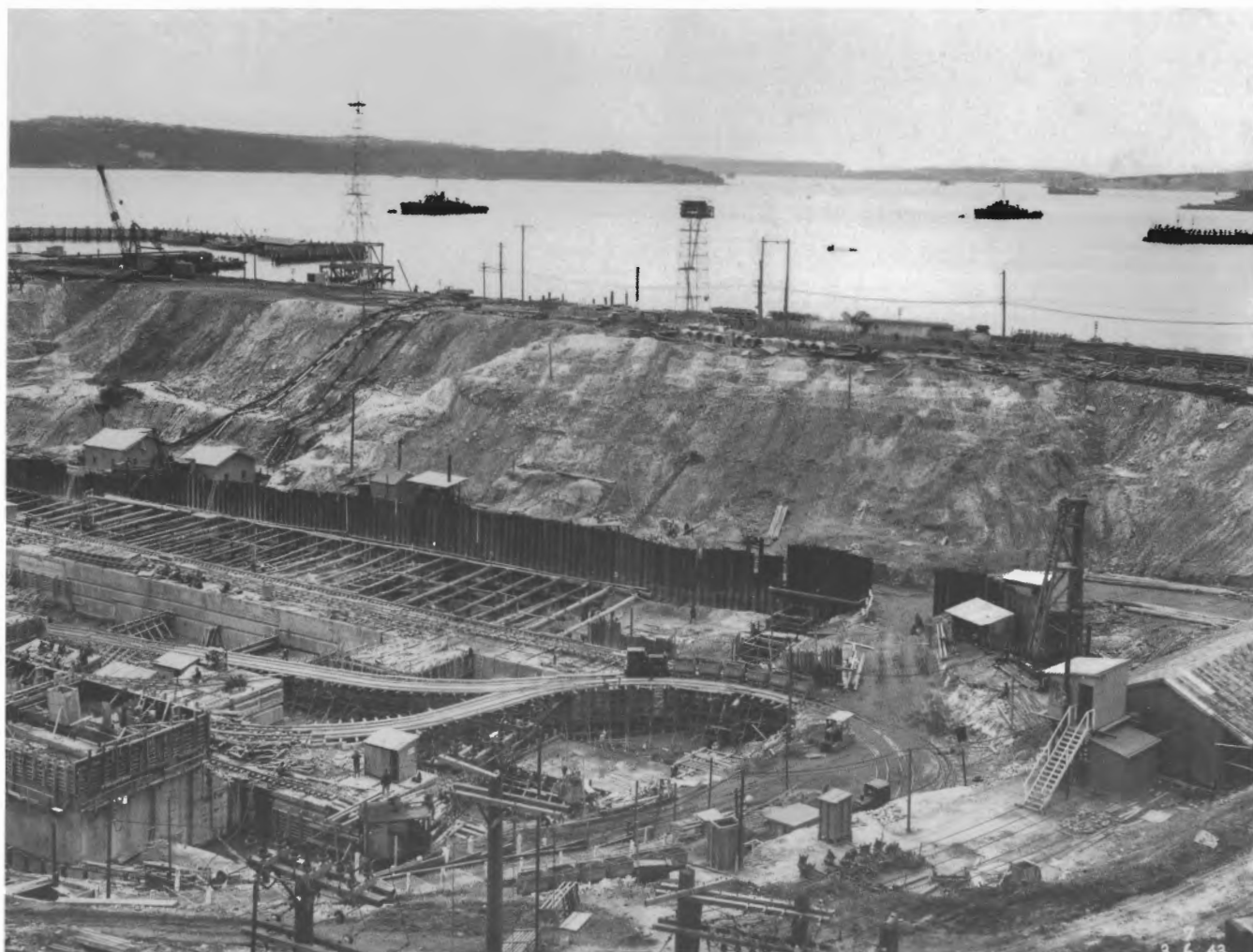
A rake of loaded concrete skips descends the incline while a Days locomotive waits at the bottom, near HILDA, which is off the track nearby. BETTY propels a rake of empties towards the incline foot. Track is nearly completed along the eastern line of floor blocks, which will allow the removal of the lines along the centre line of the dock, 3 June 1943.
