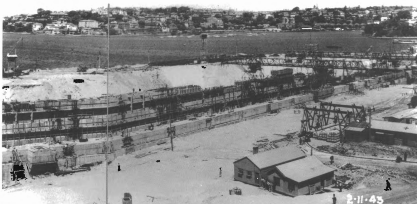
Backfilling behind the western walls of the dock has been completed and the pile storage yard can be seen on the right with piles stacked beneath the lifting gantry, 2 November 1943. The line running from the storage yard connects it with the pile casting yard.
