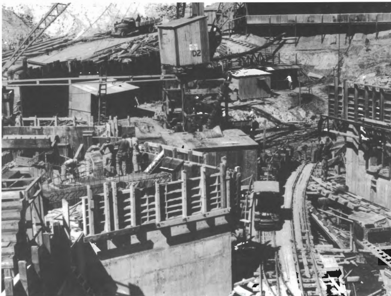
Construction of the walls at the south end of the dock is well advanced but a gap has been left for the tramline to pass through with HILDA and train occupying one of the pair of tracks, 2 September 1943. Photo: State Records NSW: CGS 12490, 6/4497, 342
