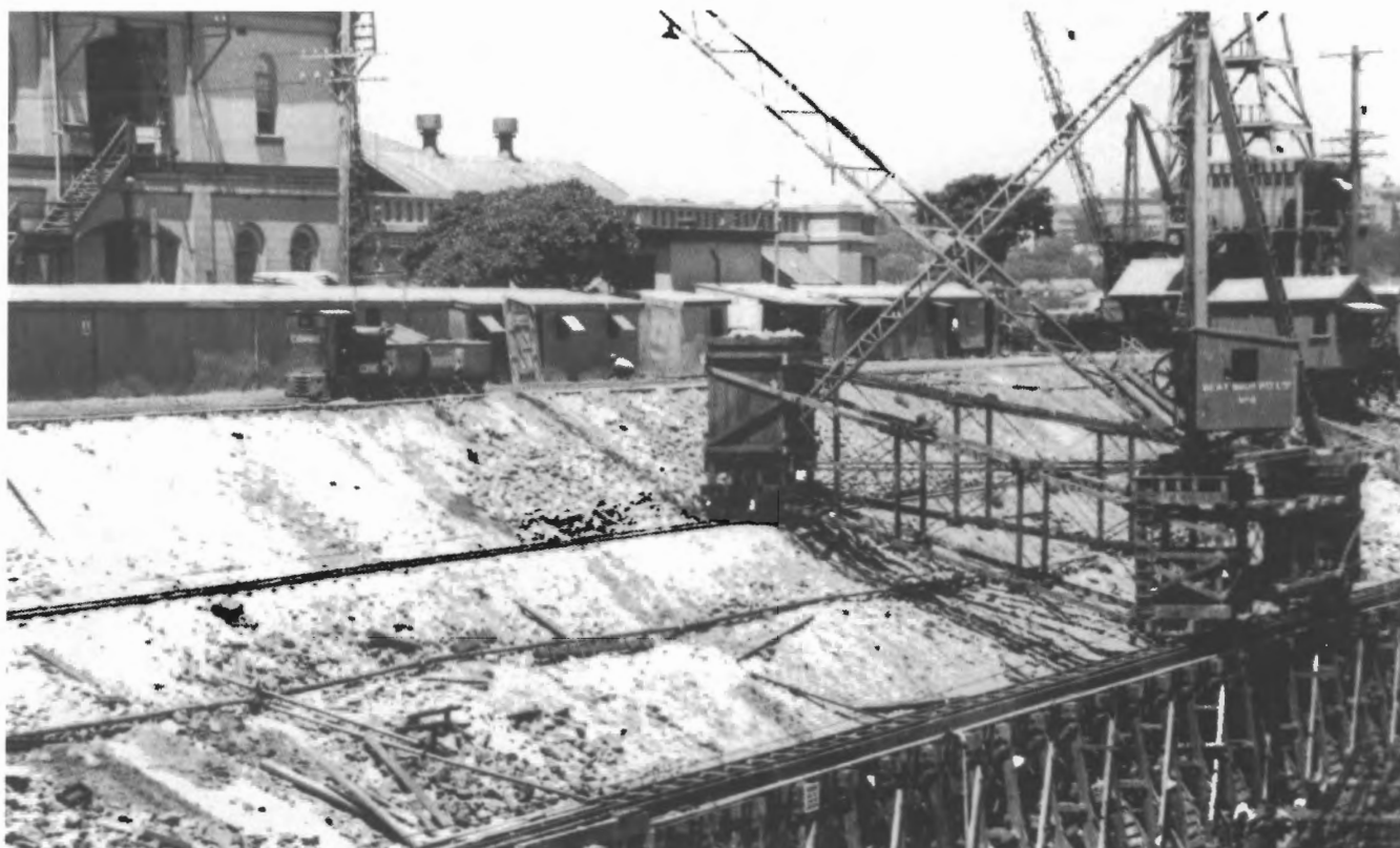
Construction of the East Wharf of the Graving Dock, 3 February 1943. Ruston & Hornsby locomotive CONNIE at the top of the coffer dam wall with the derrick crane assembly running on narrow gauge tracks on the two parallel tracks below. Photo: Jim Longworth collection
