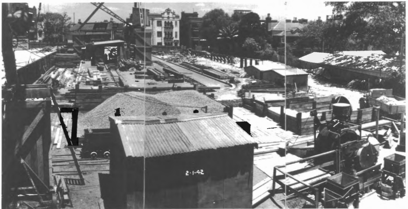
The sawmill and concrete mixing plant off Collins Avenue, Potts Point, with associated 2ft gauge railways in the early stages of construction of the Graving Dock, 2 January 1942. Photo: State Records NSW: CGS 12490, 6/4495, 68
