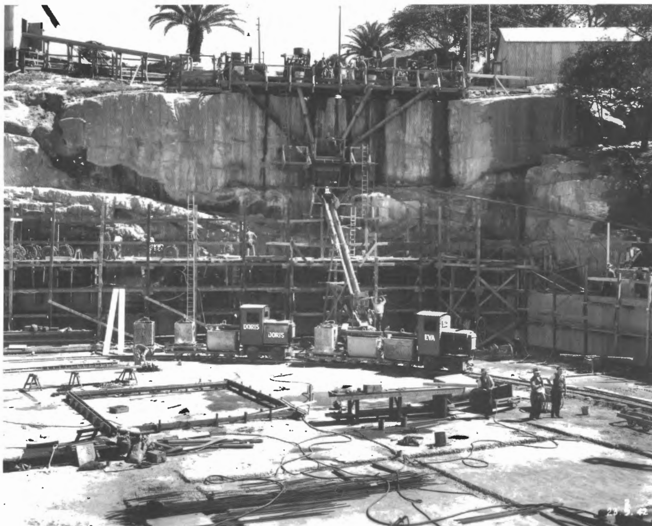
The Domain Oil Tanks Construction. Days locomotives DORIS and EVA, with skips at the bottom of the concrete delivery chute, 23 September 1942. Photo: Jim Longworth collection
