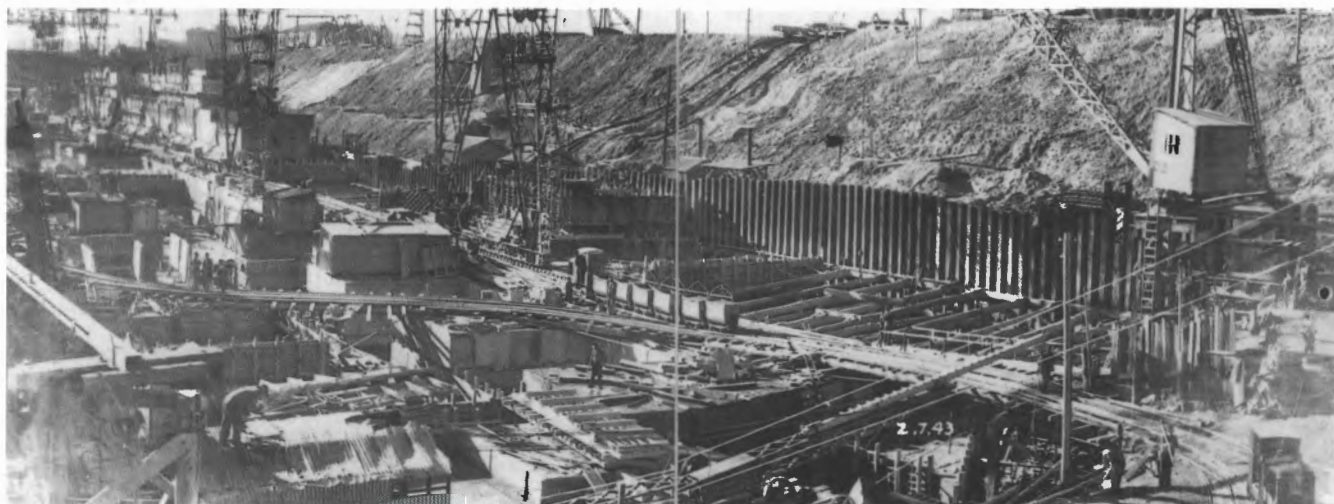
Afternoon shadows creep across the dock on 2 July 1943. A Ruston & Hornsby is on the right with a Days type on the eastern side line in the centre and another in the far distance. HILDA is lurking behind the shed left of centre. The telfer cranes are now fully operational while the centre of the dock floor is rapidly becoming covered by a mass of buildings and equipment. Photo: Bruce Macdonald collection
