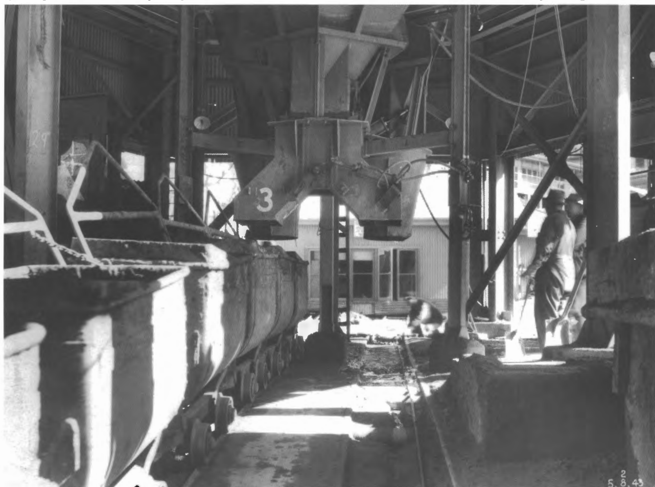
Loading Hudson concrete skips at the central mixing plant, 5 August 1943, with the winding house visible behind. Photo: Jim Longworth collection
