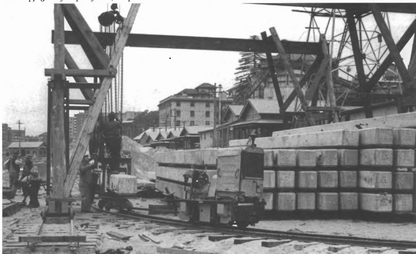
The small locomotive handling a set of pile bogies at the pile storage yard, 3 November 1943. Note the long connecting bar. The overhead lifting gantry runs on 2ft gauge track. Photo: Jim Longworth collection
