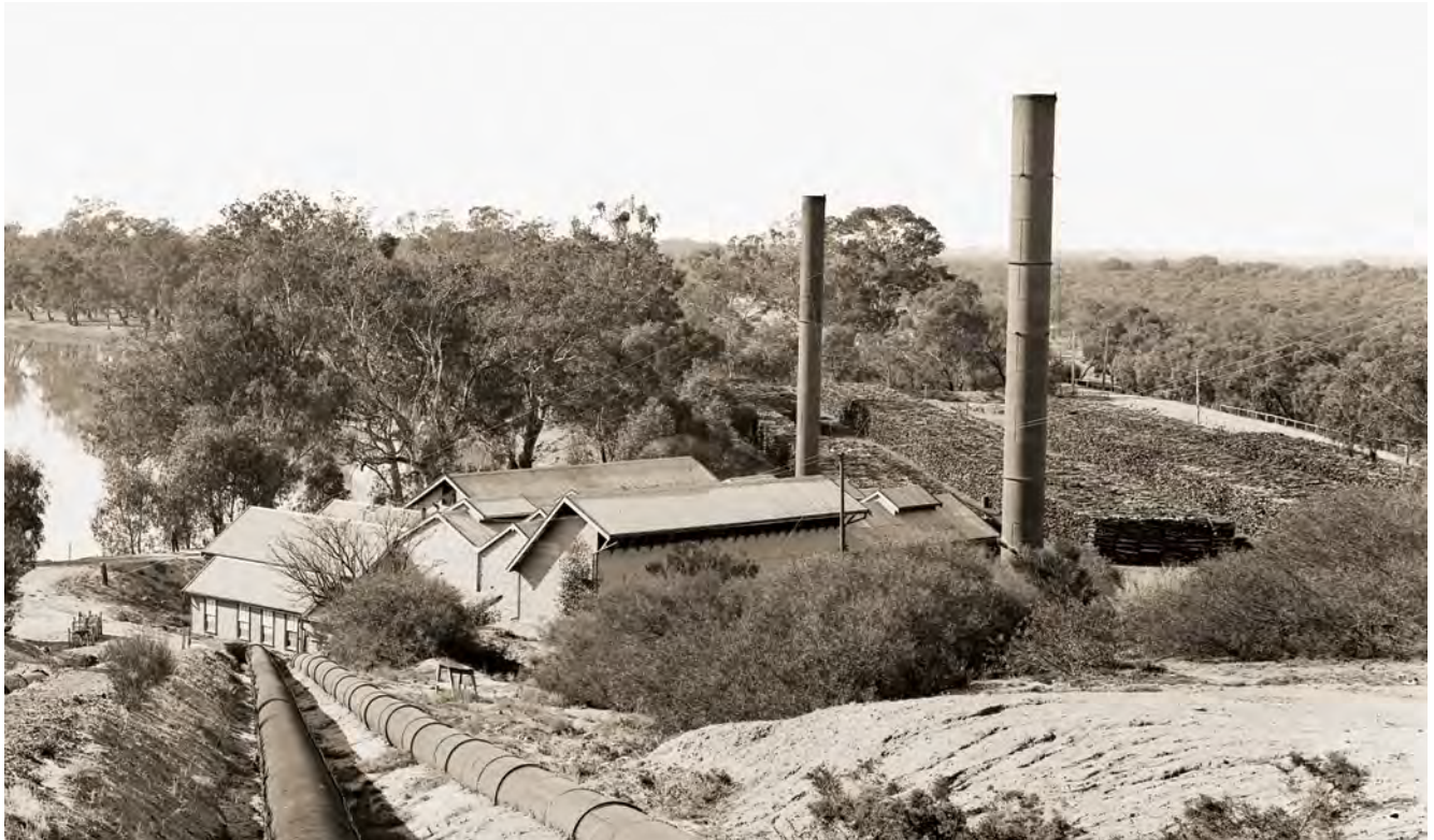
Merbein pumping station c1930. Constructed in 1909, it supplied the Merbein irrigation area to the west of Mildura. By 1935 it was consuming 20,000 tons of firewood a year which was deemed to be not sustainable. A decision was made to convert it to electrically powered pumps with the electricity to come from alternators at Red Cliffs pumping station. The change was to have a profound impact on the volumes of coal and/or briquettes carried by the Red Cliffs pumping station light railway.
