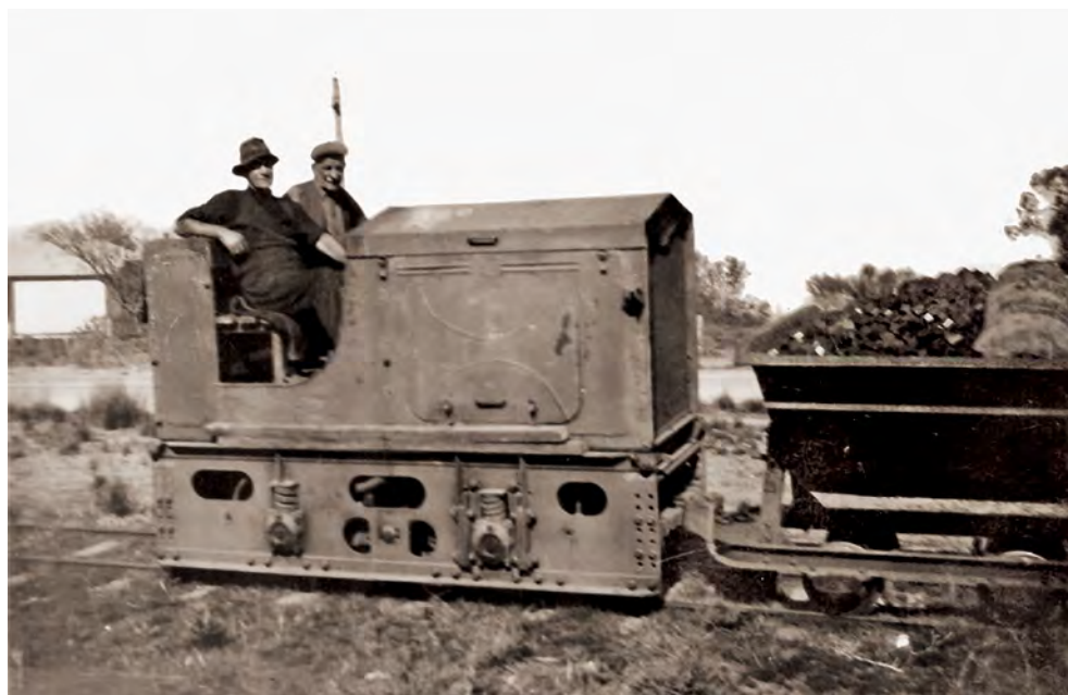
SR&WSC 18-C-12, a Malcolm Moore V8 powered petrol engine locomotive about to pass onto Fitzroy Ave in Red Cliffs c1953. This was the last of the 1000 series Malcolm Moore locomotives to arrive at Red Cliffs, and had previously been in use at the Rocklands Dam project in Western Victoria. It was later put to work by the SECV on the ash tramway at the pumping station and in 1977 it was donated to the Puffing Billy Museum at Menzies Creek where it was restored to operating condition. It remains there to this day. Photo: R Earle, Red Cliffs and District Historical Society
