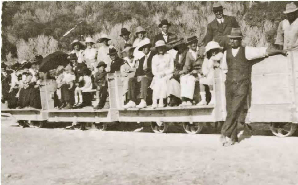
A study of available photos of the 2ft-gauge passenger trucks shows that prior to the 1913-14 season the unsprung flat trucks merely had a footboard and uncomfortable wooden longitudinal knife-back seating. For the 1913-14 season solid timber ends were added, presumably for passenger safety. Unfortunately, no extra trucks were added to the fleet, leading to extreme crowding at times, with the overflow passengers jammed, standing or sitting dangerously on the sides of the luggage trucks. Photo: 'The Rottnest Tram' – Murray Views post card, Hugh Ballment colln.
