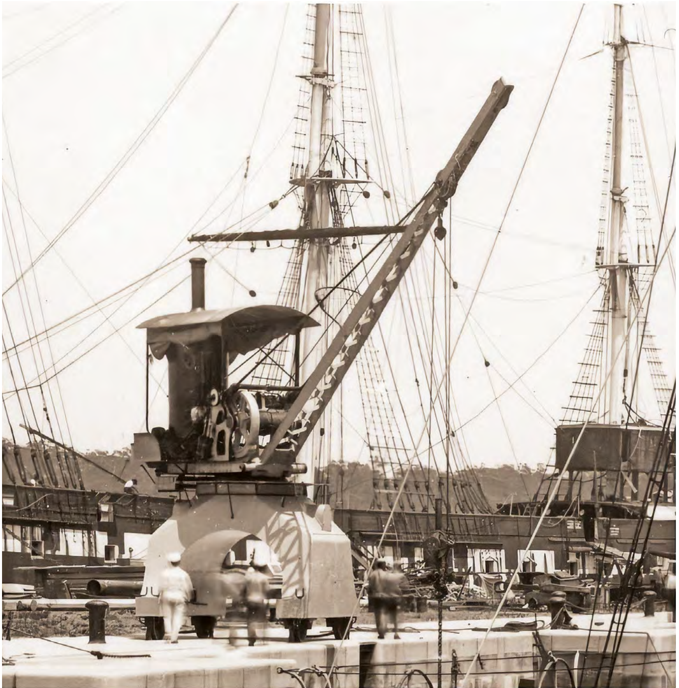
Travelling steam crane No.002 in its original condition when delivered from England with a totally open cab. It is seen here alongside HMS Karakatta and HMS Wallaroo, Sutherland Dock, Cockatoo Island, 1900. This crane and its identical twin saw active service into the 1980s.
