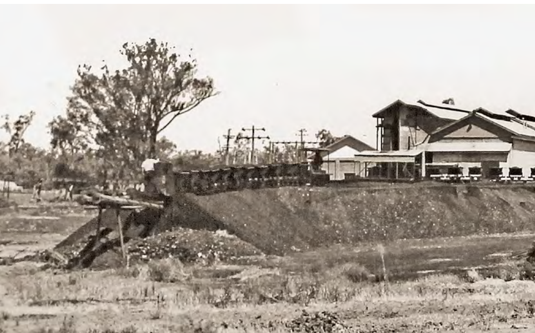
From 1946 to 1952 severe fuel rationing in Victoria saw the Red Cliffs pumping station denied access to briquettes for fuel. This meant a return to using the much-maligned Wonthaggi screened coal as fuel for the furnaces. This image, recorded c1947, shows the small Malcolm Moore locomotive at work on the coal heap. The track is laid directly on the coal and was movable to meet needs. A somewhat rustic temporary trestle is in use to allow the skips to offload beyond the end of the heap. A man is engaged in tipping a skip. Photo: State Library of Victoria, Rural Water Collection
