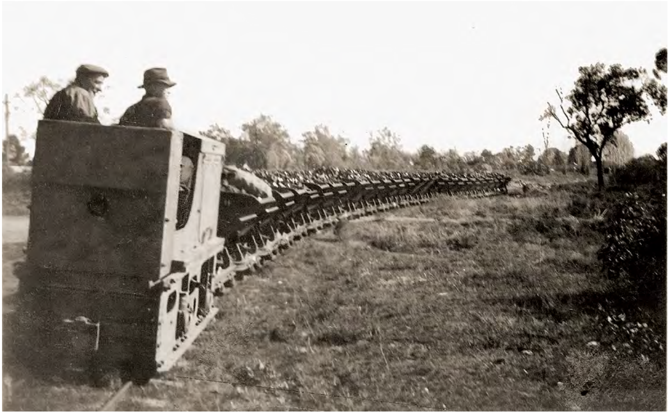
A rake of 22 trucks laden with briquettes on the curve approaching Fitzroy Avenue, Red Cliffs during the months leading up to closure in 1954. The locomotive is SR&WSC 18-C-12, fitted with a Ford V8 engine. Photo: R Earle, Red Cliffs and District Historical Society
