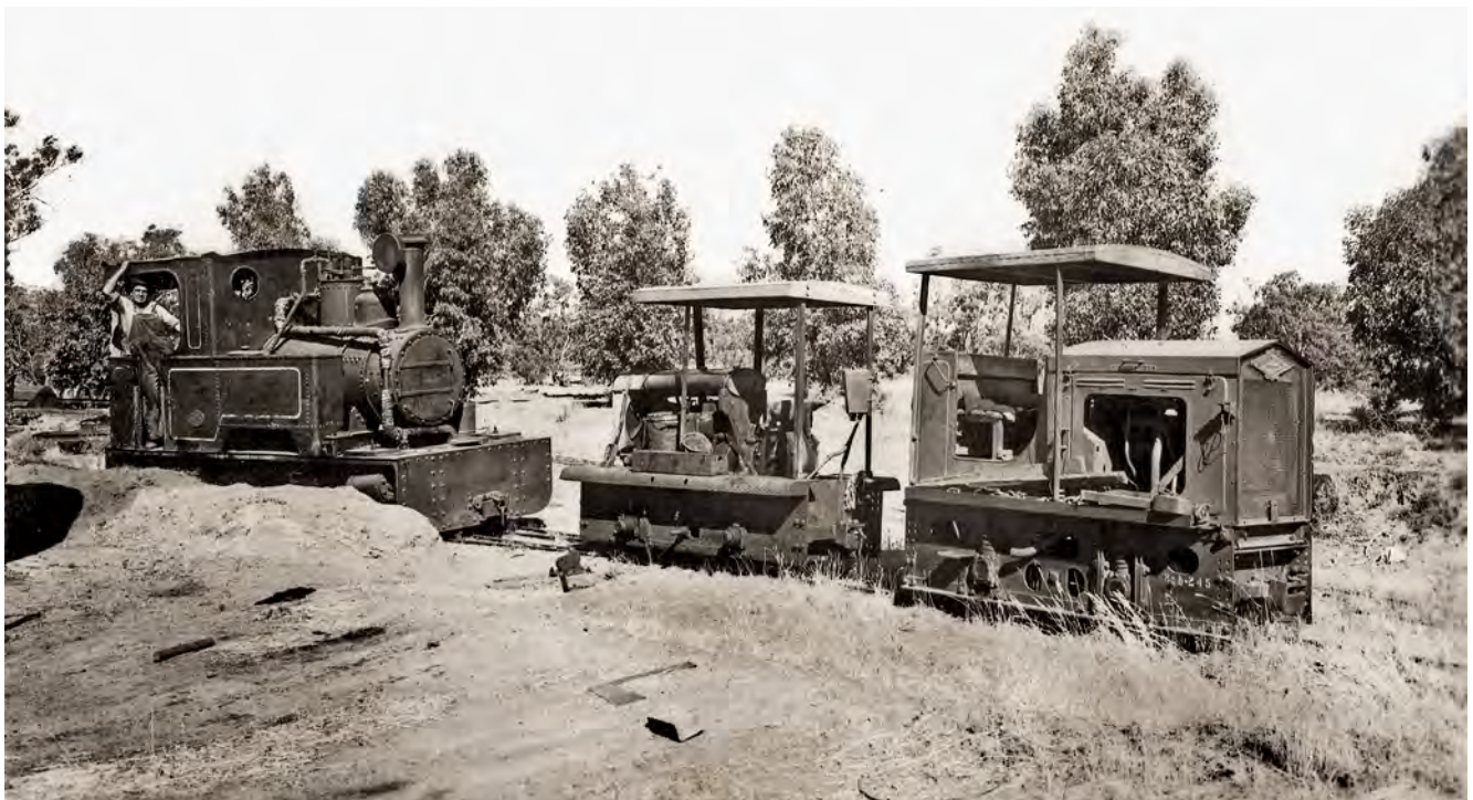
Malcolm Moore 8-B-245 has pulled the small Fordson Major powered loco and the Kerr Stuart out into the sunlight for the benefit of an Arnold Lockyer photograph in March 1951. Wooden skip sprags and a rerailing jack sit on the larger Malcolm Moore while the smaller unit has been given the benefit of what appears to be a sandbox at its rear. The Kerr Stuart displays its heavier tank-side lining applied after the 1940/41 rebuild. Photo: Arnold Lockyer
