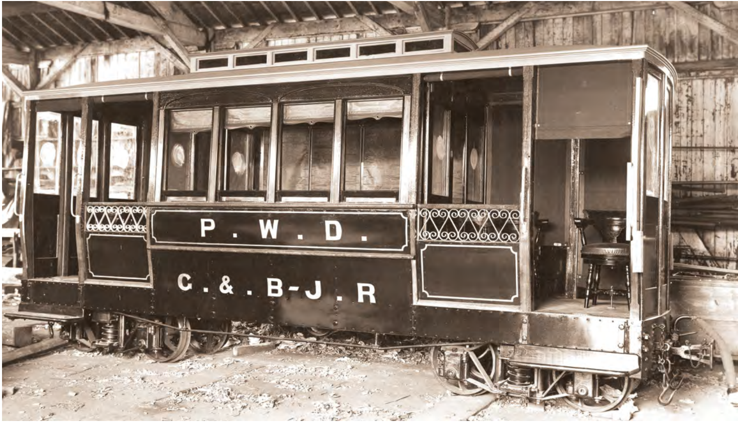
The State Car built on Cockatoo Island for the Goondah-Burrinjuck Railway. This beautiful little vehicle must be one of the most ornate narrow-gauge carriages ever to operate anywhere in Australia. Lavishly appointed to transport dignitaries and senior management it was also fitted with a full air brake system.
