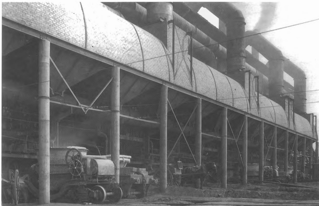
The huge scale of the Cobar furnaces and the various modes of transport for industrial waste products are evident in this classic scene of the 'slag road' on the eastern side of the furnaces. Two electrified rail sidings serve each of the five 'settlers'. Slag pots are being charged from the 'settlers', while an electric 'motor' waits on the far right to haul a pot to the slag dump roads. Reclaimed dust was collected from the chutes above the rail sidings, and the horse and cart is presumably engaged in transporting this product back to the furnace bins. Photo: Cobar Regional Museum
