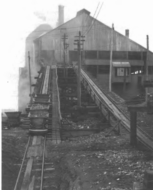
Ore for the blast furnaces in narrow gauge side-tipping skips being hauled by electric winches up to the furnace "feeding floor".
