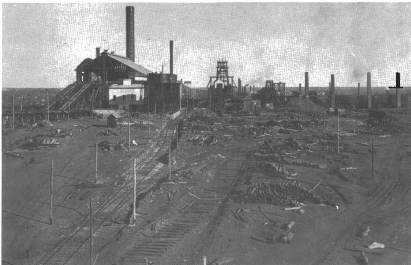
The Great Cobar Mine and Smelters, as they appeared in 1908. Some idea of the magnitude of the operation can be gained from this view of the works under construction. In the foreground an old siding is being removed and the electric line constructed. Photo: Great Cobar Ltd
