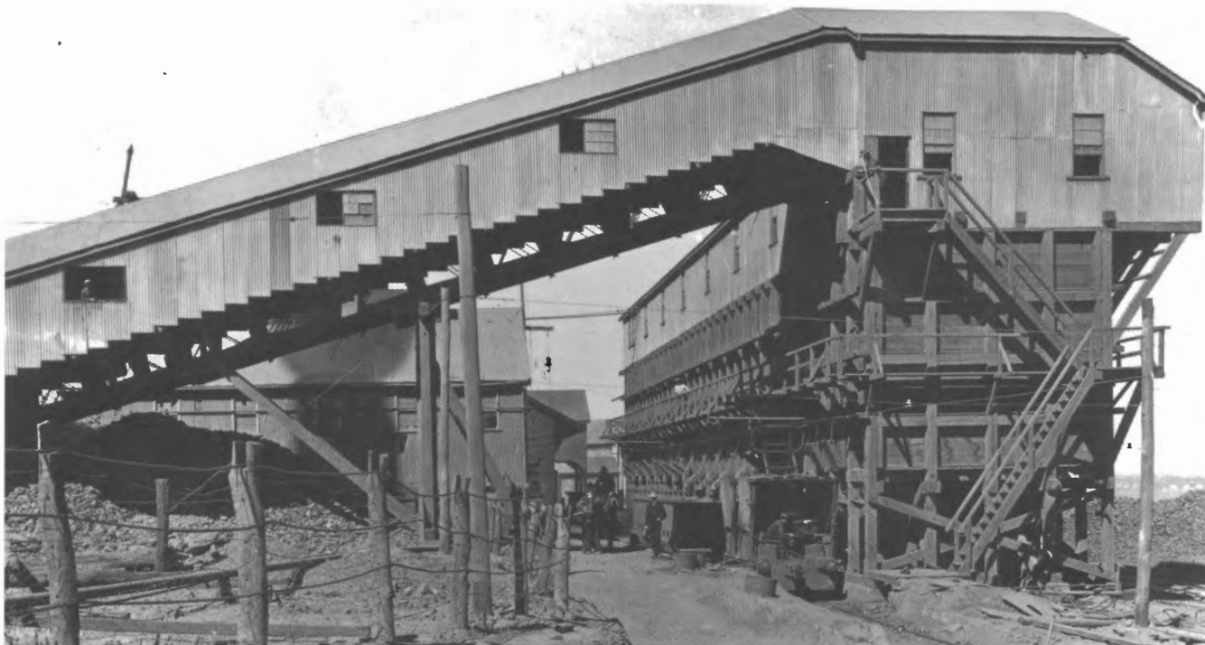
This mood scene depicts an electric 'motor' on the track beside the 6000-ton "Bedding Bin", while a horse providing more traditional transport surveys the scene. The steel-plate conveyor from the crushers to the bin dominates the scene. Note discarded refuse on the left and the "picky boy" in the process of adding to the pile from the window on the left.
