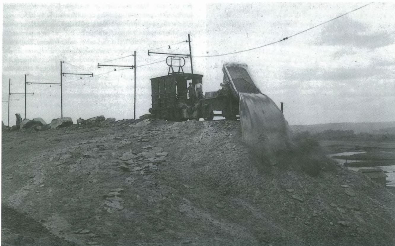
One of the Pollock end-dump pots being emptied at the Great Cobar slag dump. The car has been chocked to the rail and the motor has moved away to pull the tipping chain. At night, the glare could sometimes be seen from over 25 miles away. Photo: Cobar Regional Museum
