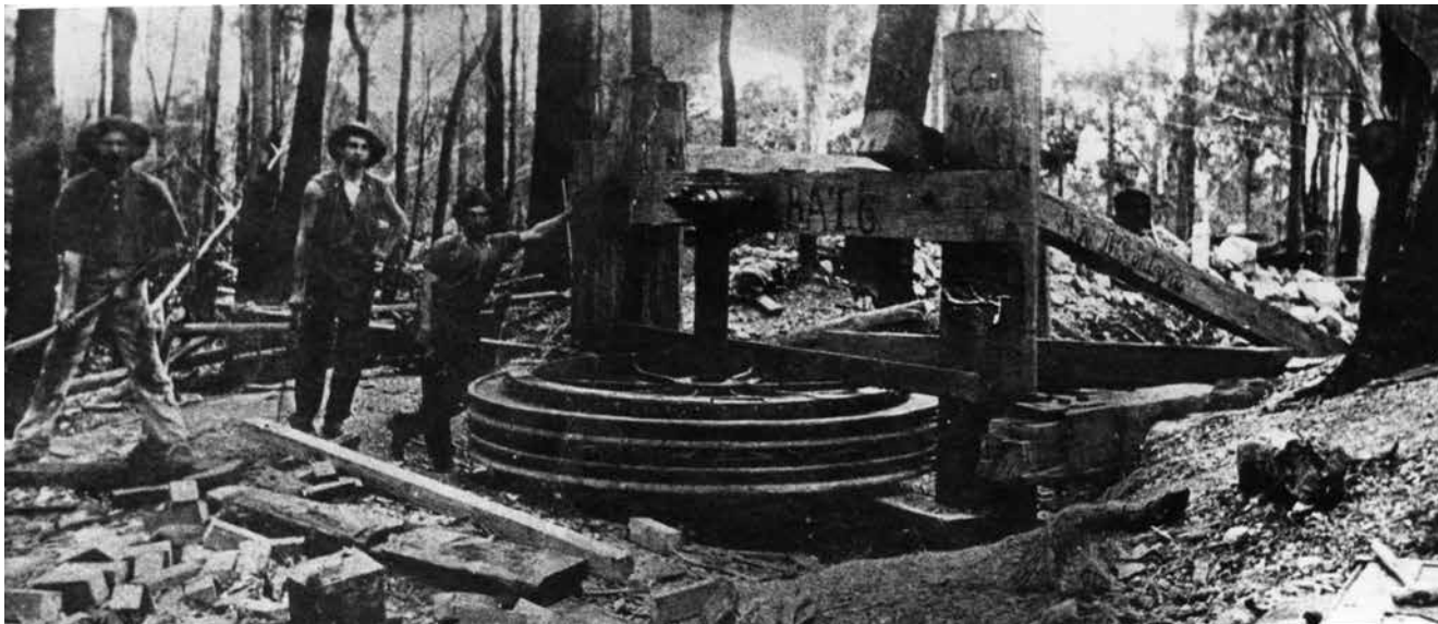
Workmen installing the horizontal bull wheel at the top of the tramway incline in 1908. The ½ mile 1 in 5 incline was gravity operated, with descending loaded timber trucks hauling empty trucks up hill. The earth platform that supported the bull wheel was still visible in 2014.
