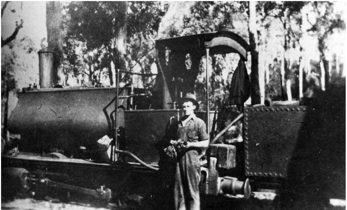
Following the closure of the BATCo's Woolgoolga operations in 1914, the Murray and Paterson locomotive was acquired by Hepburn Mackenzie for his timber venture on Fraser Island. Arriving there in 1918, the locomotive acquired a homemade tender to carry additional water and fuel.
