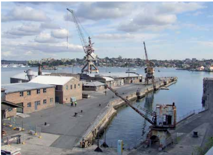
Massive rail based cranes were capable of being moved around the Sutherland (pictured) and Fitzroy graving docks via a network of tracks.
