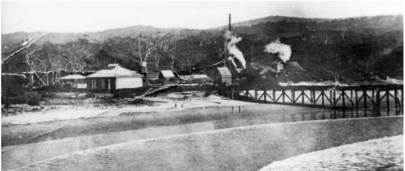
The BATCo's Jetty Sawmill was situated beside Woolgoolga's ocean jetty. A short siding connected the mill to the 3ft 6in gauge tramway which ran the length of the jetty to a steam crane at its outer end. The mill's sawn and hewn timber products were loaded onto 4-wheel flat trucks and horse-hauled out to the crane to be loaded onto coastal steamers. Photo: Neal Yates collection
