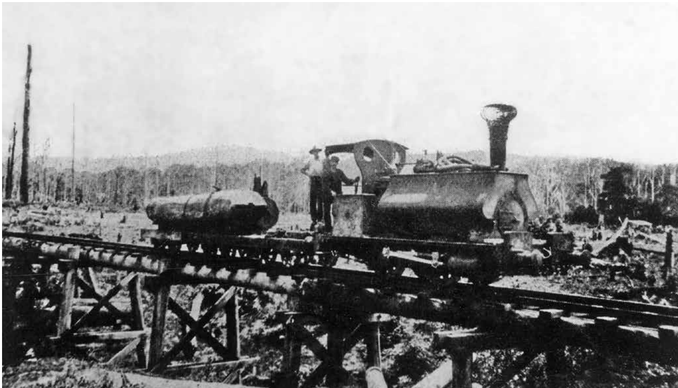
The only known photograph of the BATCo's Murray and Paterson 0-4-0ST locomotive (205 of 1886) on the company's 3ft 6in gauge Woolgoolga timber tramway. The basic timber trestle bridge is probably one of the bridges constructed to criss-cross the line over Woolgoolga Creek on the way up to the base of the gravity incline.
