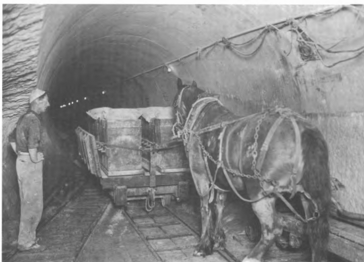
Aggregate Truck being pushed to the working face during installation of mild steel lining at Pressure Tunnel. Note bags of cement on top of batch boxes. Photo: Sydney Water Board.
