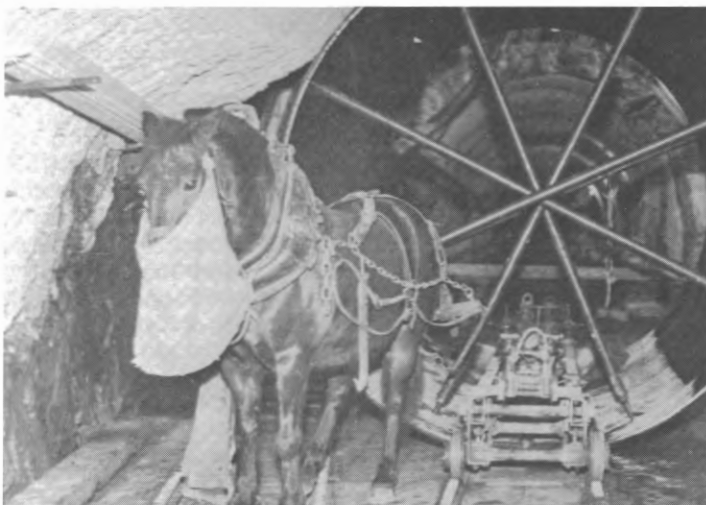
8 ft. 3 in. steel linings being placed inside ruptured original concrete lining as a remedial measure. Photo: Sydney Water Board.
