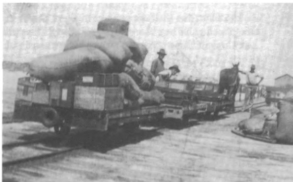
Horse operated tram at jetty head, Mauds Landing, hauling three wagons, c. 1925. Photo: Courtesy Ric French.
