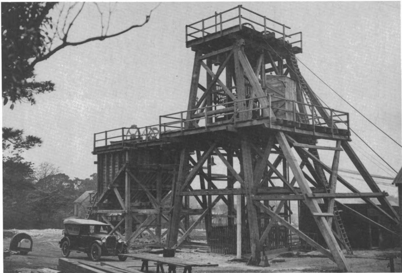
Poppet head and double rotary tippler over spoil bin at Shaft 13 on Sydney Pressure Tunnel excavations.
