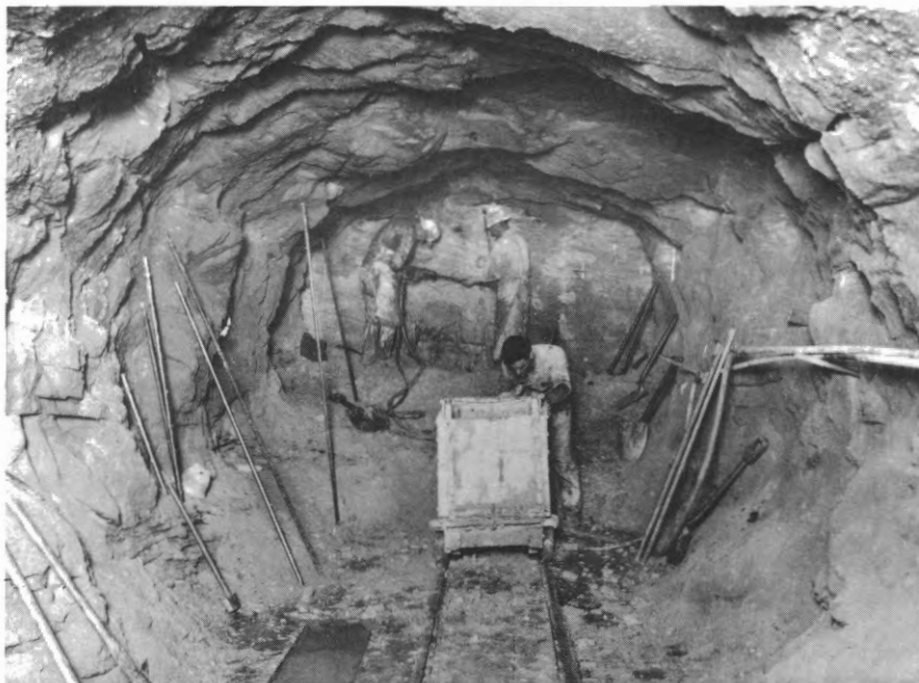
Pressure tunnel excavation by drill and blast methods.
