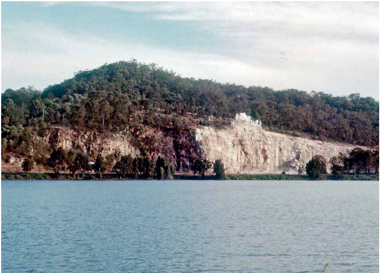
Blasting stone at Ilarwill Quarry, Woodford Island, for Clarence River breakwater construction during the 1960s. The earlier 1900–1903 Woodford Island Quarry workings are shown by the darker rock face on the left. Much of the evidence of these workings disappeared as Ilarwill Quarry expanded. Photo: Norm Brown collection
