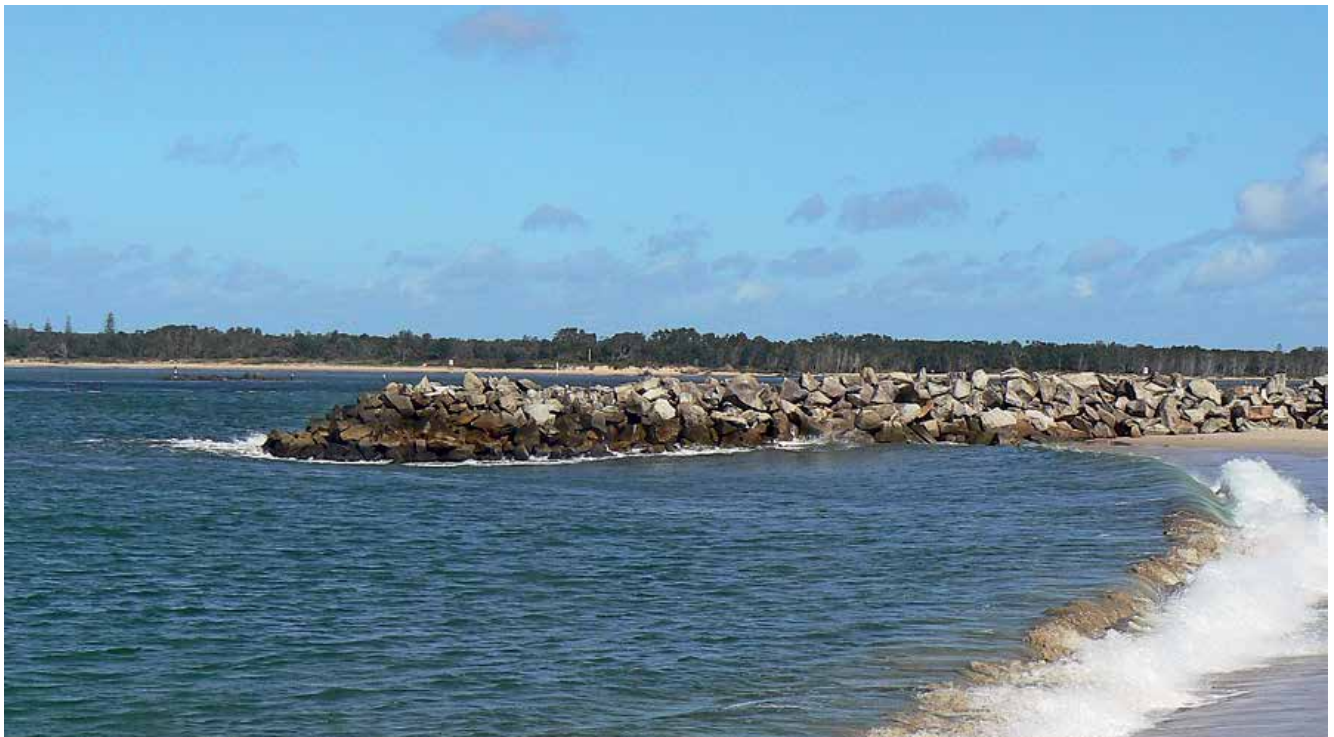
The seaward end of the Iluka Training Wall with the end of the partly-submerged Freeburn Island Training Wall just visible behind it. For over 50 years the Iluka Training Wall was the de-facto North Breakwater, defining the northern limit of the navigation channel into the mouth of the Clarence River.
