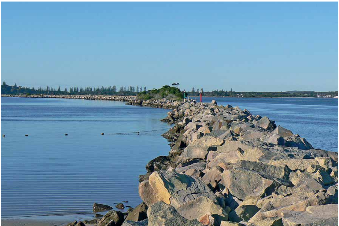
The Iluka Training Wall stretches in a long curve eastwards towards the sea, with the main river channel on the right and the sheltered waters of Iluka Bay on the left. A standard gauge steel-railed horse railway on top of the wall was used to transport stone from the crane wharf, located behind the green channel marker, to the seawards-advancing tip face.
