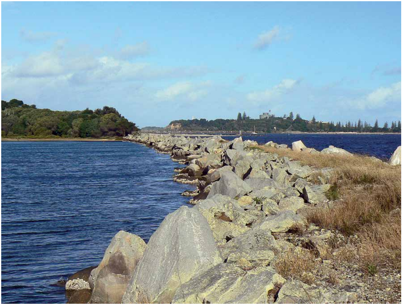
The Iluka Training Wall on the approach to what was then the North Sand Spit. Deeper water and increasing exposure to heavy seas dictated that large blocks of stone up to 10 tons weight were used in its construction and the practice of hand-throwing small pieces overboard off punts was discontinued. South Head and the Yamba foreshore are visible in the background.
