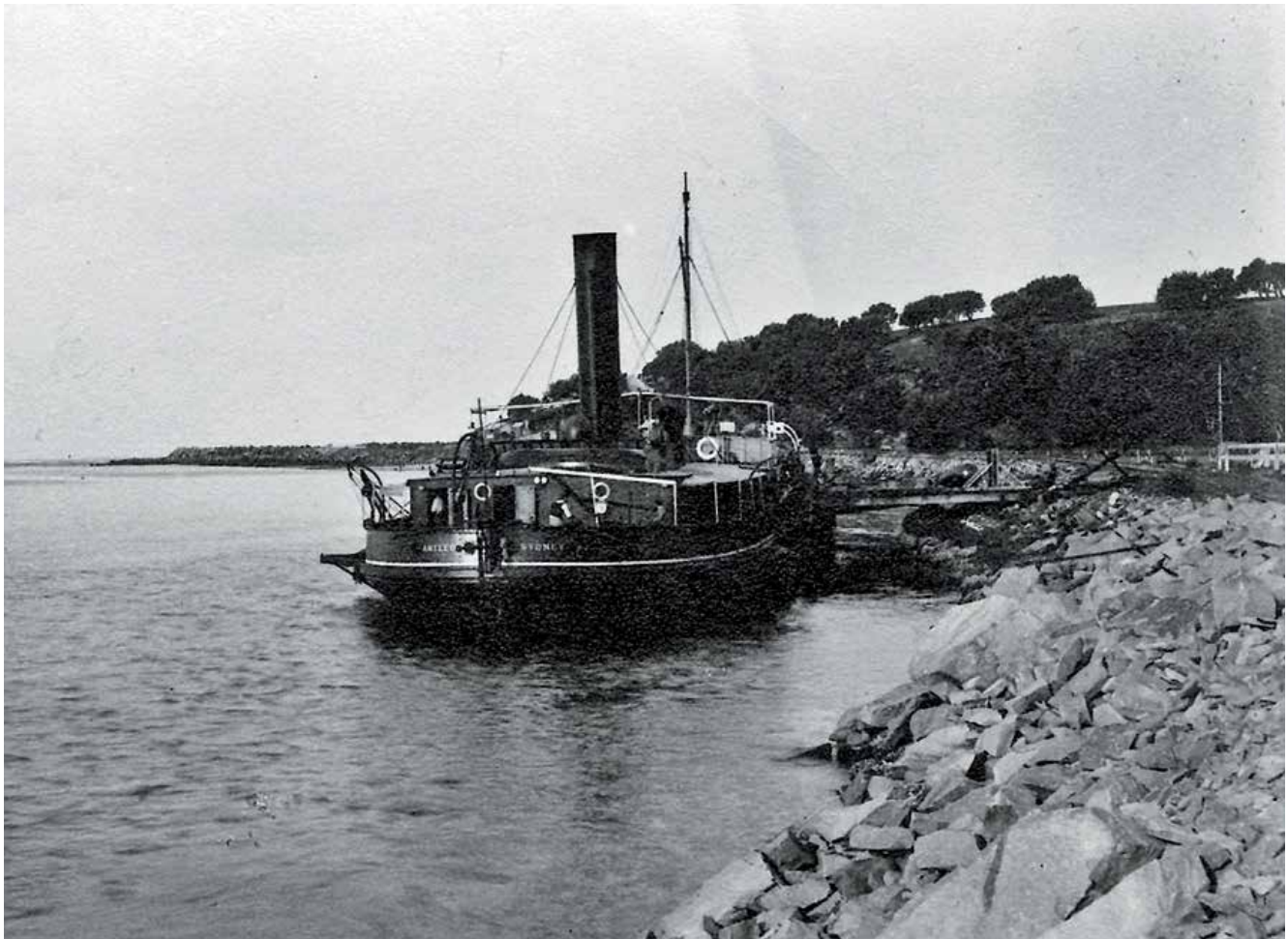
The bar-dredge 'Antleon' moored alongside the Yamba Training Wall. The PWD relied upon its large fleet of dredges as a more economical option to keep the mouths of NSW's navigable rivers open, instead of building and maintaining expensive breakwaters.
