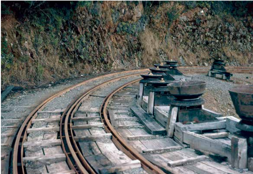
Bottom of the Williamsford Incline showing the track arrangements and cable rollers to allow trucks to go around the corner. Photo: Geoff Thorpe
