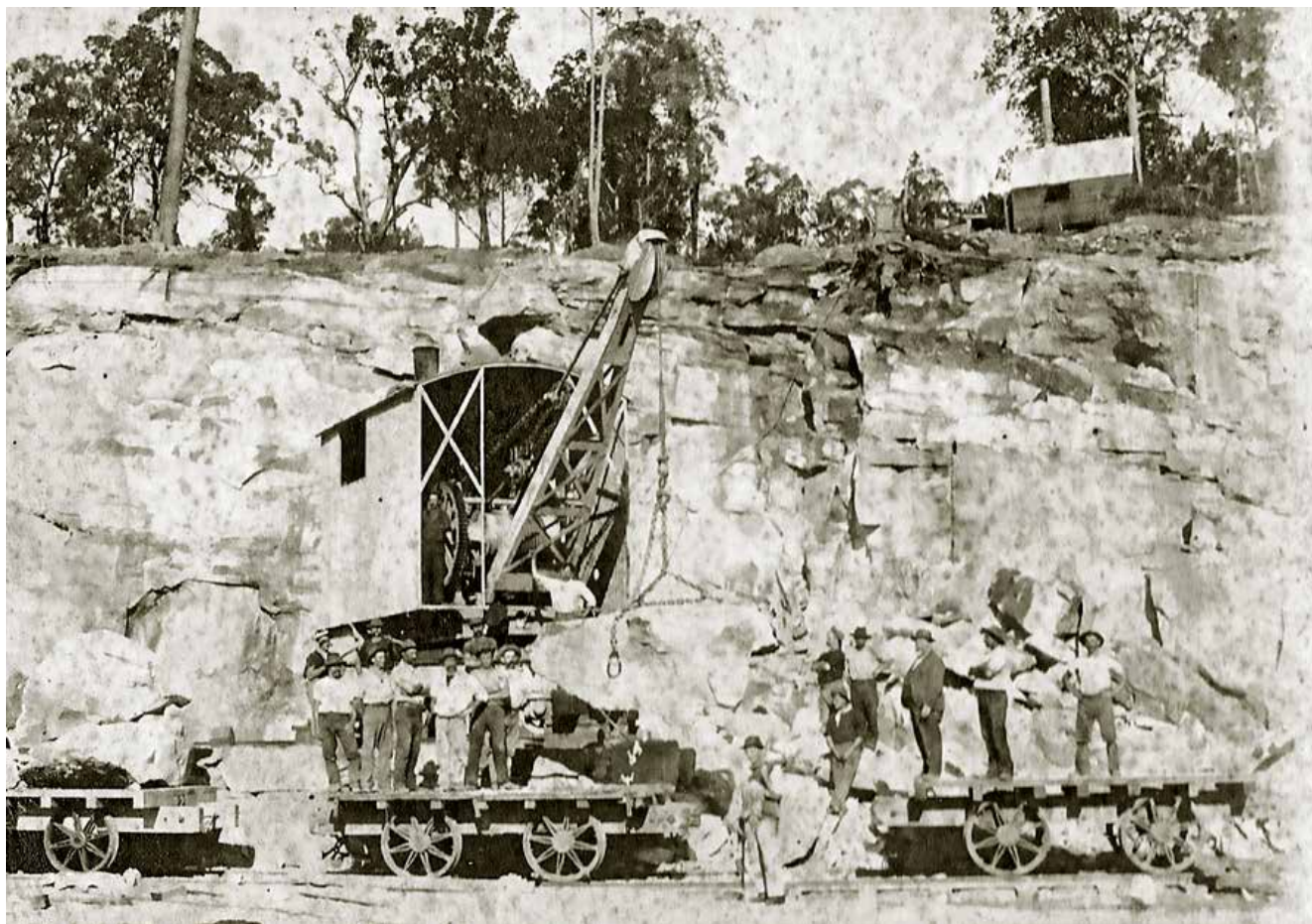
One of the four Woodford Island Quarry steam cranes loading stone onto flat-top rail wagons which will be horse-hauled to the nearby Clarence River stone wharf. The photograph dates to late 1902 or early 1903 when larger stone sizes were needed to construct the seaward section of the Iluka Training Wall. Before that all stone had to be broken up into pieces small enough to be thrown off punts by hand.
