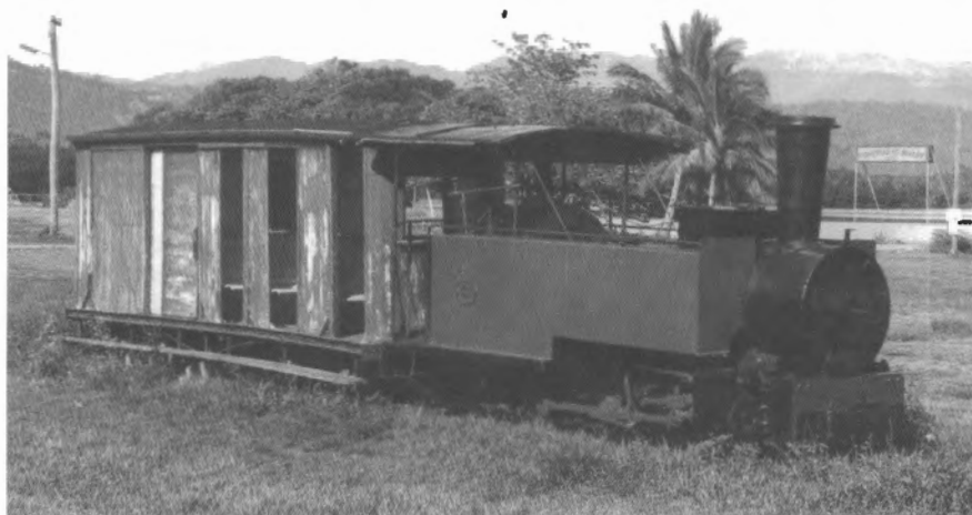
The much-rebuilt passenger car 'preserved' in a sea-front park at Port Douglas, in company with Fowler 0-6-0T FAUGH-A-BALLAGH (8733 of 1901), 17 August 1966.. Photo: GLC Rogers
