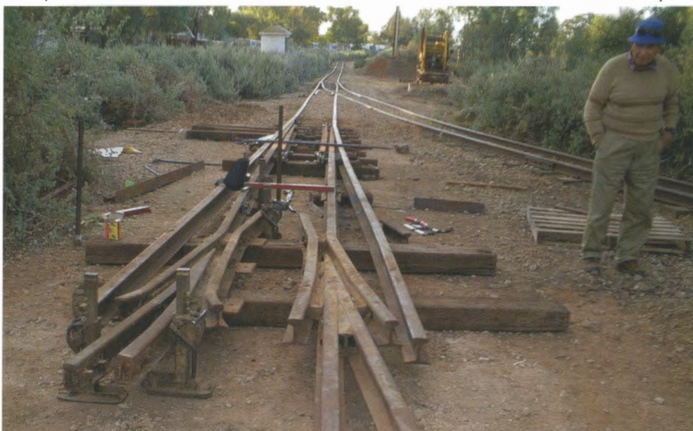
At Cobdogla Irrigation Museum, a start has been made on building a set of triple points to service the two tracks into the new loco shed and the existing storage line.. Photo: Denis Wasley
