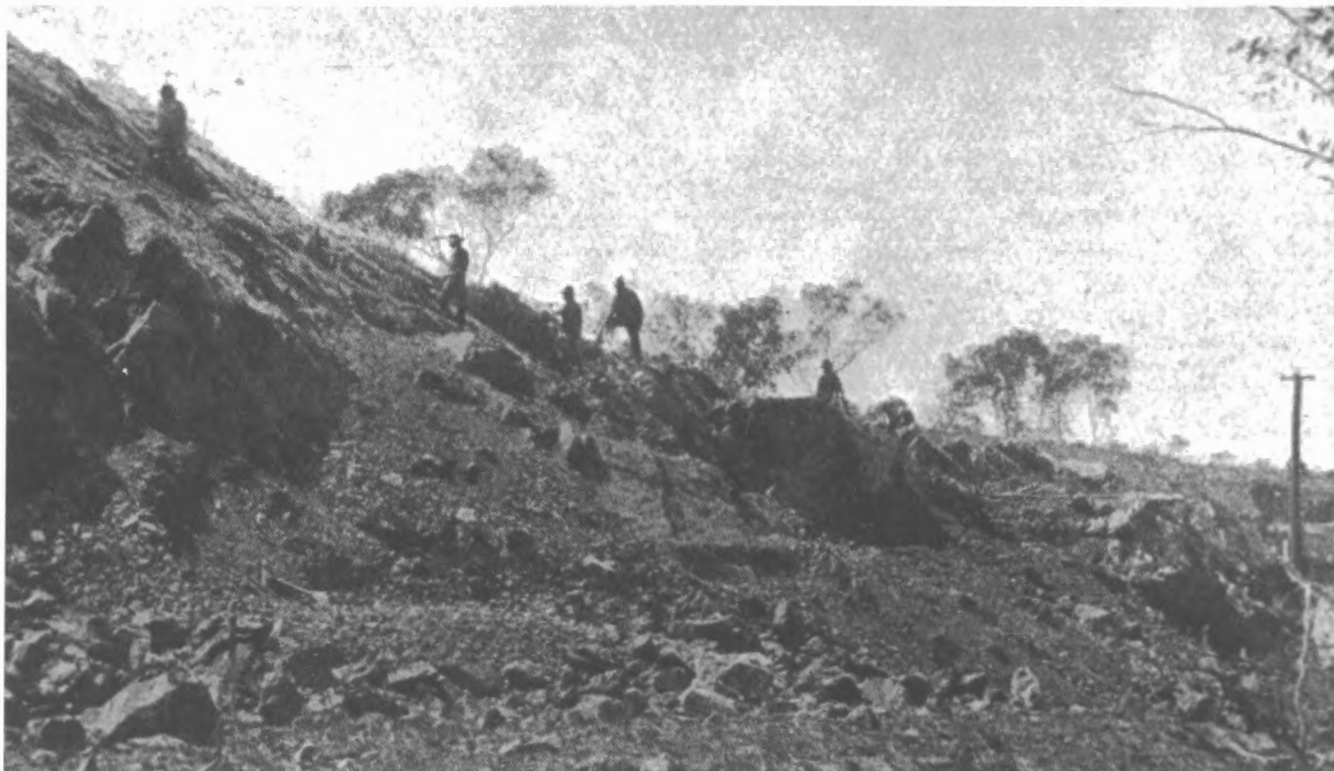
Building the MacGregor tramline, showing the terrain that encouraged the company to choose 2ft gauge.
