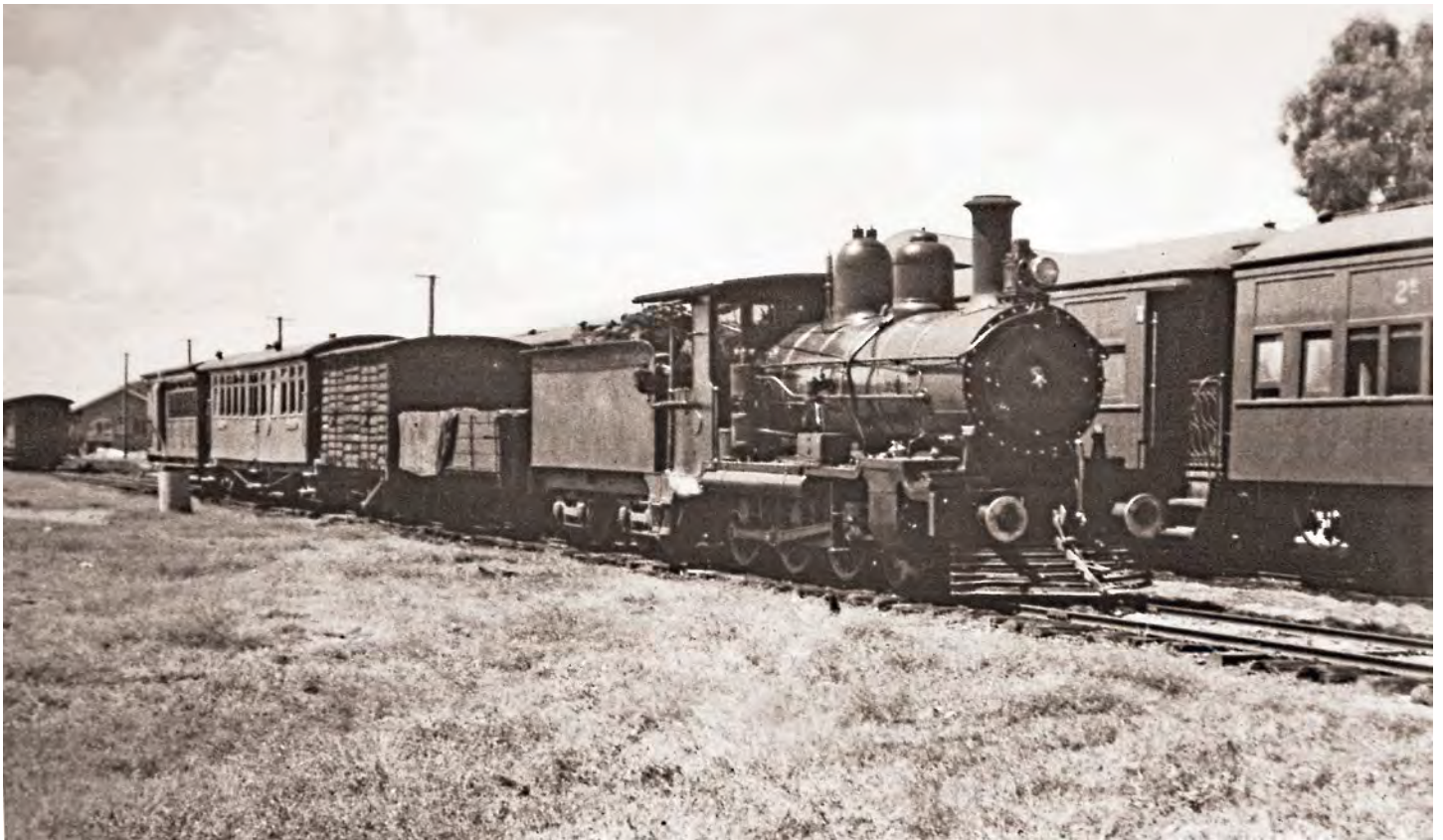
Barcaldine station. Aramac Tramway's No.A1, a 4-6-0 built for them by the QGR's Ipswich shops (b/n 103/1924), ready to depart for another run across the 'black soil plains' to Aramac in the 1950s. The carriage and combination van are the tramway's entire passenger accommodation and in the early years would be supplemented only when absolutely necessary by carriages hired from the QGR. Initially, the charge for using Barcaldine station was such that the Tramway considered building their own station. Photo: courtesy ARHS Queensland 1959 filmstrip, PICT0023
