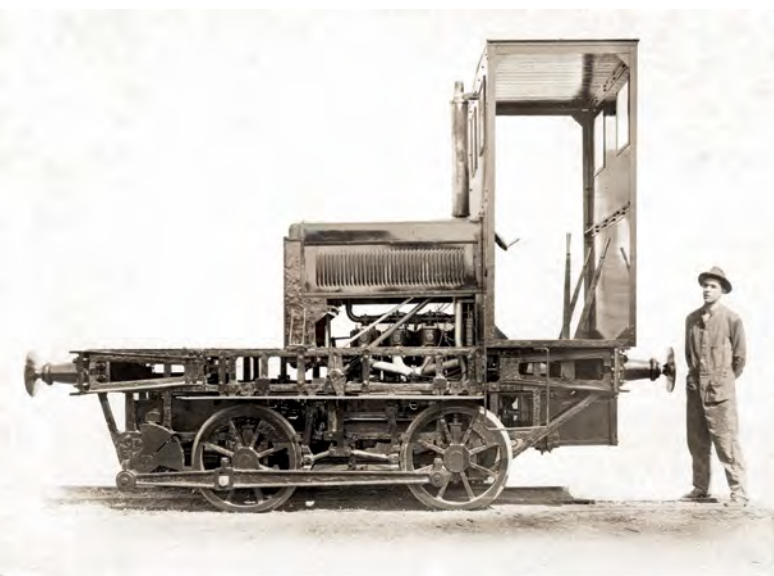
Builder's photograph of the ungainly-proportioned 0-4-0PM locomotive built for the Nepean Dam construction project. This photograph was selected for use on company advertising post cards.
