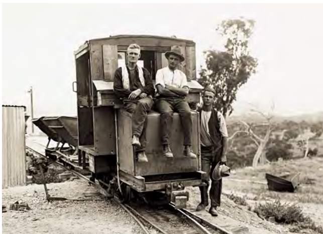
Three workers pose with the Purcell locomotive and skips, Mugga quarry. Note the homemade sandbox made out of old gelignite packing cases from Ardeer, Victoria. Photo: Alexander Collingridge, National Library of Australia obj-142653501LA
