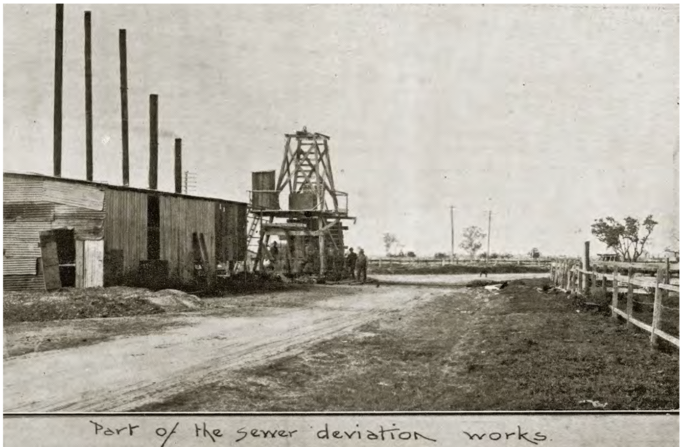
The headframe and powerhouse at Shaft 41, Pinkenba, at the eastern end of the Dunlop Deviation, looking east. The tramway was on the other side of the power house.
