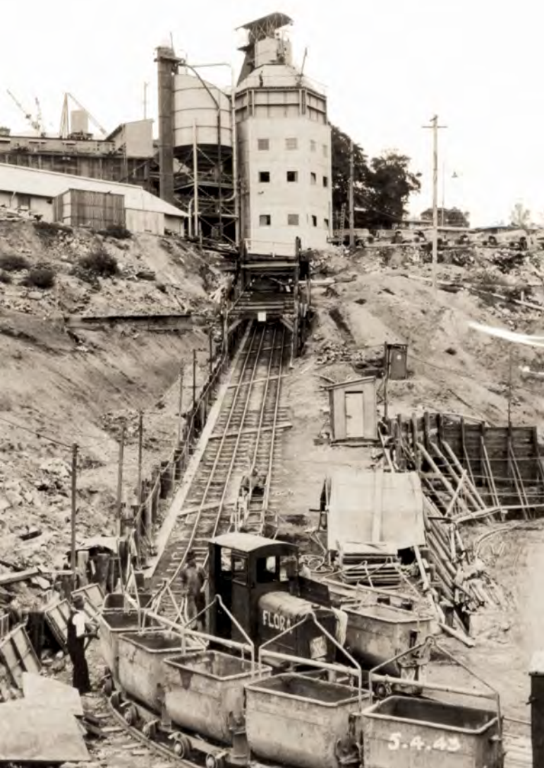
Flora at the base of the double-tracked incline descending down from the concrete mixing plant at the Captain Cook Graving Dock site, 5 April 1943. Two rakes of empty concrete trucks stand on track on either side of the locomotive. Photo: State Records NSW CGS 12490. 6/4496, 203
