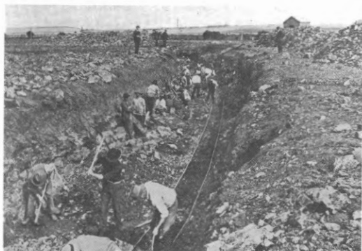
Excavating the railway cutting for access to VR lines, Corio Quay, 1909.
