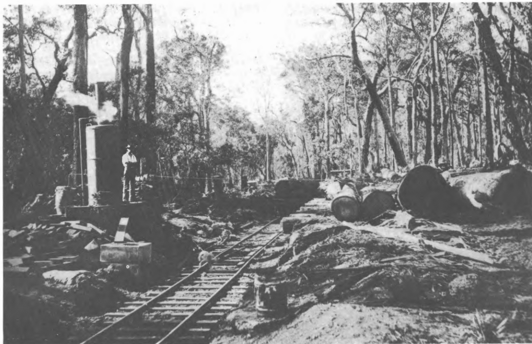
Vertical boilered winch used for loading logs onto train.
