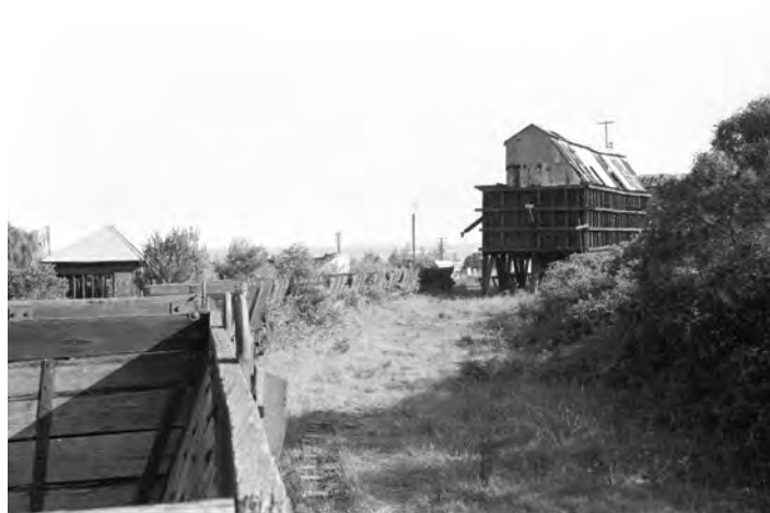
Looking south in the 'Down' direction into the Excelsior Colliery yard with the slack coal box on the right in 1969, the company's standard gauge wooden coal wagons, built by Goninan, were painted Indian Red and lettered 'EK' (Earnshaw and Kirton) in white. There are thought to have been at least 20 of them. Photo: ARHS collection 459289
