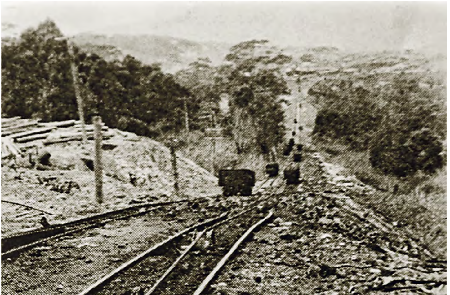
Looking down the endless rope skipway from No.2 Colliery, 1953, Australian Coal, Shipping, Steel and the Harbour, 2 November 1953. There seems to have been a spill of coal covering the track for the descending full skips. Photo: Ross Mainwaring collection
