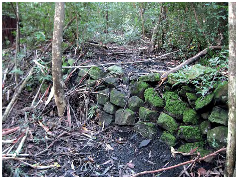
Above: Bricking up the mine portal with an Atlas battery electric locomotive standing by, March 1962, facebook, accessed 12 July 2023. (Some of the men in the photograph are gradually being identified by name – check facebook for latest results.) Below: An intact dry-stone wall supporting the No.1 skipway not far from the convergence points with No.2 skipway above Kirton Siding screens in May 2023, It has been 77 years since a set of coal skips passed this way. Photo: Ross Mainwaring
