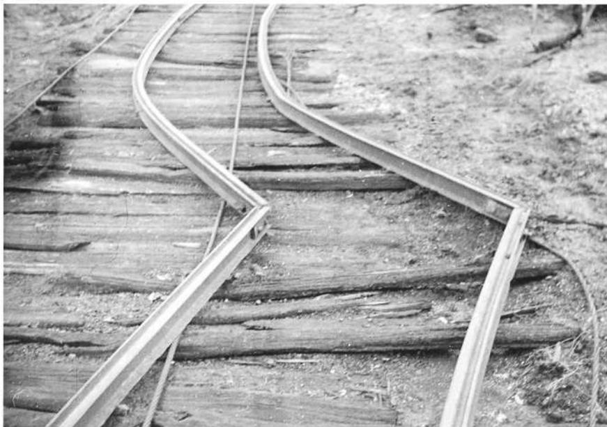
Rails (ex cable-tram ?) on Ada side of High Lead, buckled by bushfire. June 1939.
