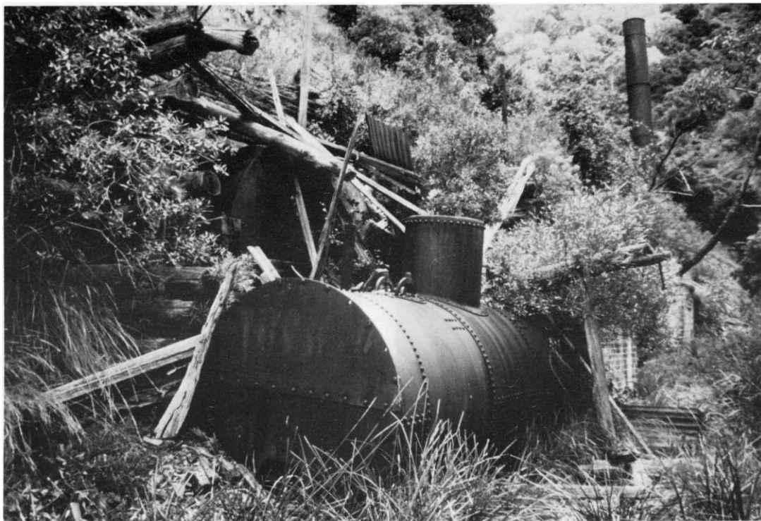
Ruins of the West Sunlight Mine, with boiler and shaft winding engine on the left, beneath the timber, in 1985. Photo: author
