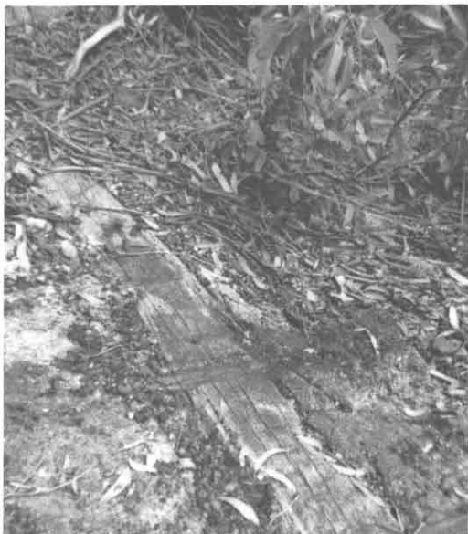
Sleeper at commencement of incline. Note the spikes and cable marks. Taken January 1974.
