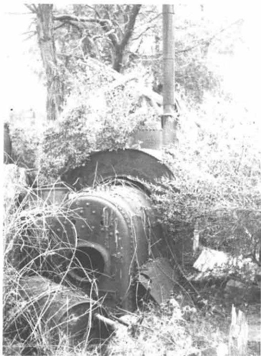
Well hidden from casual observation. The boiler and saddle tank of Davenport 2ft gauge loco No. 1595 as seen at the Cleary farm in January 1979.
