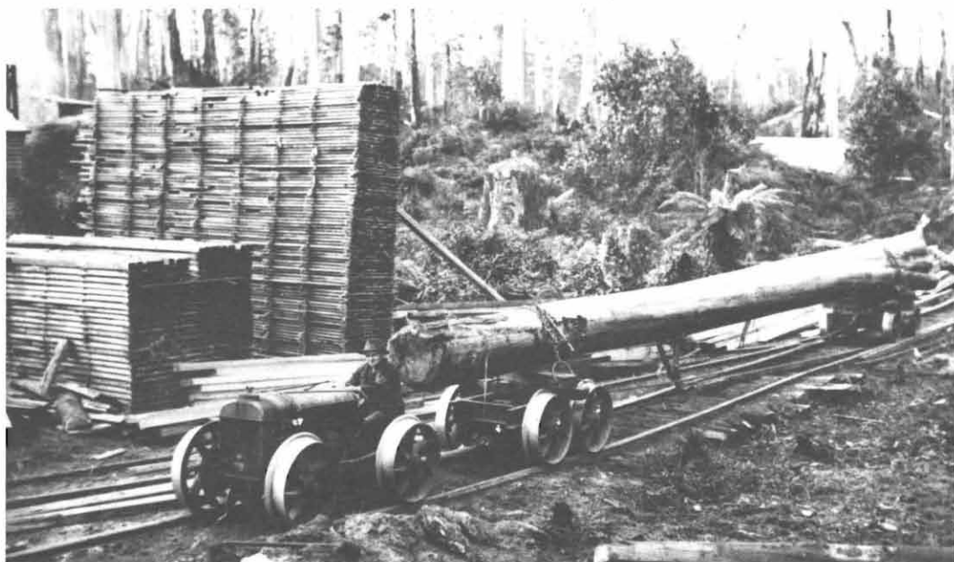
Photo shows a Fenton log tractor hauling a log jinker on sawn timber rails at Salmon River, Tasmania.
