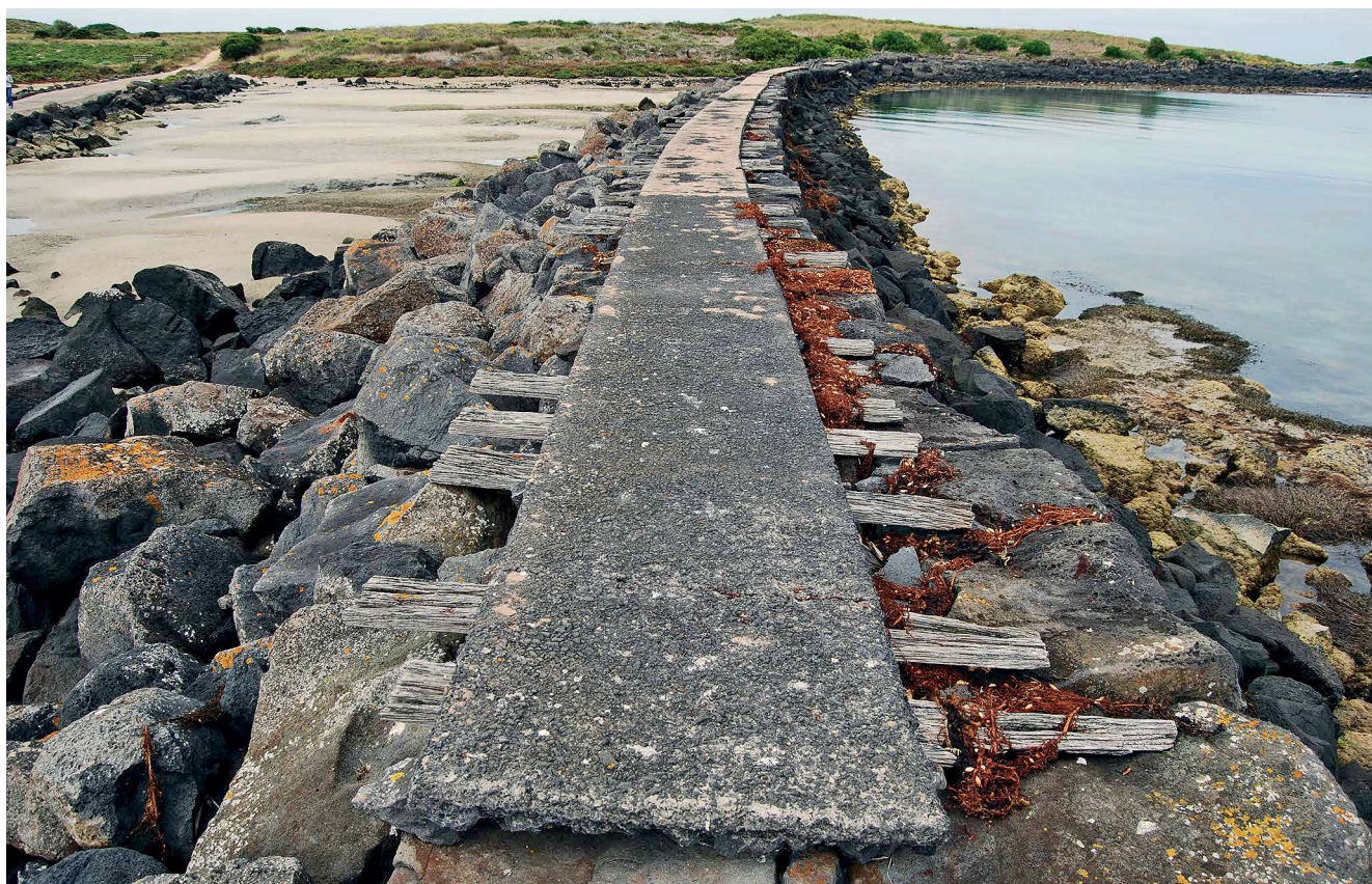
The tramway formation along the eastern wall of the South West Passage, showing the timber sleepers intact under the concrete capping. Photo: Peter Evans
