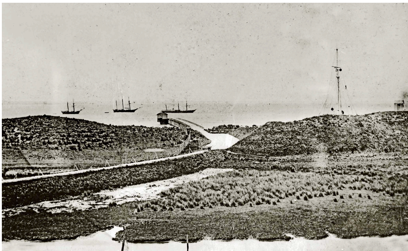
The earliest known photograph of the jetty and tramway as they were in 1861. Features of note are the ships moored in Port Fairy Bay, the lifeboat shed on the jetty, the shallow cutting through the dunes (with a tramway truck visible), and the long embankment leading to the River Moyne. The only other sign of activity on the sand dunes is the signalling flagstaff to the right of the tramway cutting (later the site for a battery of guns to defend the port). Photograph by J. S. Adcock, courtesy Port Fairy Historical Society, image 62-09A-001.
