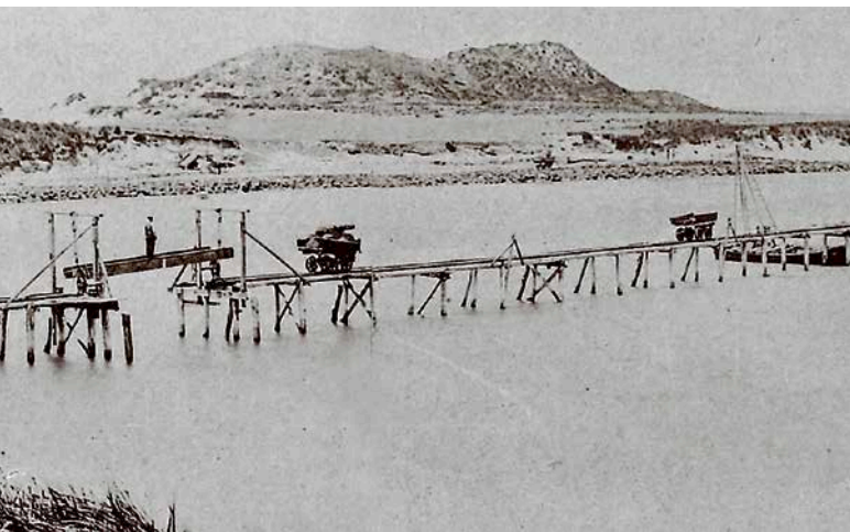
A detail of the 1870 photograph showing the manually-operated lift span with its twin crab winches, and details of the trucks used on the tramway. Note a third truck on the original south training wall.
