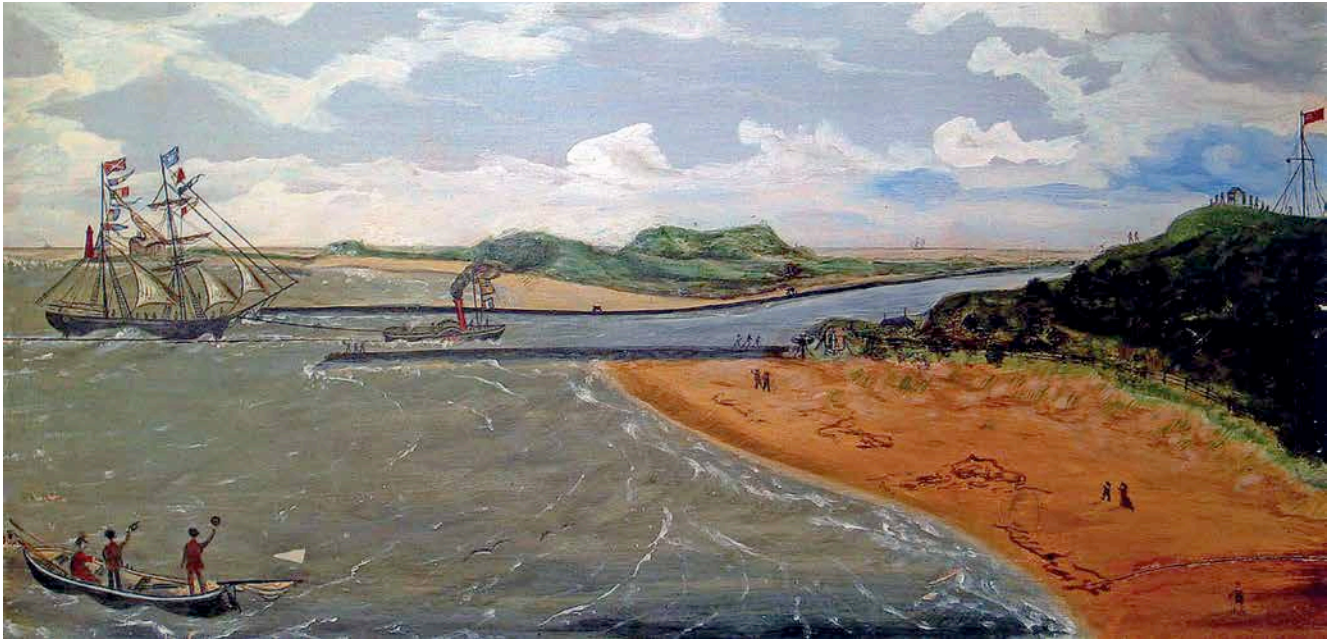
The steam tug Surprise towing the topsail schooner Elizabeth (62 tons, 64 ft long, built in Tasmania in 1851) upstream through the still under-construction training walls on 29 May 1872. The Elizabeth drew 6 ft 6 in of water and was fully laden with general cargo, so the exercise demonstrated beyond doubt the efficacy of the new harbour works.
