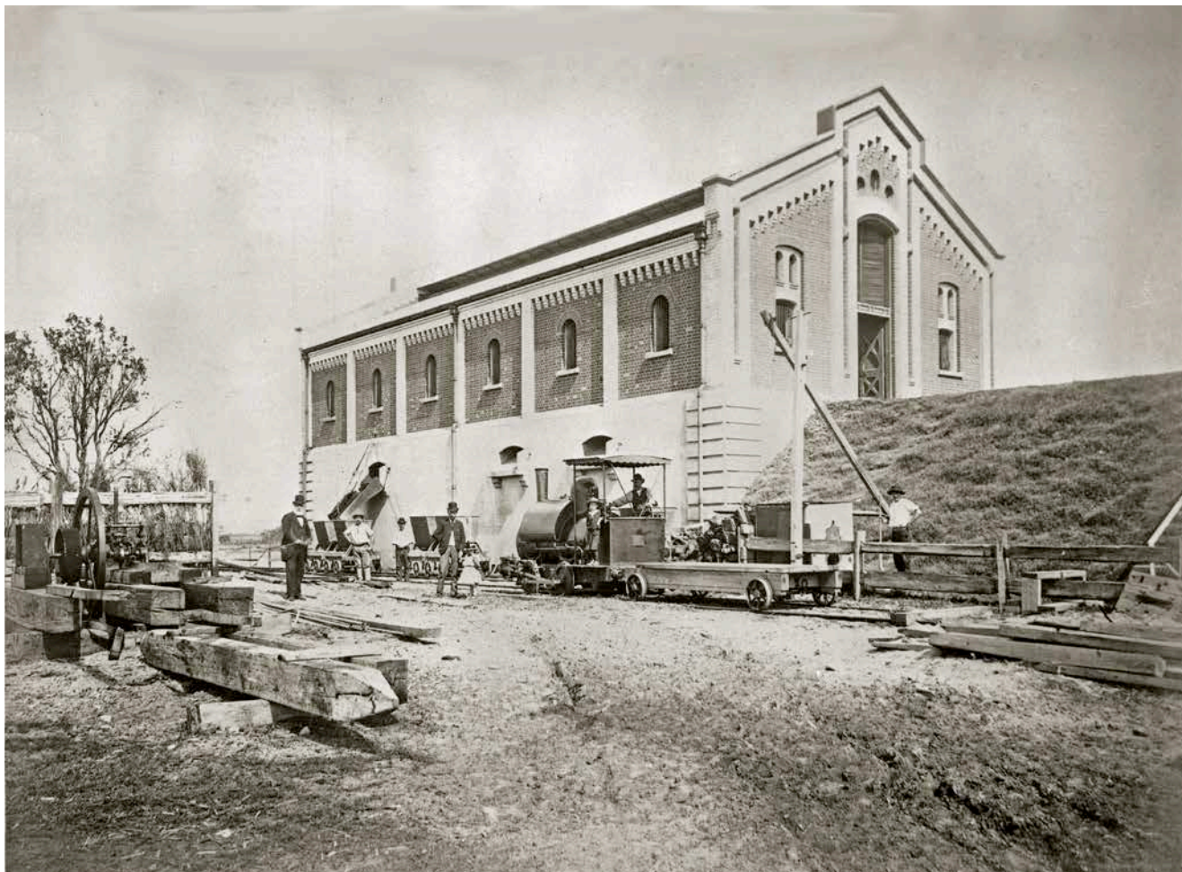
Mort's Dock locomotive and nondescript flat truck on the works siding near the Inlet House. Note the builder's plate on rear cab wall – the only Mort's Dock small industrial locomotive known to be fitted with one.
