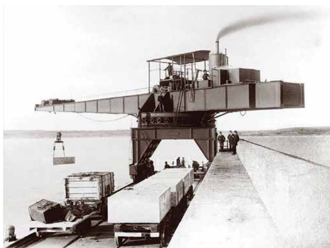
Left: The blocks from Laws Siding being placed into position for the Breakwater Pier extensions. The Titan crane had the capacity to lift the 30, 22 and 20 ton blocks used at different times in the pier construction. Photo: State Library Victoria Right: Laws Siding site in 1926, having been removed in 1916 so there is not much left to see. The turnout and approach line from the road corner has been obliterated by sandy soil movements over the intervening years. The white strips are concrete pads laid on each side of the rail siding for the travelling crane to move along when lifting the concrete blocks onto the rail dollies. The rabbit siding was on the same site, probably the same turnout being used for Laws. The rabbit factory itself was to the right in Stanley Street, out of the picture, and not far from the road bridge. Photo: FL 10083545 State Library Victoria
