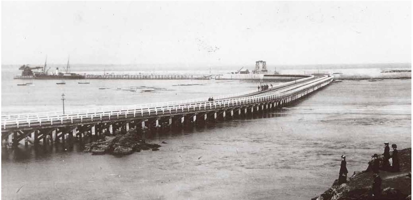
The viaduct crossing the waters to the pier. The coastal waters are freely circulating under and through the viaduct, as was their natural disposition. It was when these flows were cut off after 1914 that the harbour began silting up. The crane at the end of the pier is working on extensions and was not a permanent feature.
