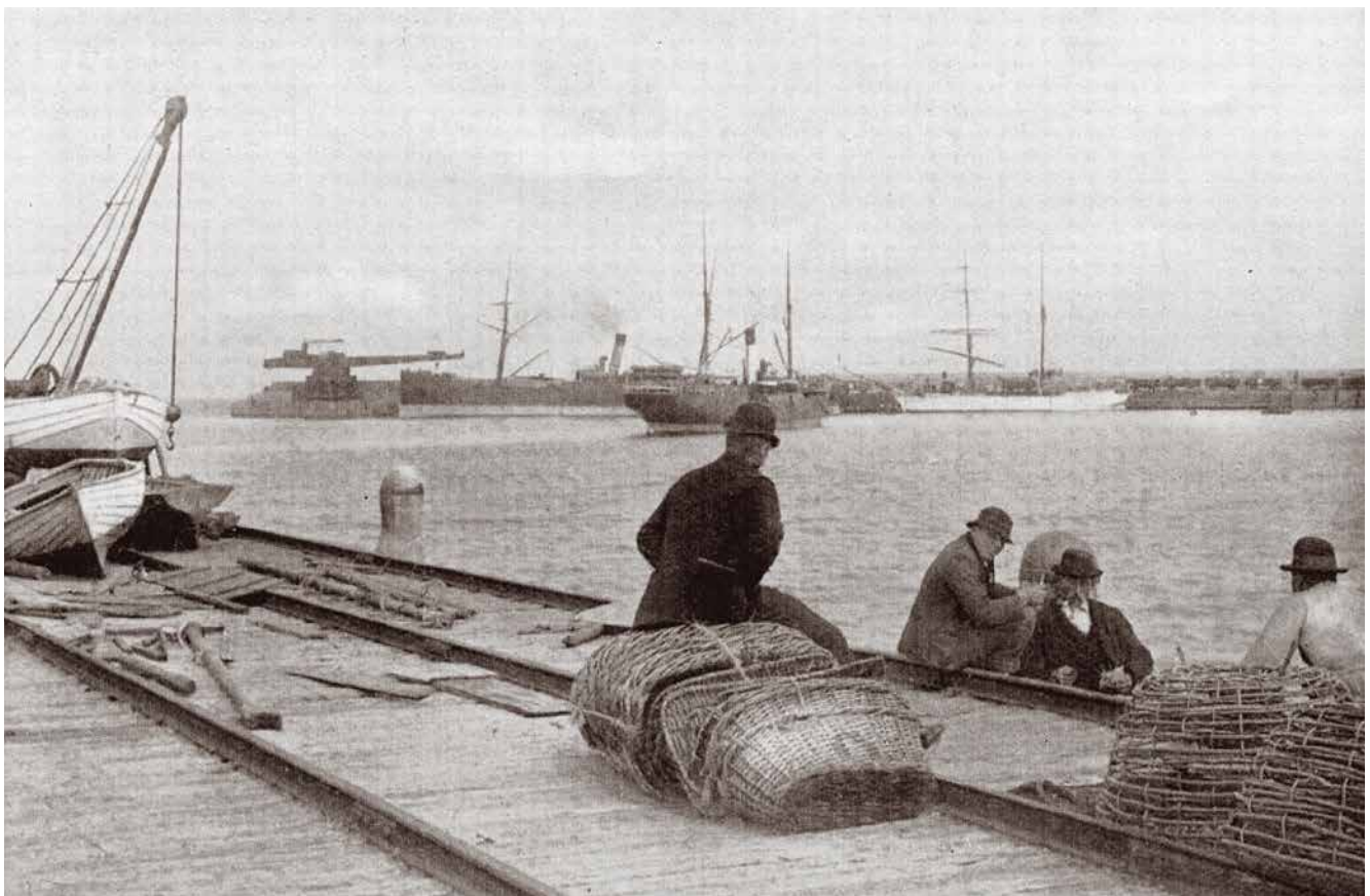
Tramway jetty in its later years, circa 1905, when no longer used by the tram. The 'four foot' rails can be seen in the centre and with the transfer gantry rails on the outer edge.
