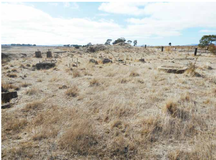
Machinery zone on the 'island'. The twin humped mound in the background is the remains of the loader ramp. Originally the ramp was straight sided supported by metal slabs and timbers but these were removed when the site closed. One circular well can be seen on the right and there are two more water pits further around.
