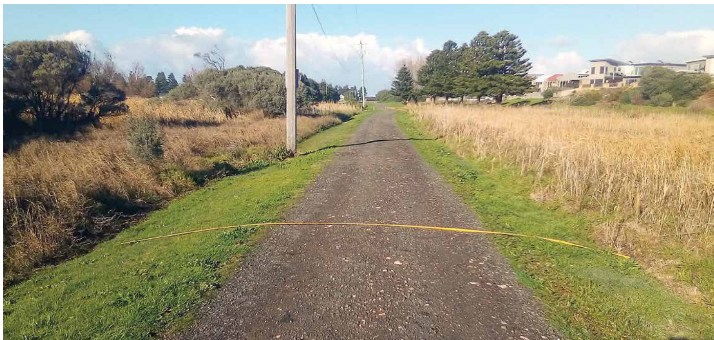
Typical cross section of the formation as it crosses the swampy bits of Lake Pertobe. The formation could be up to a metre high. The running road- bed was as wide as it was to allow for horses and pedestrians to walk alongside the tram 'four foot'. Photo: N Houghton
