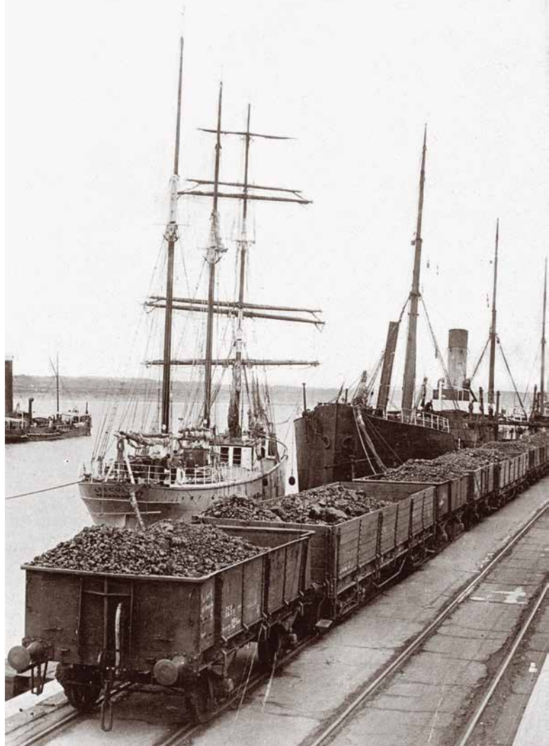
Above: Discharging coal from ship to rail. The coal is lifted from the hold in baskets/slides and taken across a gangway or slide where it is dumped into the rail truck. A dredge can be seen in the left background. Photo: State Library Victoria
