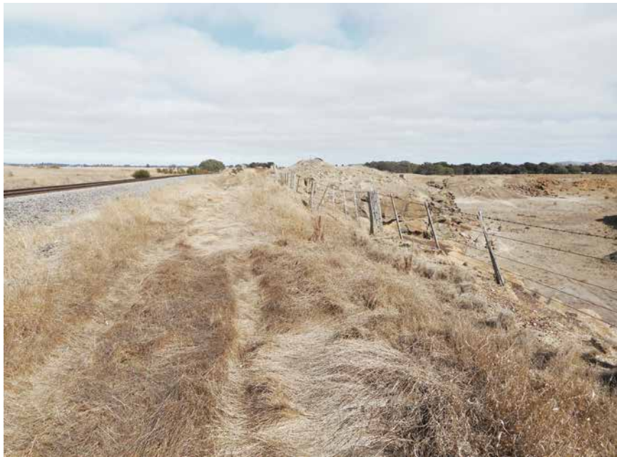
Looking south along the loop siding site at CRB 1. Quarry hole to the right. The quarry stone was loaded onto rail at a ramp and chute, the remains of which are represented by the mound. At this ramp site, out of picture on the other side, was the quarry engine, crushers and screens, all placed on the level ground next to the railway fence. Remains of two small huts can also be seen there. The quarry was formed on three sides around this machinery sector so it sits on an 'island'.
