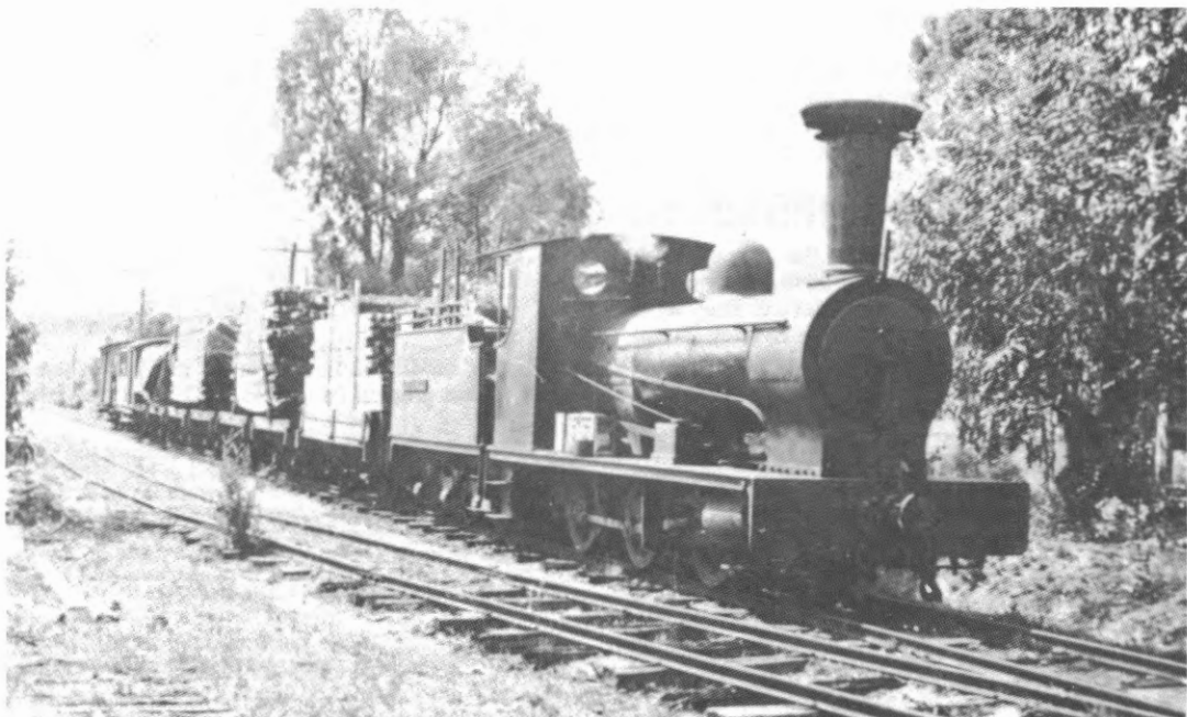
The locomotive Powellite, as fitted with a Cheney Patent Spark Nullifier in the 1930s, heads for Yarra Junction with a train of timber. Photo: LRRSA Archives
