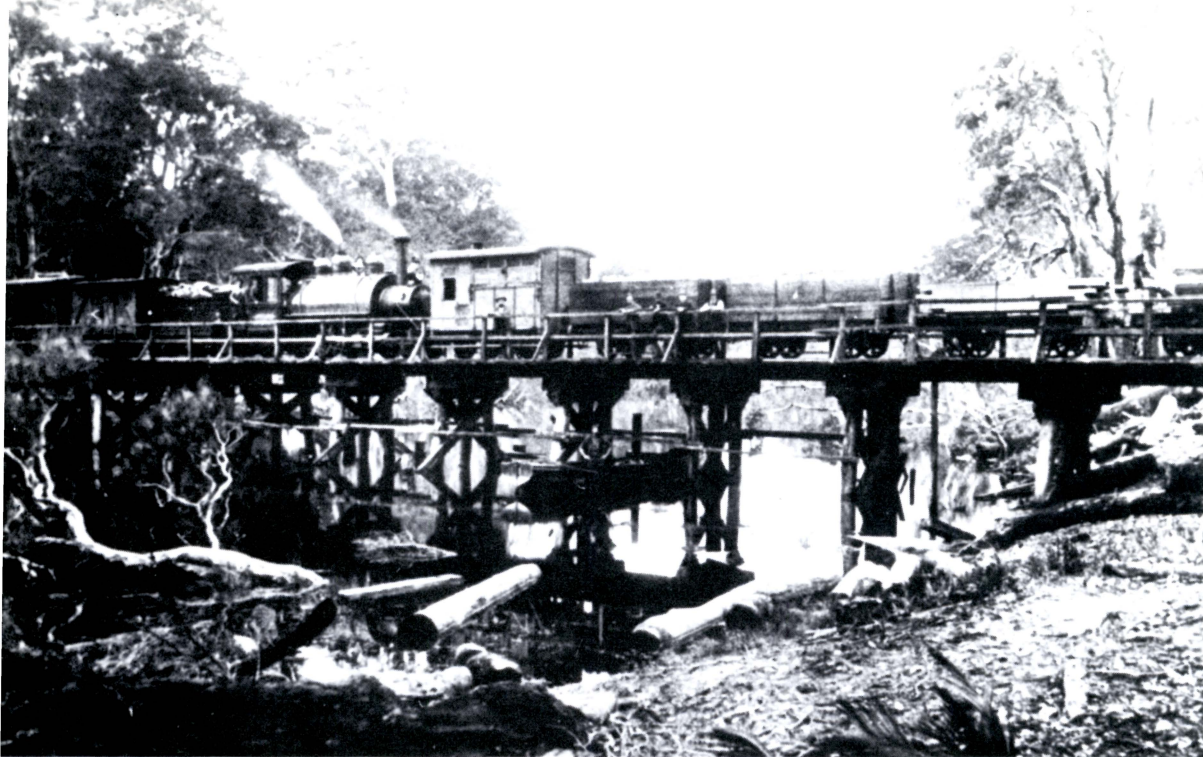
A train hauled by a 2-4-2ST&T locomotive crosses the Denmark River, on Millar's Elleker — Denmark railway, about 1896.
