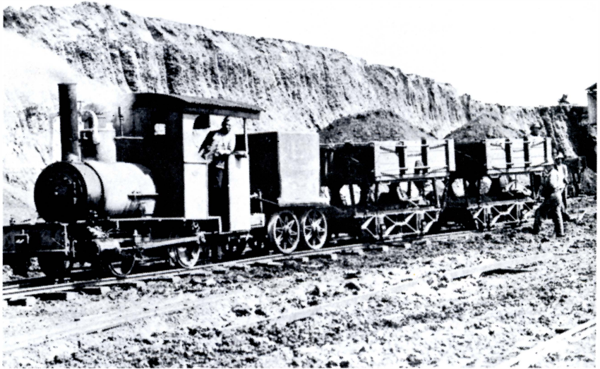
Baldwin 0-4-0 locomotive at work on the Hume Reservoir Construction. This locomotive is believed to have come from Hayden's Barwon Downs Tramway.
