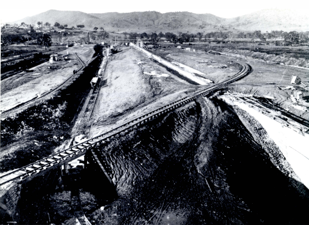
A general view of the Hume Reservoir main embankment construction site. Note the 2 foot gauge horse-hauled line under the bridge. On the right-hand side, in the distance, is a Perry locomotive on a rake of six trucks.
