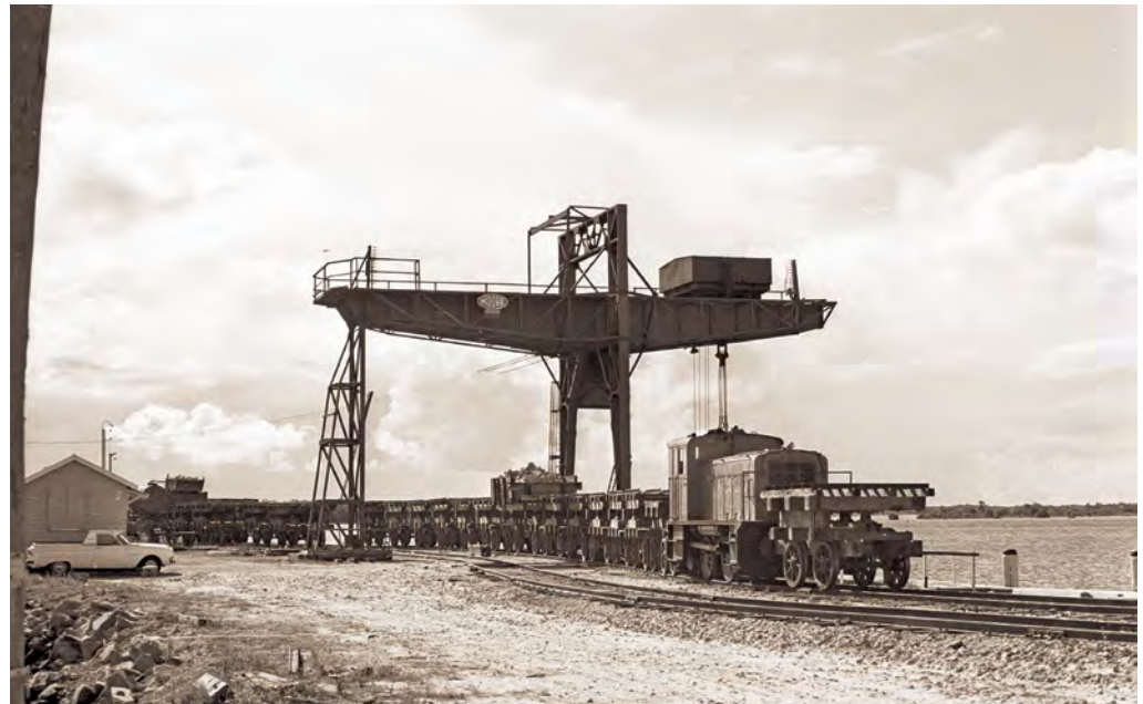
Number 82 and train at the Malcolm Moore portal crane on the Yamba wharf where stone or concrete blocks were transhipped from water to rail transport. Of interest is the timber crate containing loose rubble on top of one of the trucks. September 1969. Photo: Alex Grunbach courtesy ARHSnsw
