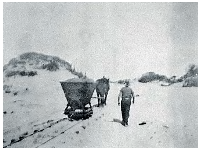
Before the diesel locomotive arrived in early 1937, horses were used to haul single tramway skips filled with black sand back to the treatment plant. Bill Derrick collection
