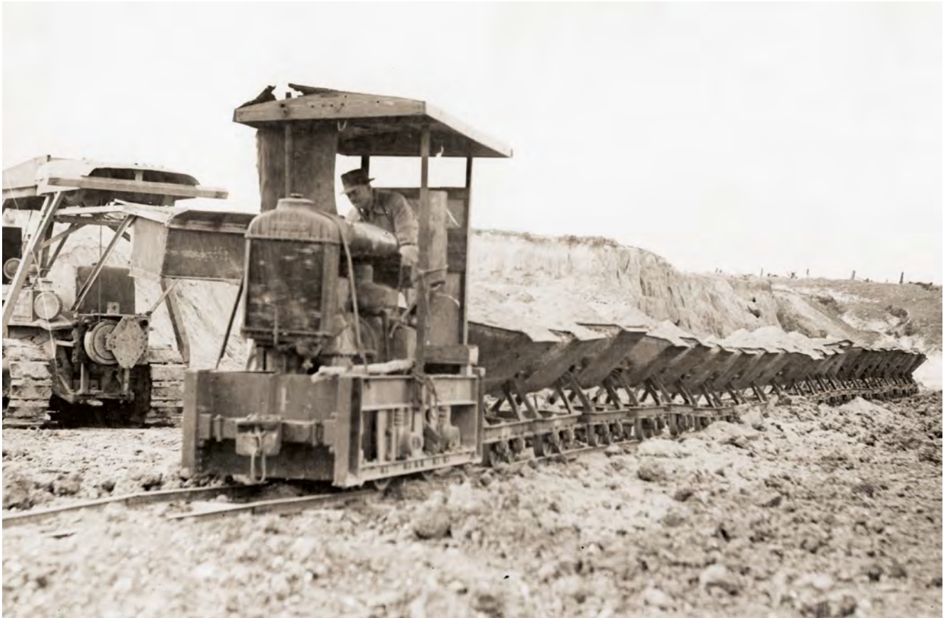
Above: The E&WS Fordson-engined Malcolm Moore locomotive number 4 with its train at the loading area. Note the Cat 7D9 with the Le Tourneau loader in the background near the locomotive.
