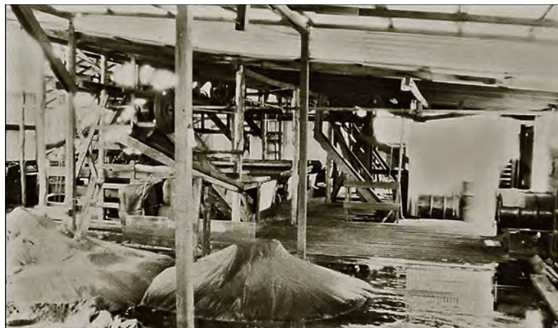
A small elevator stacker, fitted with a swivelling chute, dropped soaking wet concentrates produced by the Wilfley Tables onto piles on the shed floor. When partly dry the shed crew wheelbarrowed the heavy sand to the main drying area. Bill Derrick collection
