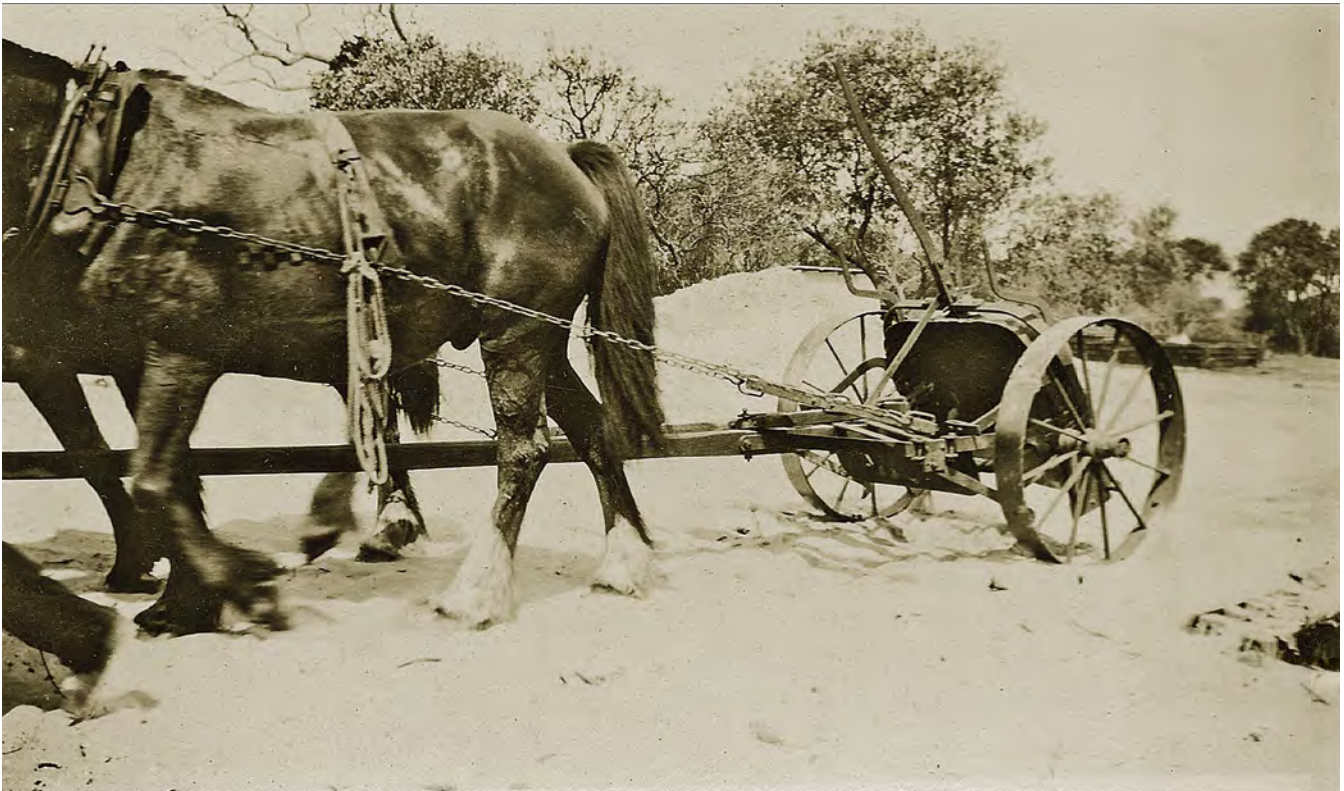
Porter & Derrick used horse-drawn scoops on their beach mining leases, primarily to strip beach sand overburden off black sand deposits. The rear handle controlled the angle of the scoop blade: lowered down when filling the scoop with sand, held horizontal when pulling the loaded scoop to the dumping area, and raised to the vertical to dump the load. It was hard, demanding work for the scoop operator who also held the horses' reins around his neck to control the team. Jan Brown collection
