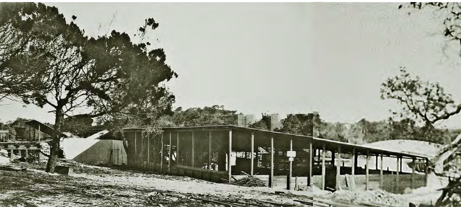
A composite image of the Yamba Treatment Plant circa 1940. The raw sand unloading stage, with a tramway skip standing on top, is on the far left; the rectangular white shape (a corrugated iron structure) beside it is the raw sand feed hopper. On the far right is the waste sand stacker and a large pile of waste sand. The outline of the water storage tanks is visible behind the shed roof. A large part of the shed floor was used to air-dry black sand concentrates. Bill Derrick collection
