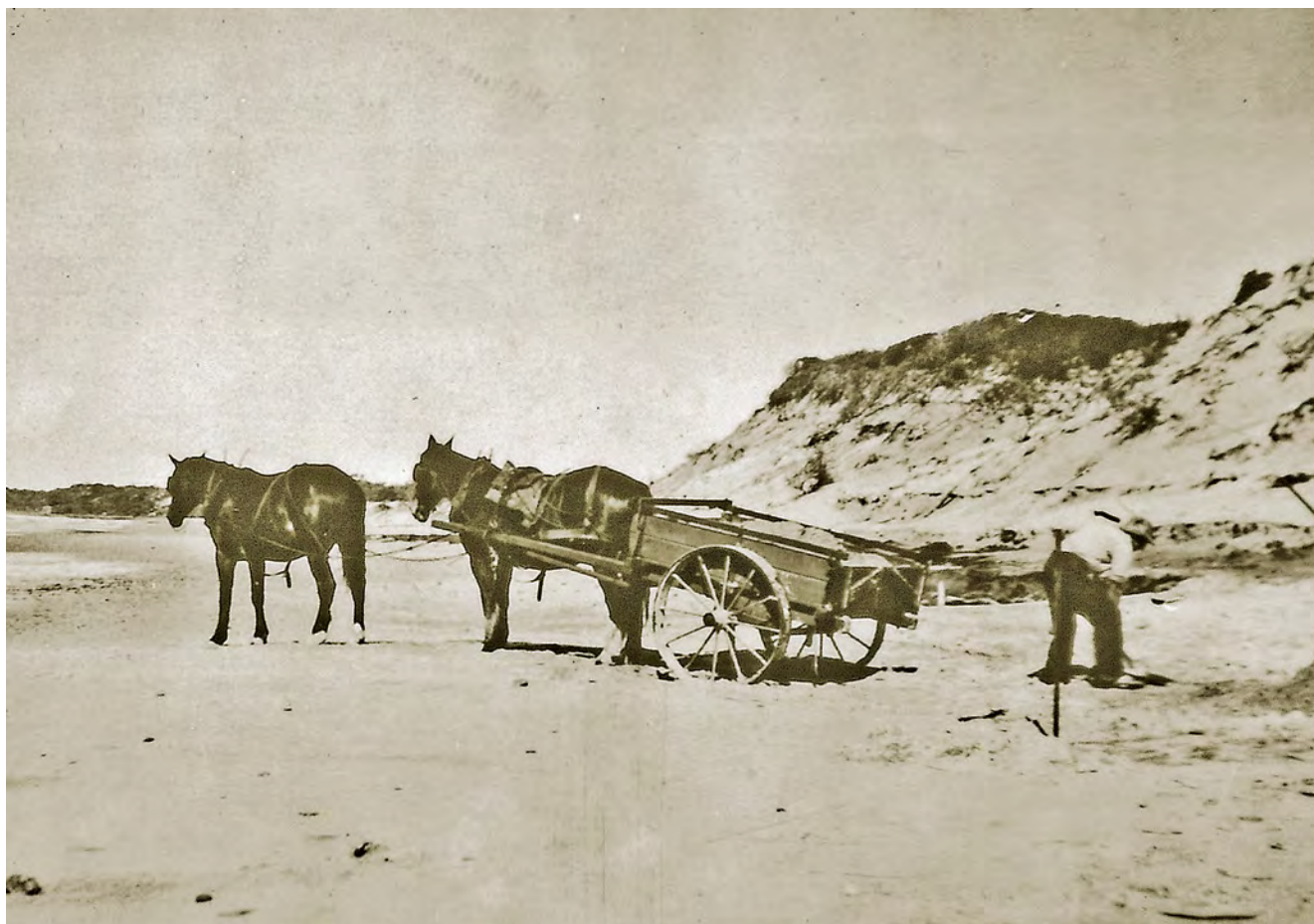
Mining black sand on Barri Beach in 1935. Porter & Derrick employed a horse-drawn cart to haul black sand back to the treatment plant for the first few months of operation. Horse and cart haulage was replaced by horse-drawn mine skips on the newly-constructed beach tramway in early 1936. Bill Derrick collection
