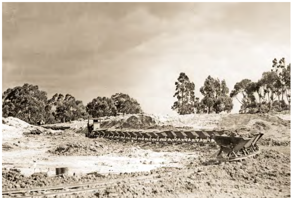
Above: The E&WS Fordson-engined Malcolm Moore locomotive number 4 with its train at the loading area. Note the Cat 7D9 with the Le Tourneau loader in the background near the locomotive.
