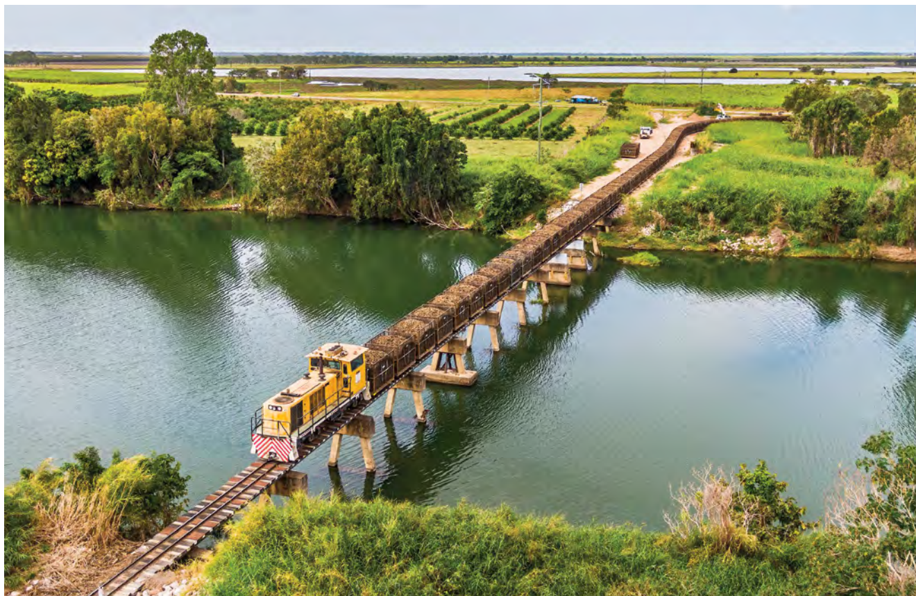
Invicta Mill's Walkers B-B DH Minkom (710 of 1973) crosses the Houghton River bridge on 1 August. Clean up operations after a recent derailment can be seen going on in the background. Photo: John Kirk
