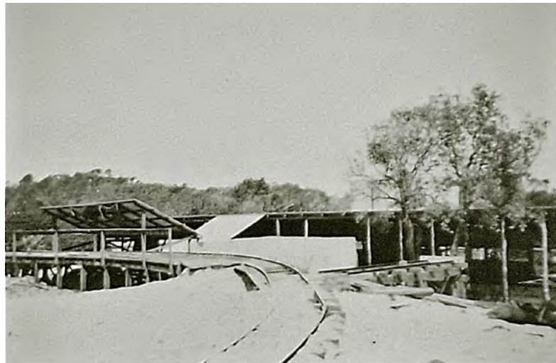
The beach tramway terminated on an elevated timber stage above a sand feed hopper (the white structure) which fed the belt elevator taking sand into the plant. Bill Derrick collection
