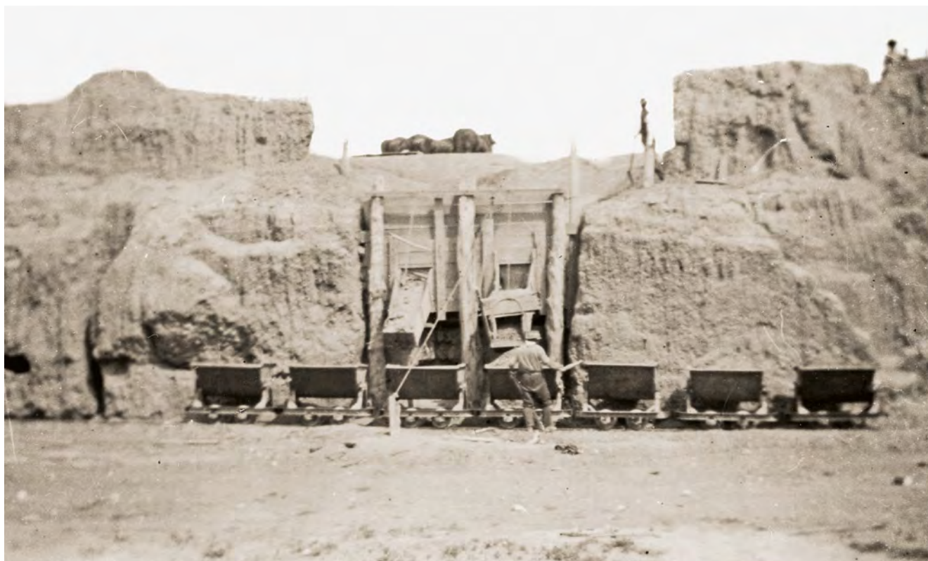
A train being loaded via chutes below bins filled from the cliff quarry above them. This was possibly during repairs carried out after the 1917 flood. 8 Photo acquired from the late J C Morphett (courtesy of Chris Andrews) and dated between 1918 and 1923.
