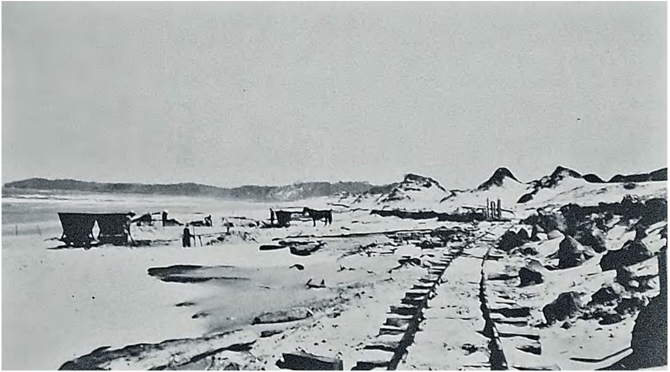
Beach diggings at the northern end of Porter & Derrick's lease on Pippi Beach, Yamba. The 2km-long beach tramway ran south to the treatment plant at Barri Beach. Workmen are shovelling black sand into tramway skips stabled on short temporary spur lines. Bill Derrick collection
