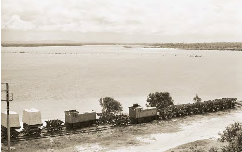
The passing loop on the Yamba side was situated close to the location of the original Yamba quarry – the sign indicating that camping is prohibited. Number 83 pauses in the loop while its driver watches number 82 pass with concrete blocks ready for tipping. Both locomotives have a “runner wagon” fore and aft to reduce the risk of damage should a tipping mishap occur. Number 83 has the roof-mounted oil drum but number 82 appears to have roof mountings for the same purpose. September 1969. Photo: Alex Grunbach courtesy ARHSnsw
