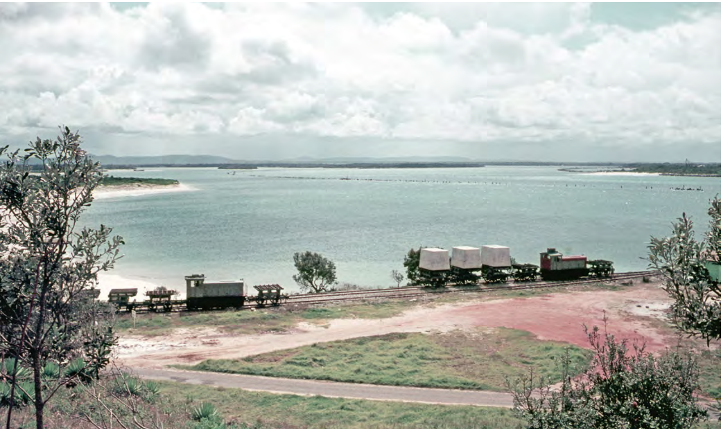
Number 83 leaving the passing loop at the old quarry site with its load of 40-ton cast concrete blocks. The view beyond is up river with the wharf crane at Iluka on the extreme right in the far distance. The timber piles of the Middle or Freeburn Island training wall are just visible above the surface of the water. September 1969. Photo: Alex Grunbach courtesy ARHSnsw
