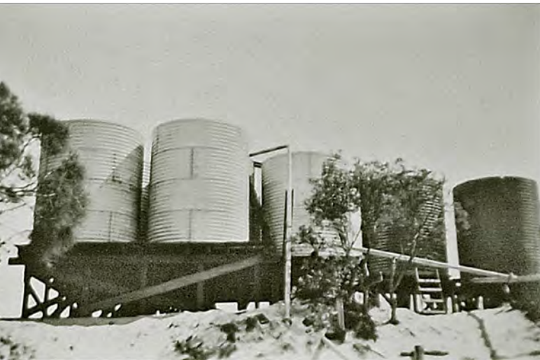
The treatment plant required a steady supply of fresh water to operate the Wilfley Tables. This was pumped from nearby Riley's waterhole into a battery of ten corrugated iron water storage tanks set on a sand hill behind the plant. Water gravitated down a pipeline to the plant. Bill Derrick collection
