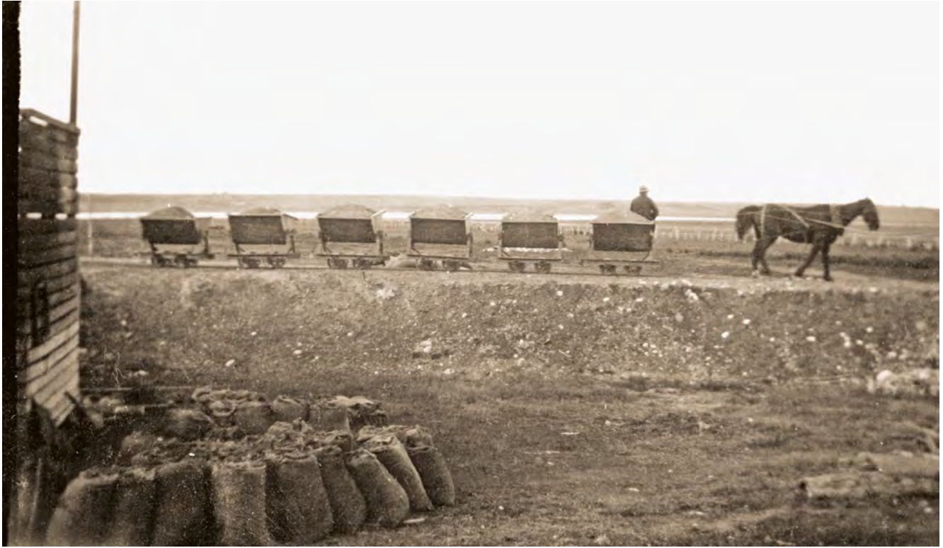
A loaded horse-hauled train heads to the embankment for the repairs. Note the Murray River in the background. Photo acquired from the late J C Morphett (courtesy of Chris Andrews) and dated between 1918 and 1923.
