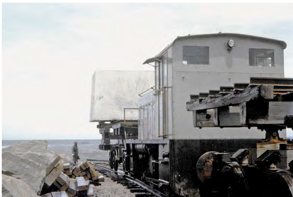
Number 83 at the Iluka tip end. The 40-ton concrete block manufactured at Ilarwill is about to be launched off the end of the breakwall. 2 December 1965. Photo: Peter Neve
