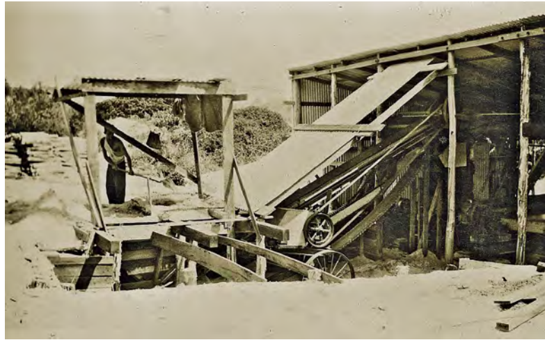
A small conveyor transferred raw black sand into the treatment plant, raising it high enough to gravity-feed onto the Wilfley Tables. Labourers shovelled sand onto the conveyor for the first few months, until the beach tramway was commissioned. Jan Brown collection
