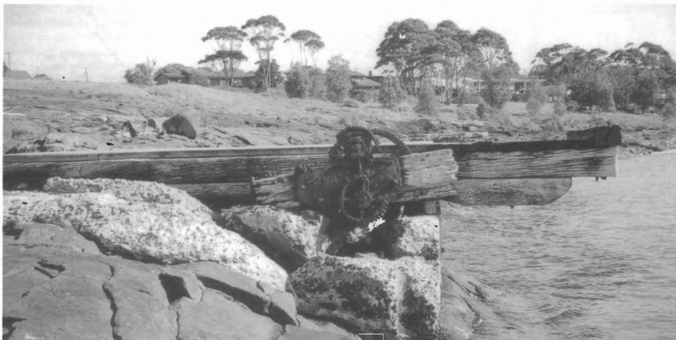
The Bawley Point wharf and winch that drove the endless rope used to move sawn mixed hardwood timber from the mill offshore to anchored steamers of the Illawarra Steam Navigation Company (the old Pig and Whistle Line) for shipping to Sydney. Photo: Ian Bevenge
