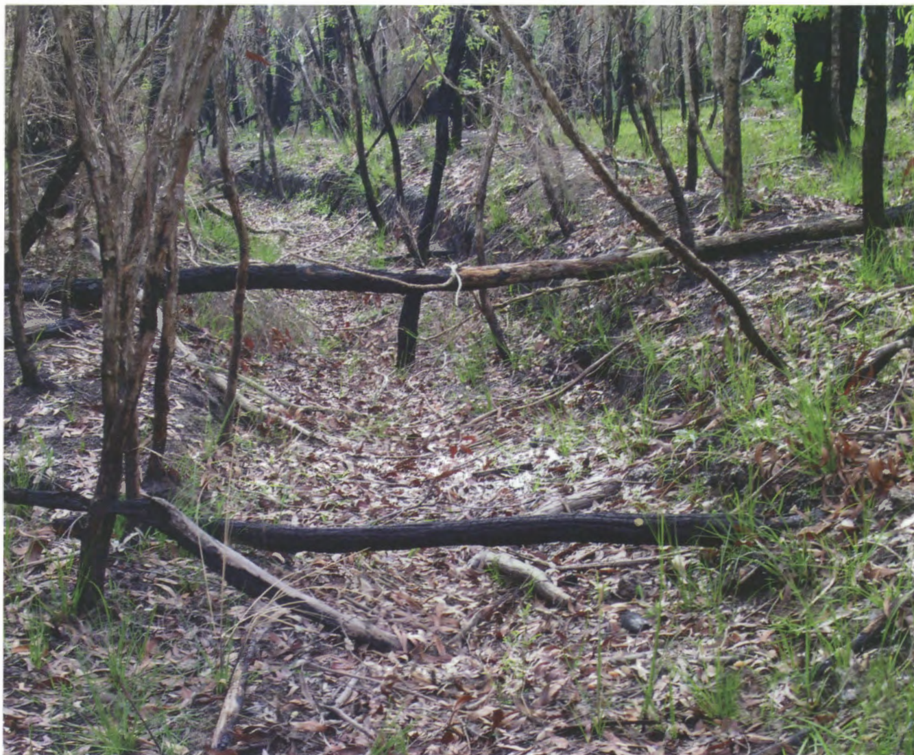
Kirchhubel's log tramway was well constructed with many shallow cuttings and low makeups to provide even grades and curves for the Day's tractor that worked the line. This cutting on a curve was photographed about 200 metres south of the Seninis Track crossing. 20 May 2006.
