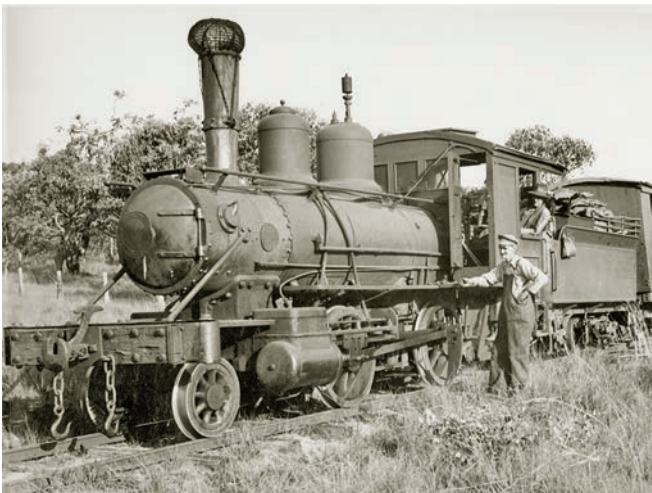
The Powelltown tramway had six steam locomotives. Little Yarra (Baldwin, USA No.37718 of 1912), pictured at left, and Powellite (Bagnall, England No.1965 of 1913), pictured at right, were mainly used between Yarra Junction and Powelltown. Both were bought new by the VPWPL.
