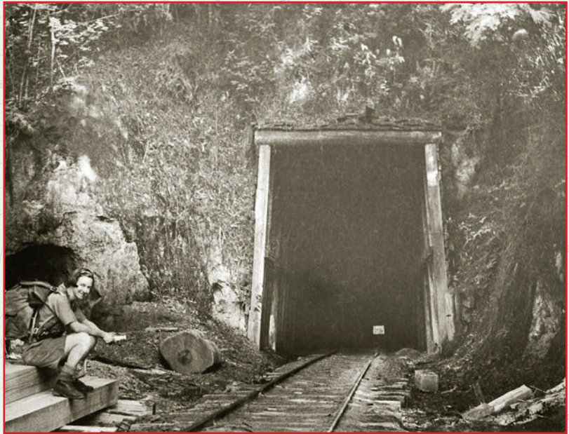
The west (Powelltown) end of the Bump tunnel in 1937. The hole in the embankment on the left was excavated to provide track ballast. AR Lyell
