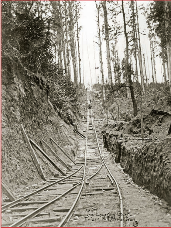
The foot of the west (Powelltown) side of the Bump incline, about 1918. In 1926 it was replaced by a 317 metre long tunnel. Rev. Brenton
