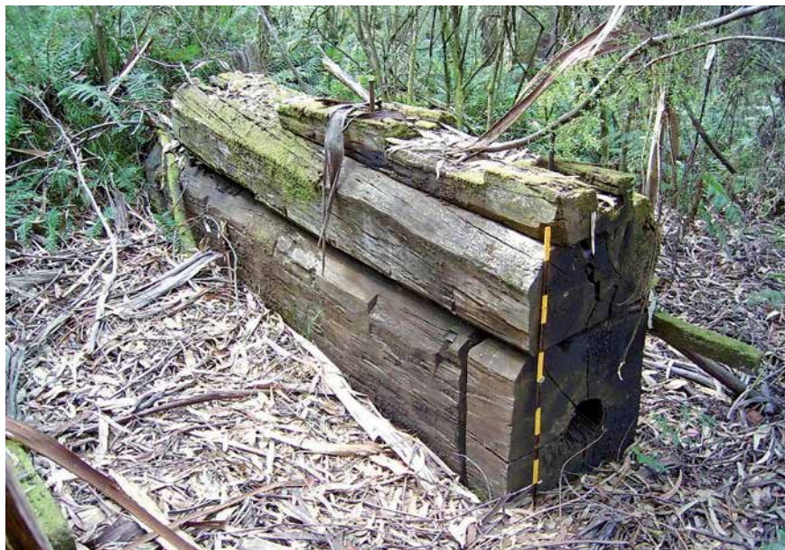
A: Heavy timbers and holding-down bolts making up part of the engine foundations at the Taggerty Sawmilling Company site on Buxton Spur (as it was in May 2005). Photo: Peter Evans
