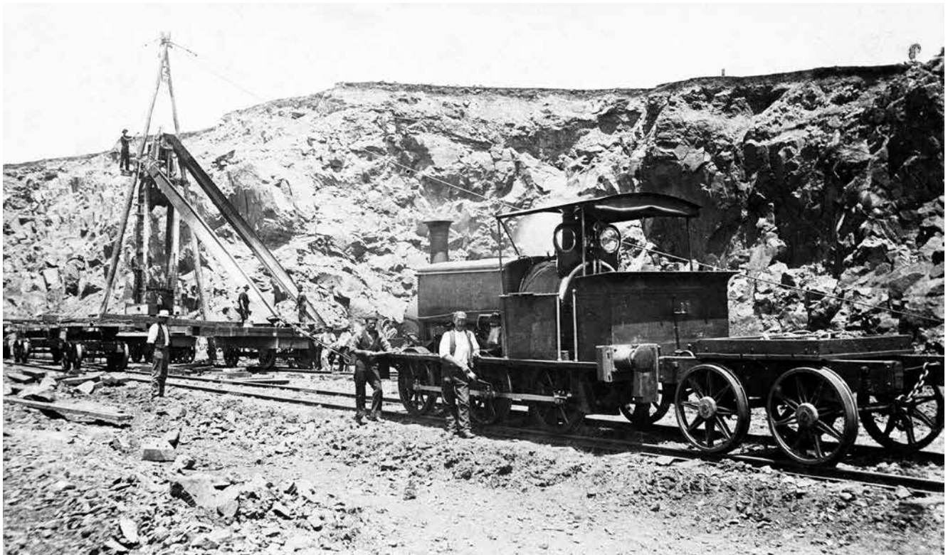
Manning Wardle 0-6-0ST (163 of 1865) at the first Port Kembla breakwater colliery, shortly after its transfer from the Clarence River. "The line from the quarry to the new breakwater at Port Kembla is finished and the locomotive and train of trucks, spick and span, stands ready for steam up 27 July 1901." E. Ellis. Photo: Bruce Macdonald collection
