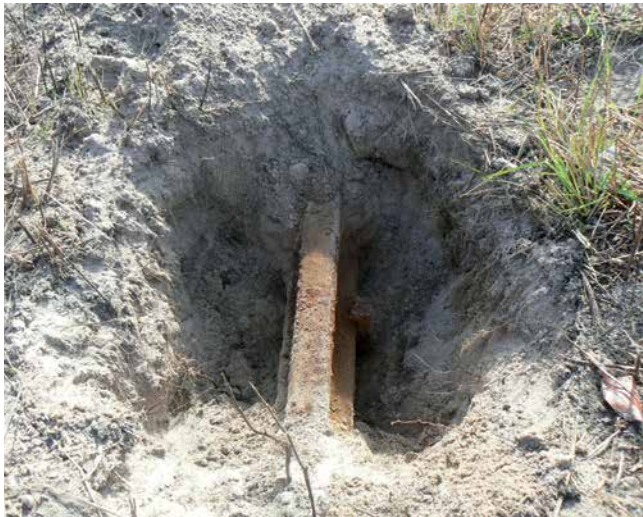
60lb rails with dog-spikes still in situ were found buried under sand on the Iluka Peninsula. They were in remarkably good condition considering they had been there for over 100 years. Photo: Ian McNeil
