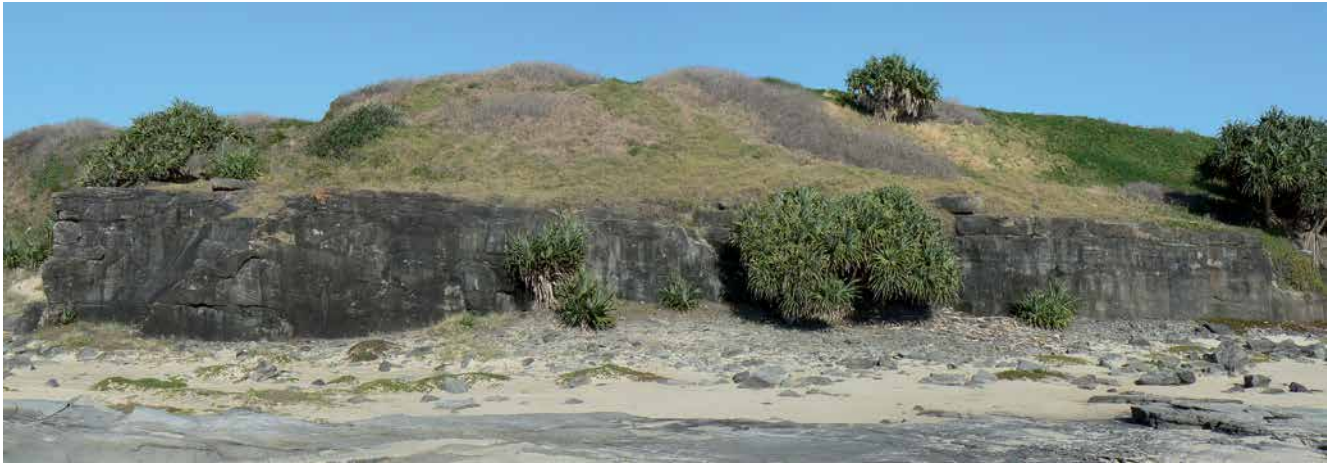
A panoramic view of the headland quarry face at Middle Bluff. Although a much smaller headland than Iluka Bluff one mile to the south, its hard blue sandstone could be quarried out in large blocks suitable for breakwater construction. The remnant hill is a shadow of its former self. Photo: Ian McNeil
