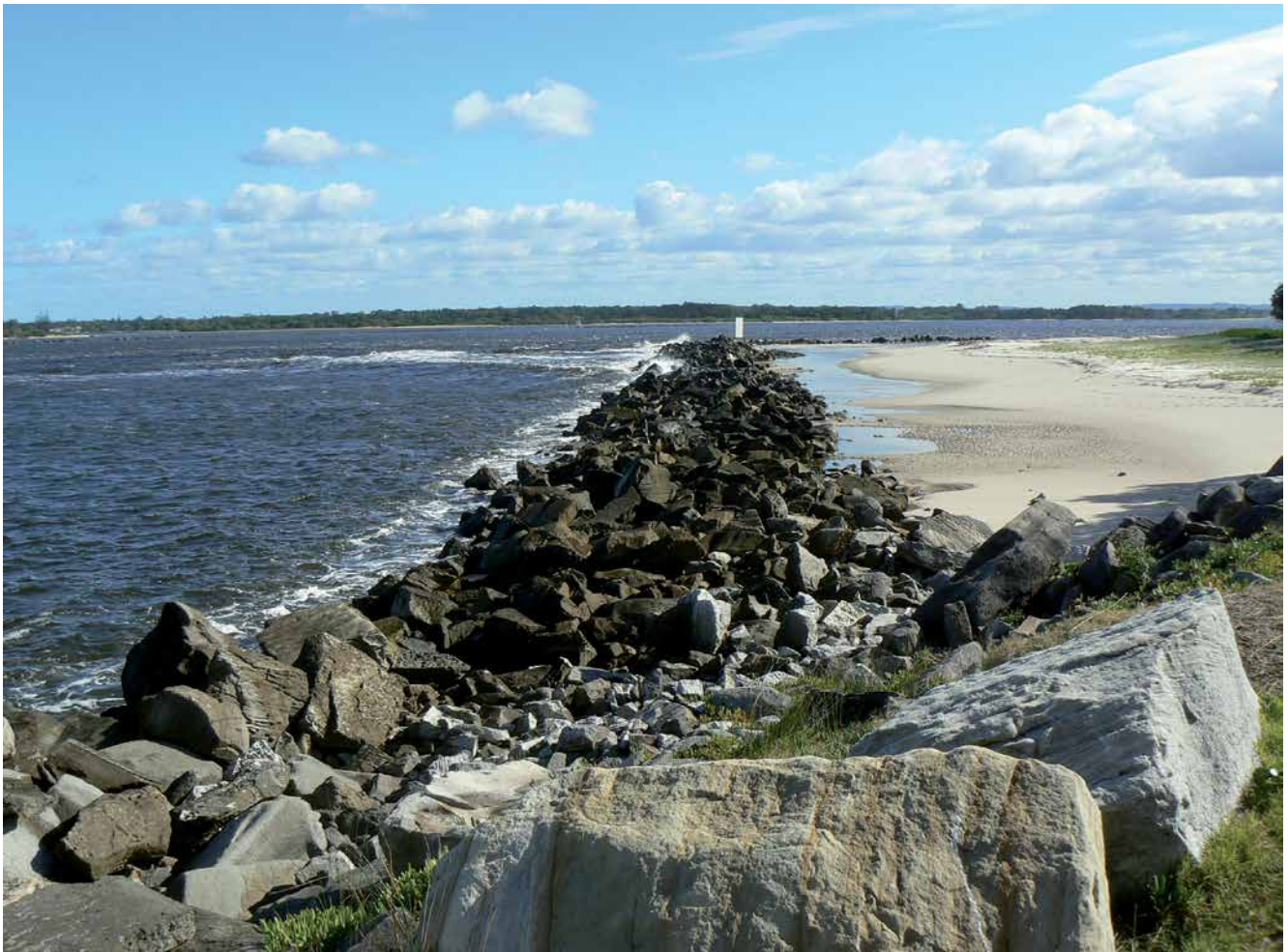
Moriarty's secondary wall across the North Sand Spit was dismantled in the 1890s to provide stone for the replacement scheme. It was partly rebuilt in 1970 when hydraulic modelling demonstrated it was a necessary adjunct for river control. Photo: Ian McNeil
