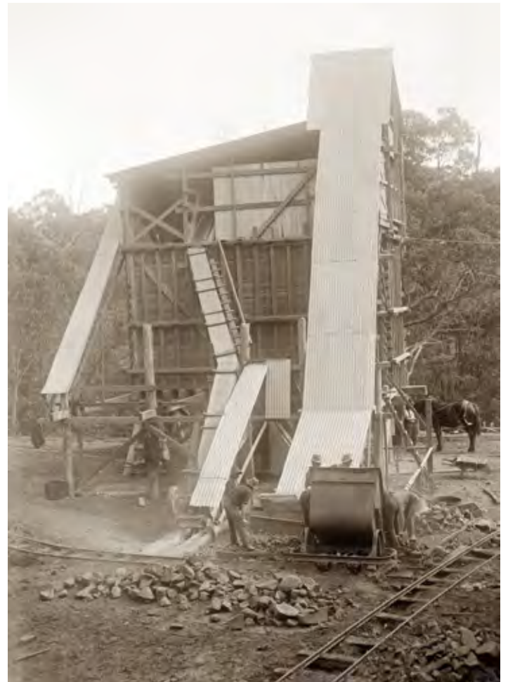
Top: The basalt quarry on 1 December 1922 showing the electrically-powered crusher and the internal track layout. There are three sets of points and at least four turntables, with spalls from the quarry face stacked ready for loading. Note the overhead lighting strung above the outlet tramway. State Library of Victoria image H2009.18/353, James Pinkerton Campbell. Above: Looking west past the crusher with a rake of skips under the loading hopper. State Library of Victoria image H2009.18/358, James Pinkerton Campbell. Right: Loading spalls into the crusher by hand. The skip in the foreground bears a distinctive oval plate showing it to be manufactured by George Fredrick Sewell at his Manchester Ironworks, West Footscray. State Library of Victoria image H2009.18/369, James Pinkerton Campbell.
