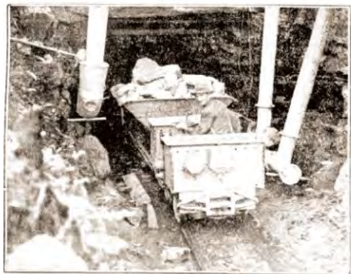
ONE OF THE FIVE-TON locomotives of the British Electric Vehicles Ltd., used to haul trucks of rock and earth from the tunnels driven through the hills for the outfall sewer.
