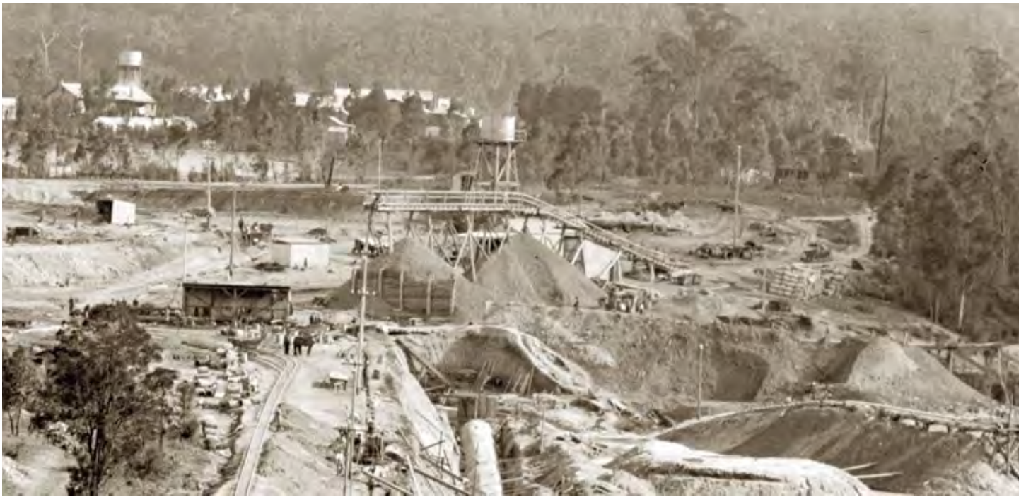
The incline trestle and stone dump at the tramway terminus, with the line to the quarry disappearing off into the bush to the right. State Library of Victoria image H2009.18/72, James Pinkerton Campbell.
