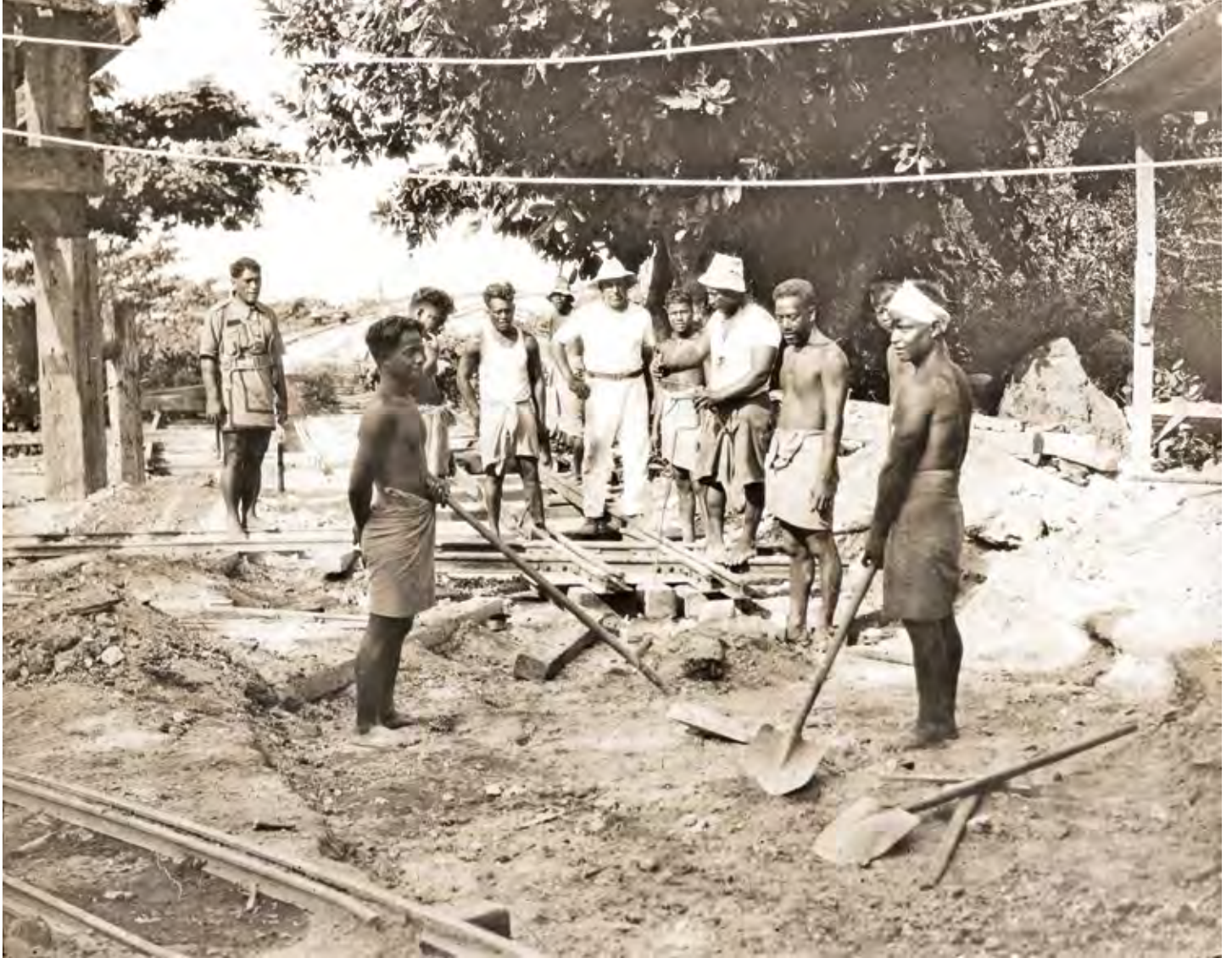
Above: Captioned by the good reverend as “Building the railway Nauru”. May be Ocean Island, date unknown; it is clearly a posed shot. A 2ft-gauge crossover has been fabricated, presumably in the workshops and is now being positioned to enable a new line to cross an existing line. A ‘pecking order’ seems to be in place – middle, in white hat is the Australian overseer, at left we have an islander, possibly a Banaban or Fijian wearing the local police’s uniform; right, also in hat is an islander wielding an auger to drill a hole in the sleeper, surrounded by eight islanders carefully noting the finer points of shovel work and railway construction. Overhead we seem to have the timbers of a bridge on one of the inclines. Photo: UoN refA5051-056.
