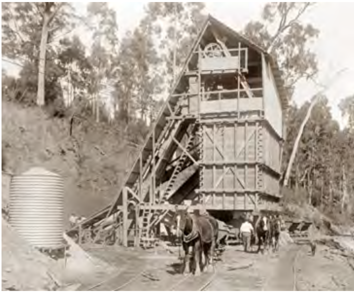
Top: The basalt quarry on 1 December 1922 showing the electrically-powered crusher and the internal track layout. There are three sets of points and at least four turntables, with spalls from the quarry face stacked ready for loading. Note the overhead lighting strung above the outlet tramway. State Library of Victoria image H2009.18/353, James Pinkerton Campbell. Above: Looking west past the crusher with a rake of skips under the loading hopper. State Library of Victoria image H2009.18/358, James Pinkerton Campbell. Right: Loading spalls into the crusher by hand. The skip in the foreground bears a distinctive oval plate showing it to be manufactured by George Fredrick Sewell at his Manchester Ironworks, West Footscray. State Library of Victoria image H2009.18/369, James Pinkerton Campbell.
