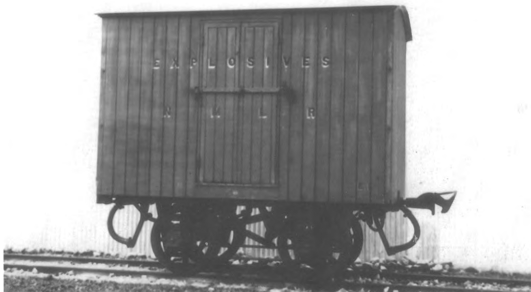
4-wheel explosives van, E-class No. 1, was built on the underframe of a Hurst Nelson hopper wagon c.1902. State Archives, courtesy Lou Rae
