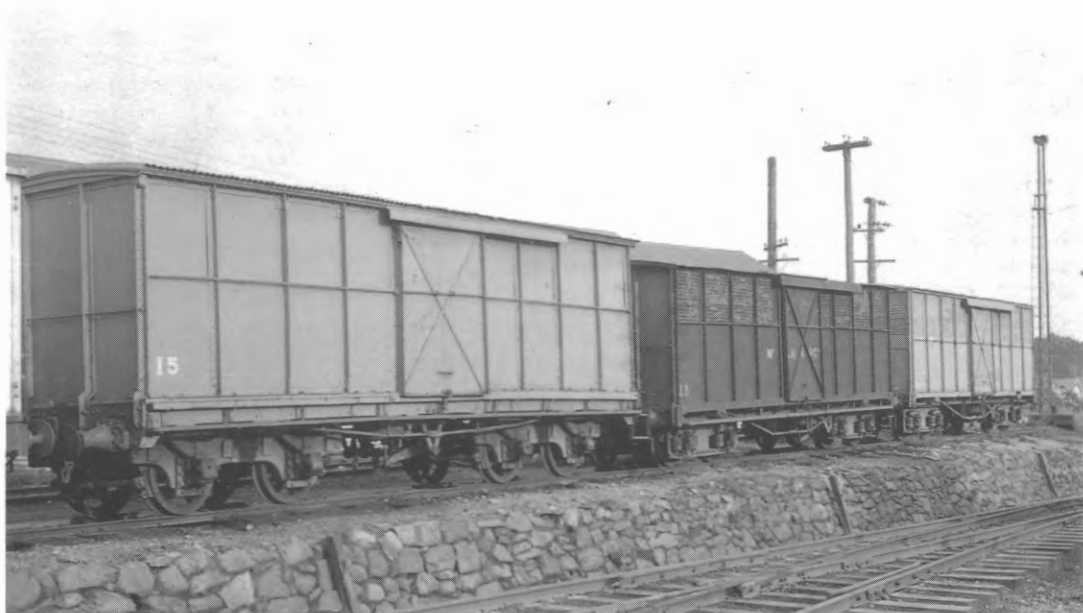
Mt Lyell steel bogie vans Nos. 15, 13 and 11 at Queenstown in 1963. No.15 was built on the underframe of a NMLR bogie open wagon from the Bristol Carriage & Wagon Company. Photo: HJW Stokes
