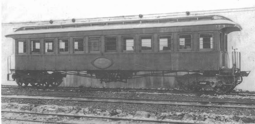
Composite passenger carriage built by the Metropolitan Railway Carriage & Wagon Company in 1899. Of interest is the unusual bogie design and the American styling. State Archives, courtesy JL Buckland
