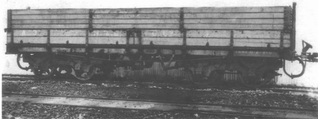
This neat 25 ton bogie open wagon was fitted with an extension frame to make it suitable for the carriage of coal and coke. State Archives, courtesy Lou Rae
