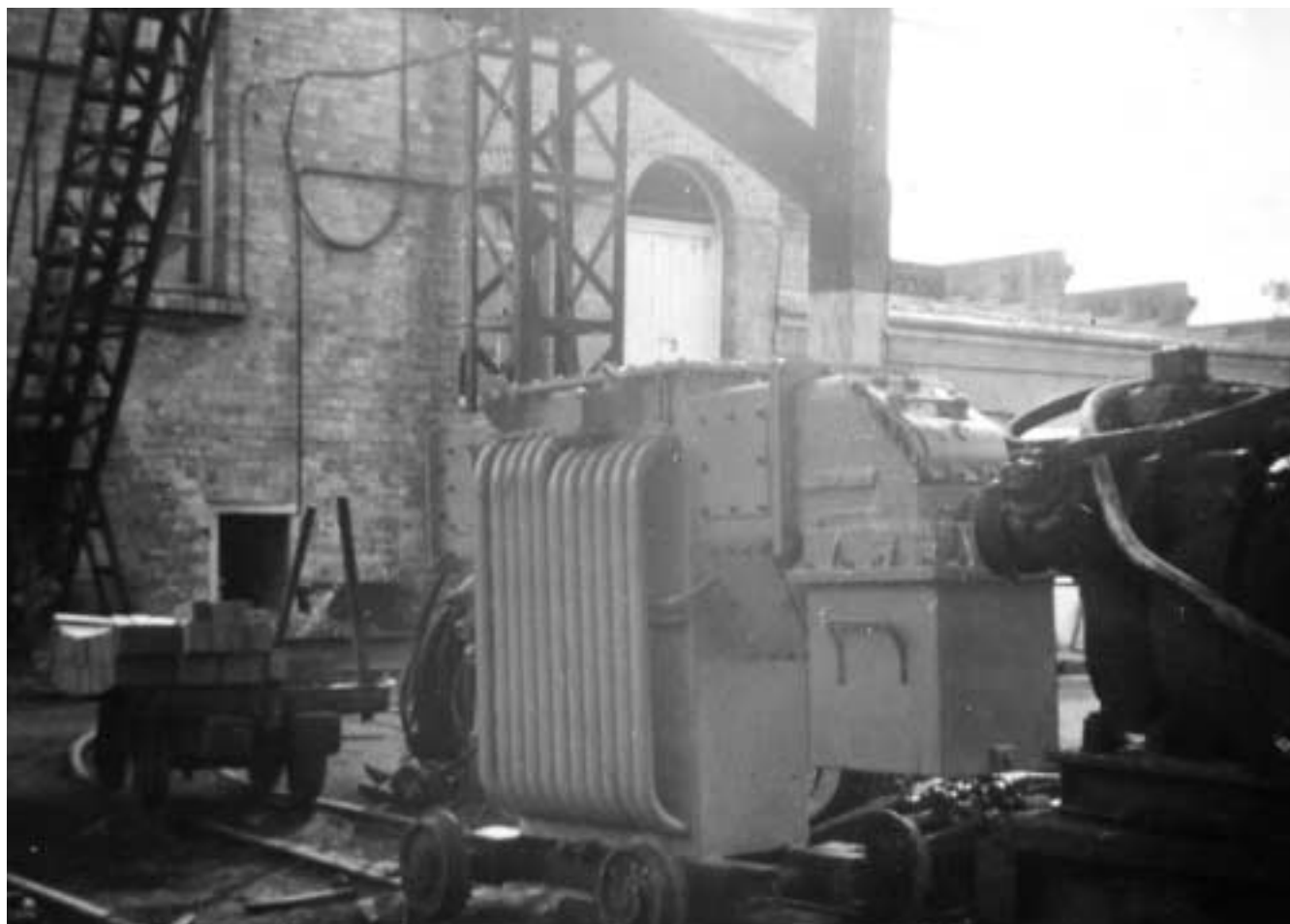
At ground level in August 1962, a variety of specialised rolling stock (from left): a 2ft gauge flat top loaded with bricks, a 3ft 6ins gauge rail mounted transformer, and a 3ft 6ins gauge flat top with air compressor.
