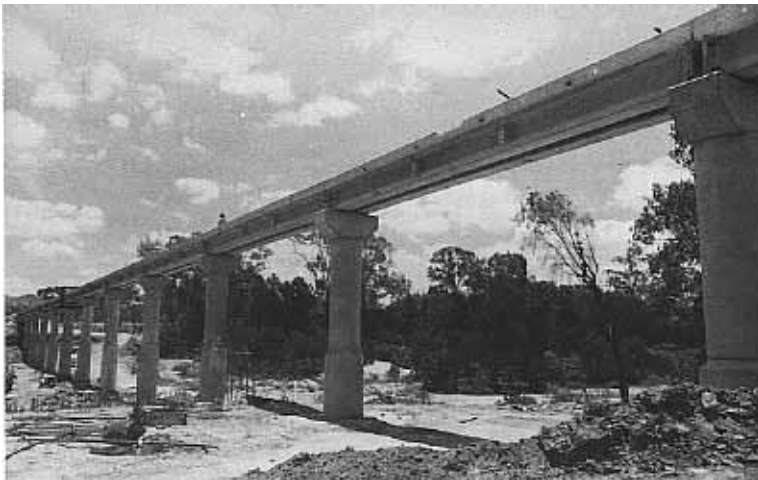
Invicta Sugar Mill, Giru Qld: 200 metre 13 span pre-stressed concrete bridge on the new 610 mm gauge tramway to Dalbeg.
