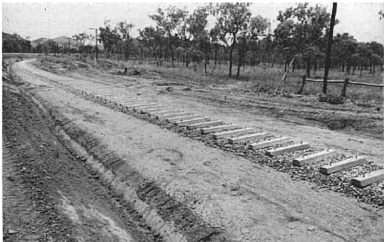
Invicta Mill, Giru: Concrete sleepers laid out between Clare and Millaroo.
