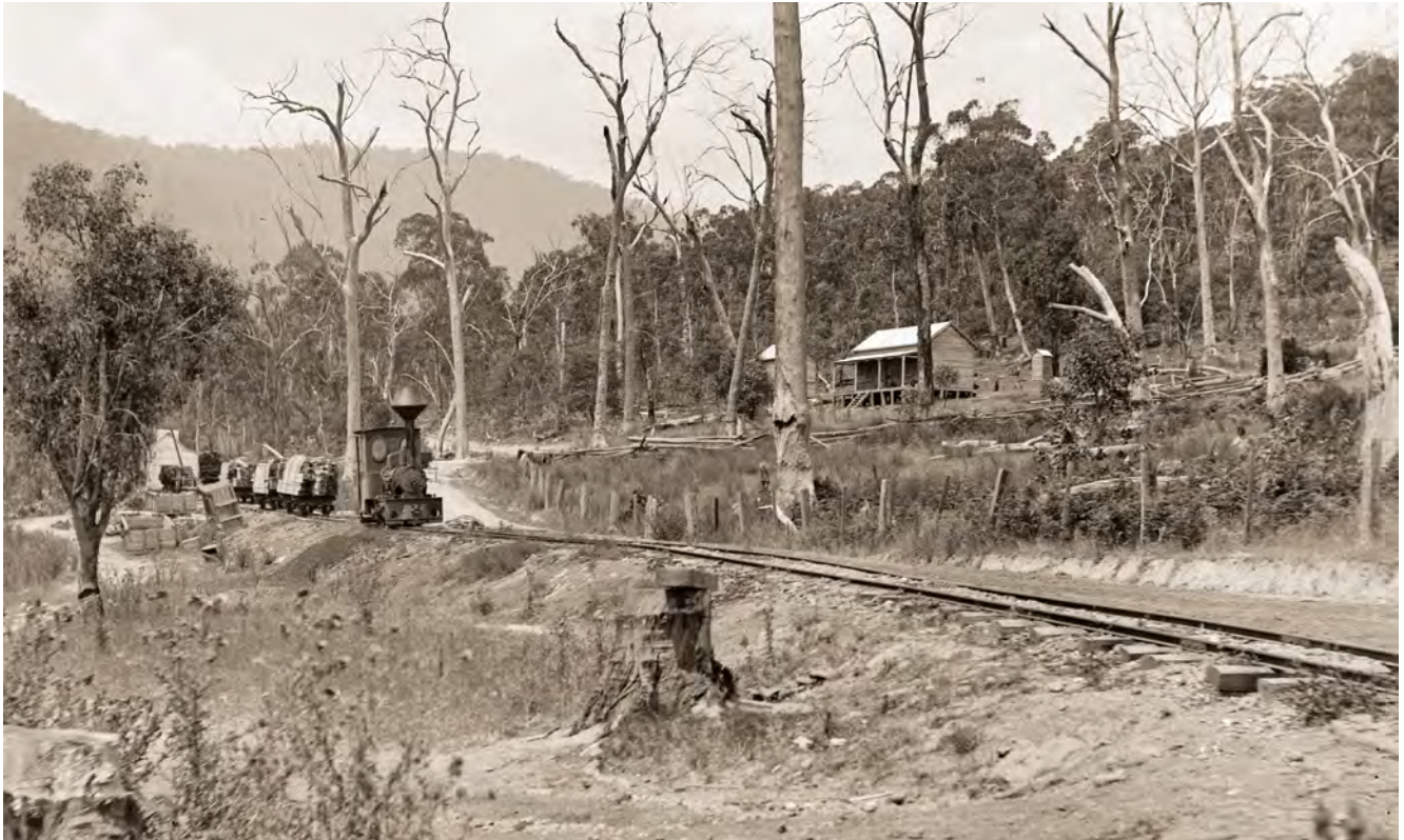
Above and below: The Depot, so-called as it was where timber from the sawmills of both Clark & Kidd and the Rubicon Lumber & Tramway Co was transferred from Clark & Kidd's 3ft 4½in-gauge wooden-railed tramway to the Lumber Company's 2ft-gauge steel-railed tramway for the remaining 12½ miles to Alexandra railway station. On a fine warm summer's day, our photographer, Lin Cumming, records the Lumber Co's No.1 locomotive, a Krauss (b/n 2459/1891) resting at its usual ashpan-raking spot while its train is prepared. Photo: SLV H2011.136/11
