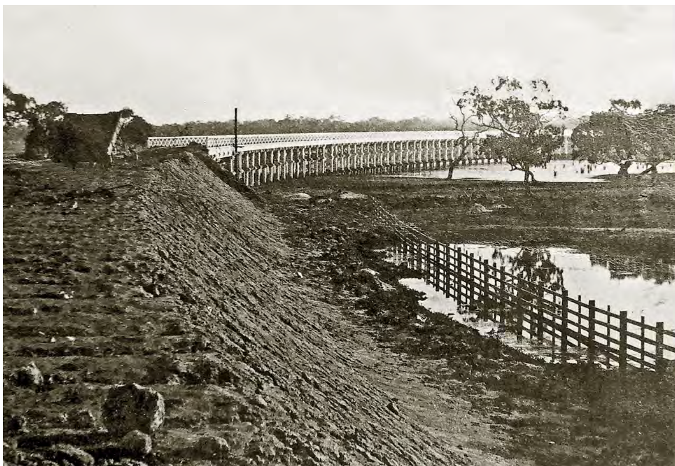
Former St Kilda and Brighton loop-line railway embankment and bridge near St Kilda station. For a line that was only used for three years an enormous amount of effort was put into building the extensive embankments and bridges. Source: Haig Collection, Newport Railway Museum. N0116a
