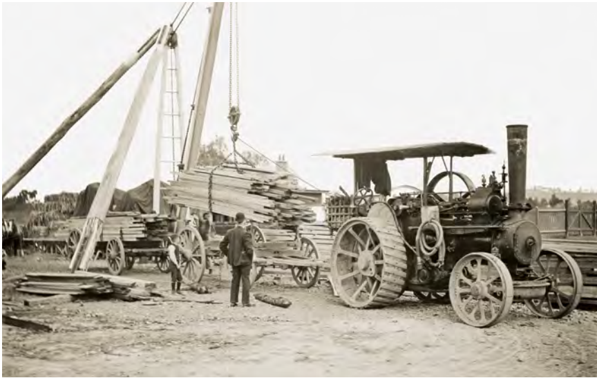
Left: Prior to the building of the Lumber Company's 2ft-gauge steel tramway from Alexandra to the forest's edge, where Clark & Kidd's wooden-railed tramway ended, the partners were using a 'light' Fowler traction engine for timber haulage to the railway station. Initially that was to Alexandra Road station, some 17 miles from their timber depot, but in 1909 the Victorian Railways extended the railway by 4½ miles, into Alexandra town where this photo was taken. Photo: State Library of Victoria H2005.88/23
