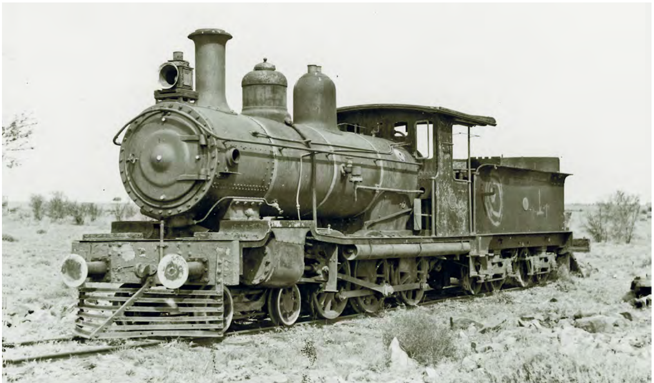
The Shire’s second locomotive, A2, was this ex-QGR B15 308, built by Walkers Limited in 1897. B15s were originally built with driving wheels just three feet in diameter but were soon re-built with 3ft 9in drivers, which put them into a useful mixed traffic category. B15 308 was sold to the shire in December 1915 for £2002 and was ‘converted’ to the larger wheels just before sale, which reclassified her to a B15 Con. Number 308’s arrival ended a long string of hired locomotives, none of which has been found successful bar one – a PB15. The second-hand B15, a predecessor of the PB15, was a useful stop-gap pending the purchase of a brand-new locomotive nine years later, at which time No.308 was renumbered A2. In 1943, needing a new boiler, it was taken out of service as soon as A1 received its new boiler. In August 1949 A2 was offered for sale. It is seen here at Aramac in January 1957 prior to being sold for scrap in 1958. Photo courtesy: late Ron Preston
