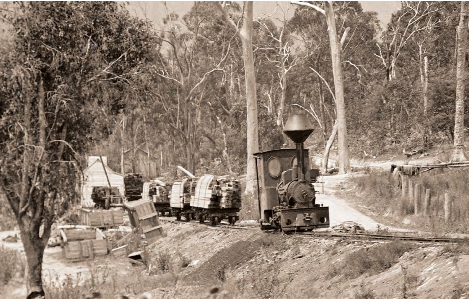
Above and below: The Depot, so-called as it was where timber from the sawmills of both Clark & Kidd and the Rubicon Lumber & Tramway Co was transferred from Clark & Kidd's 3ft 4½in-gauge wooden-railed tramway to the Lumber Company's 2ft-gauge steel-railed tramway for the remaining 12½ miles to Alexandra railway station. On a fine warm summer's day, our photographer, Lin Cumming, records the Lumber Co's No.1 locomotive, a Krauss (b/n 2459/1891) resting at its usual ashpan-raking spot while its train is prepared. Photo: SLV H2011.136/11
