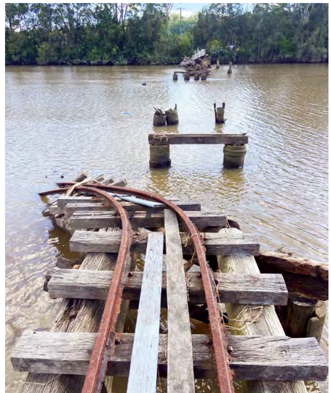
Below: Remains of the bridge after the 2022 floods. Photo: Clive Plater
