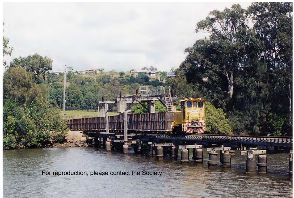
Locomotive Moreton hauls a rake of empty wagons across the Maroochy River bridge on 17 September 2002. Photo: Brian Webber
