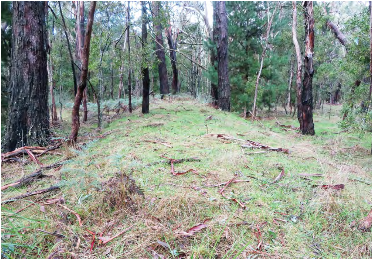
Typical formation 750 metres along the timber siding showing the 4.3 m wide formation. Photo: Norman Houghton
