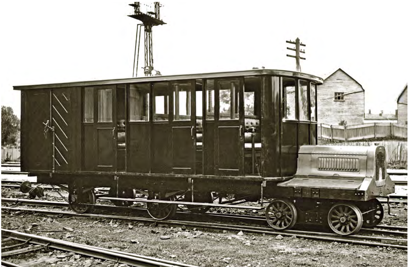
Construction of the third passenger rail motor started in 1917, designed to be larger and more powerful than the previous motors. Fitted with a 25-30hp Argyll engine (often misspelled as 'Argyle'). The engine was a product of Argyll Motors Ltd, Scotland) the rail motor was to seat from 16 to 20 persons with three sliding doors on each side plus a lockable luggage and mail compartment at the rear. Unfortunately the Argyll suffered a series of troubles – for instance in late 1919 Burnie advised the Melbourne directors that the vehicle was suffering from cylinder cracking. Photo: E A Winter, Weekly Courier 30 September 1920. Ted Lidster colln. courtesy Trainiac, Flickr
