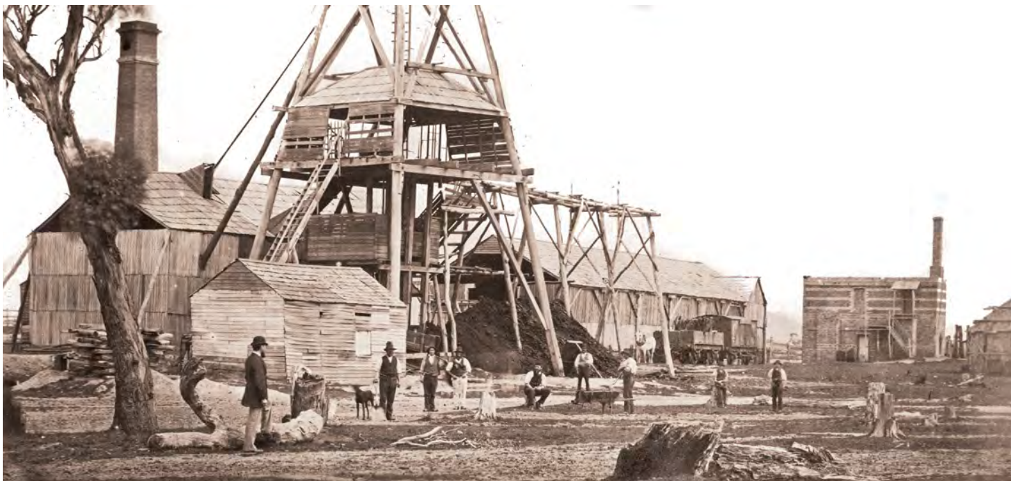
The Victorian Brown Coal Coy's lignite mine at Lal Lal circa 1882. A broad-gauge tramway has been laid from the VR boundary for nine chains [181.5 m] to the mine, with a horse leading a wooden-bodied I-class wagon loaded with timber, and what appears to be an H-class van trailing. The engine house is to the left, with an elevated tramway from the brace level of the poppet-head being used to dump lignite. This elevated tramway originally extended to the brick drying kiln in the distance (by this time disused). The large building between the engine house and the kiln is used to air-dry and store lignite undercover. Photo: Frederick Kruger, State Library of Victoria image H39614/31
