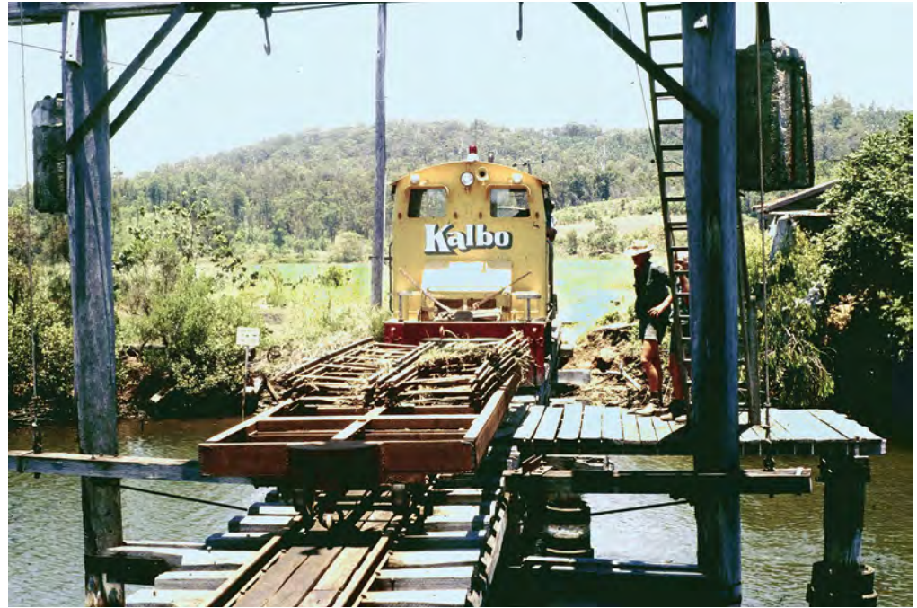
Com-Eng locomotive Kalbo eases across the lift span with a maintenance train as the bridge crew watches on 11 December 1979. Photo: John Browning
