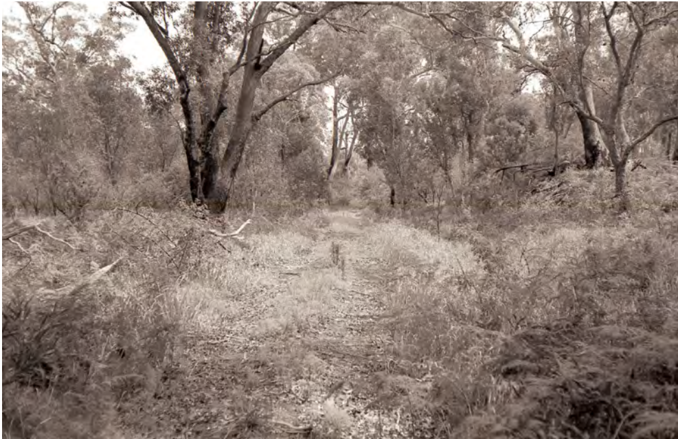
Looking along the formation from Tomago Road towards the river. Photo: Peter Sansom
