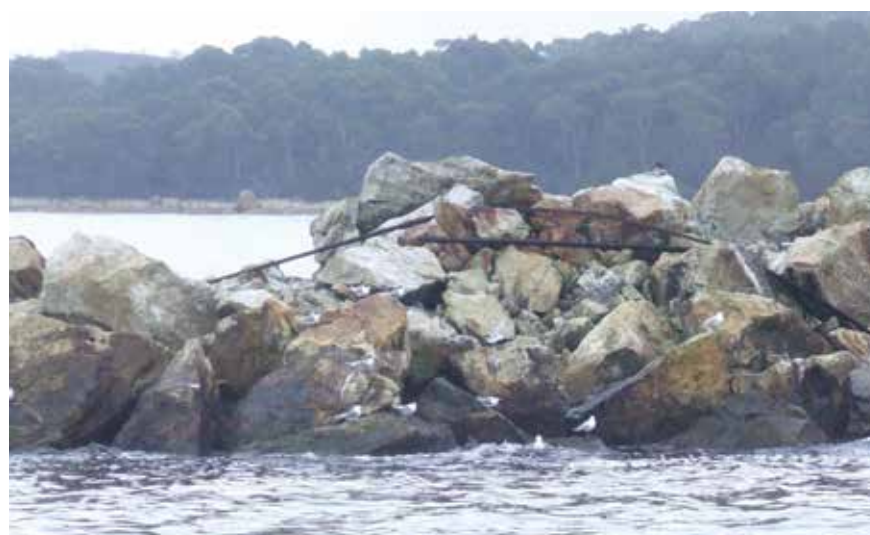
Hells Gates breakwater, showing the remains of the construction railway
