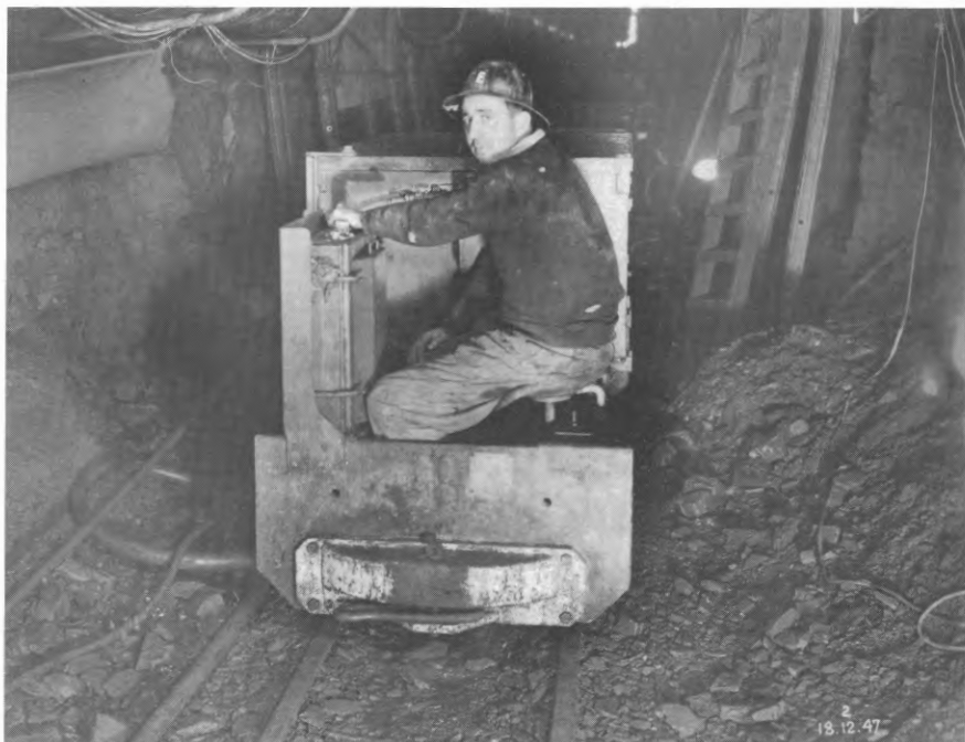
Below: A battery electric loco at the face of the tunnel. 18 Dec 1947.
