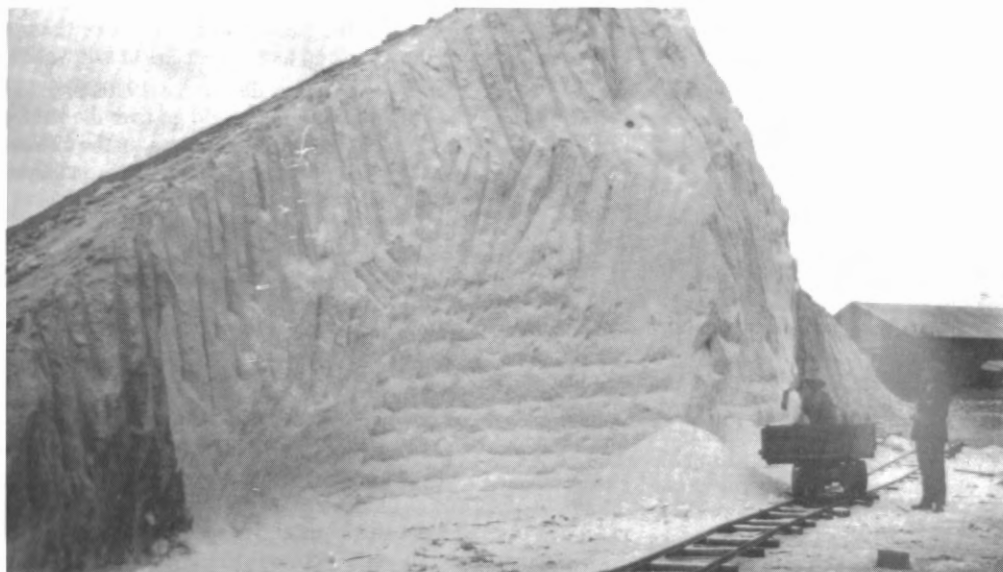
Barring down from the continuous salt stack into the tramway dobbin. 1930.
