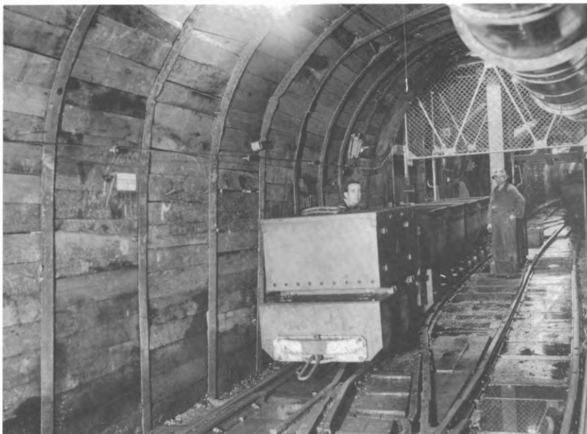
One of the battery electric locos at the plat with the safety gates raised. 18 Dec 1947.
