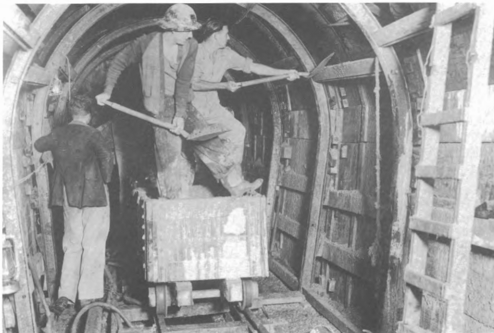
Filling the tunnel overbreak with concrete.
