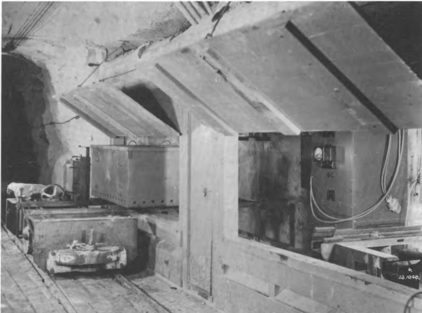
Battery charging arrangements for the locos. Shaft 7. Photo: Sydney Water Board.
