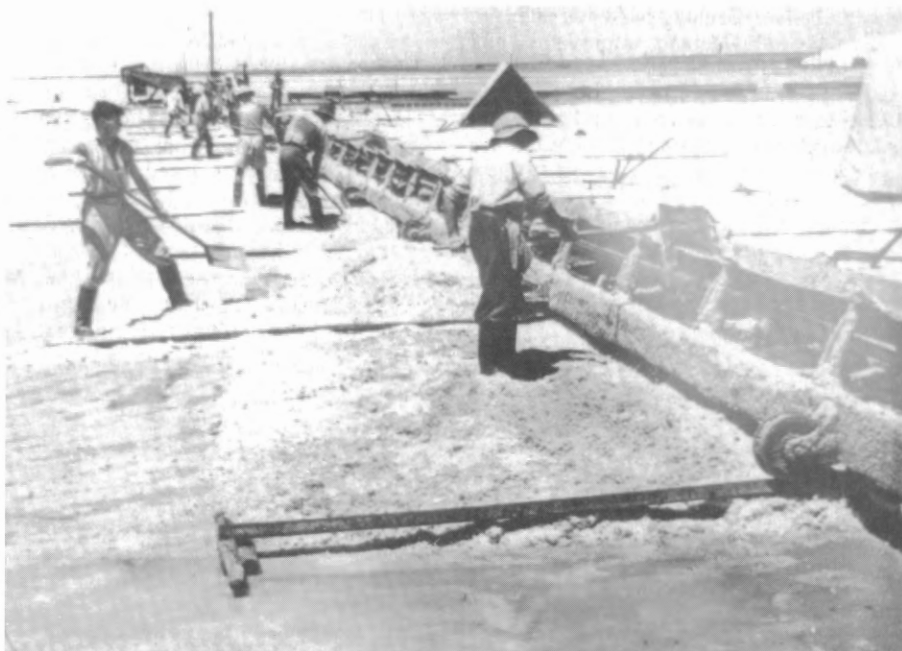
Shovelling salt onto the belt in the crystallisers prior to mechanisation in 1948.
