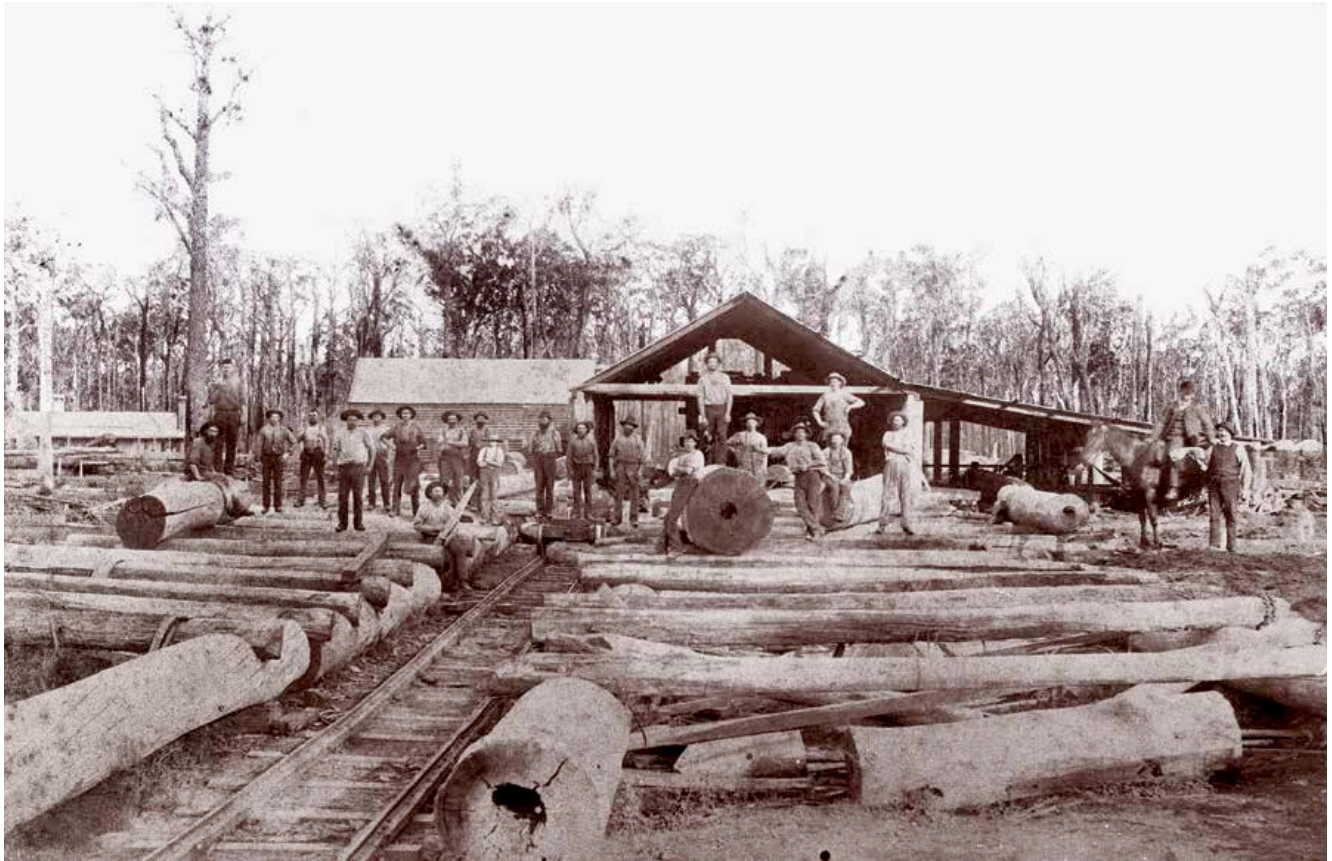
Mason and Moore's Nine Mile Creek sawmill c1891. Christopher and Elizabeth Mason's residence in left background and stables to the rear left of the mill. The log yard was configured to provide for log deliveries by tram on the left and deliveries by bullock and horse team on the right. The tramway passed through the shed and onwards to Port Welshpool.
