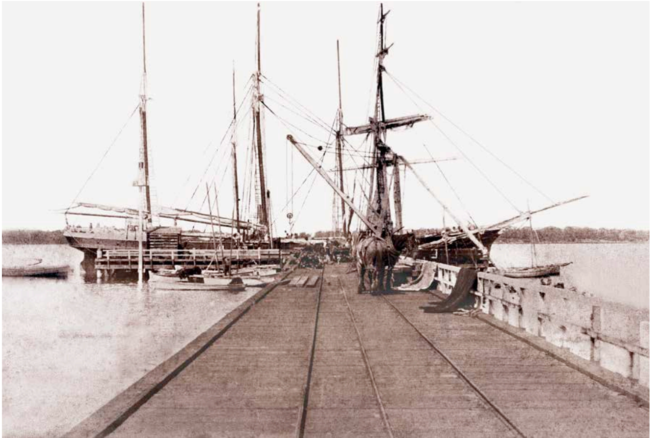
The government jetty at Port Welshpool c1891. There are two vessels tied up abreast in view. The nearer appears to be the Coquette, a regular trader to Port Welshpool. The jetty tramway, gauged to 5 ft. 3 in in anticipation of a connection to the Great Southern Railway, shares a common right hand rail with Mason's 3 ft. gauge tramway. Under the jib crane in middle distance, one of Mason's timber trucks awaits removal by the horses in the foreground. The Khartoum would have collected the assembled trucks in a siding positioned just off the jetty end. Photo: Late Beryl Atkins Collection
