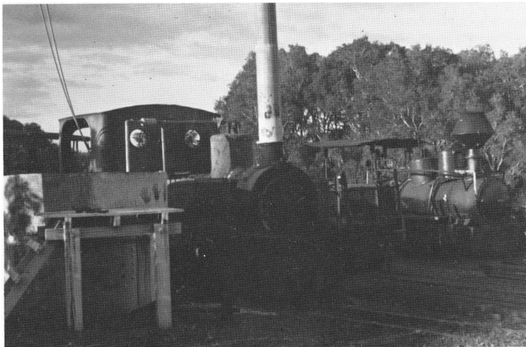
Torpedo (Decauville 245/1897) in use as stationary boiler at Cudgen. Sunlander is in the background.
