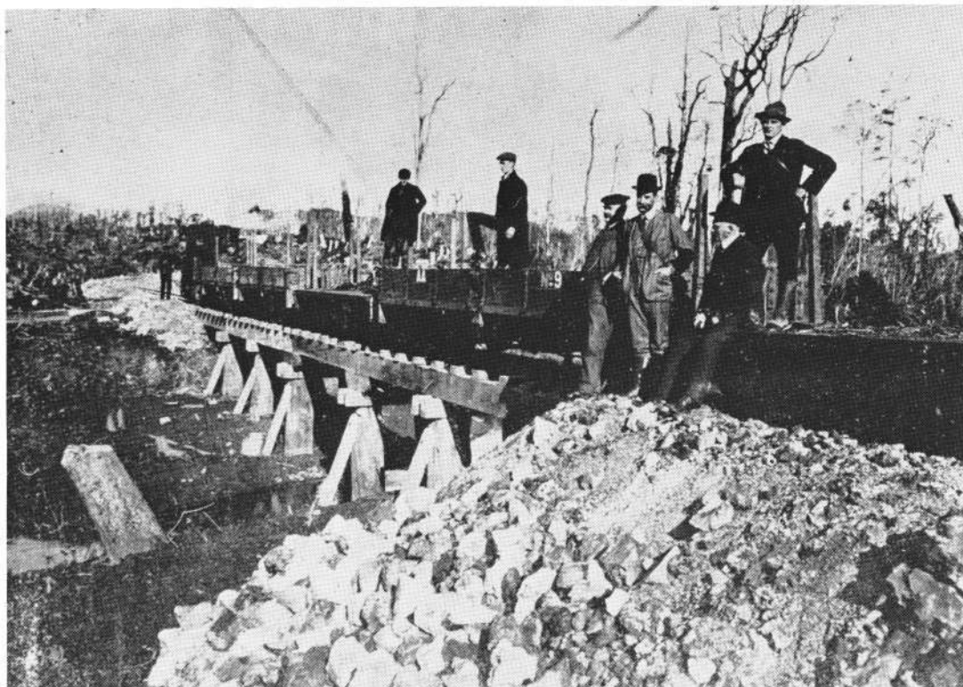
The branch line to Nickel Junction showing the bridge over Melba Creek in July 1910. Krauss locomotive H.4 (B/No 4080/1899) is on construction work.
