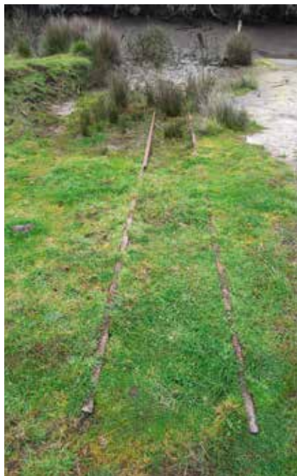
This 10m section of 610mm gauge track was clearly once used for launching fishing boats at Stockyard Creek. Judging from the heavy corrosion on the rails, it has been in situ for quite some time:
