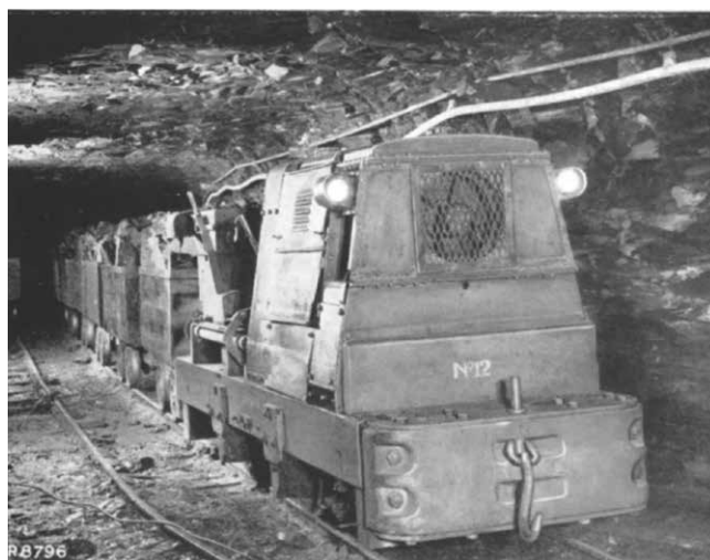
Ruston & Hornsby photograph of a 20DLU locomotive at work underground in the UK.
