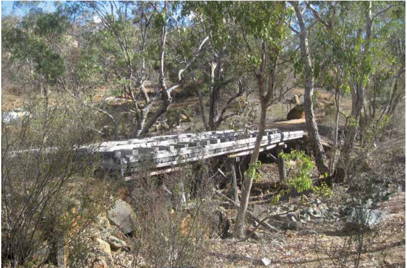
Side view on 26 April 2011 of the Munday Brook bridge on the Mason Bird Heritage Trail. It is reputed to still have elements of the original Mason & Bird tramway bridge in its foundations but has been substantially rebuilt. Munday Brook was dammed to form the Victoria Reservoir.
