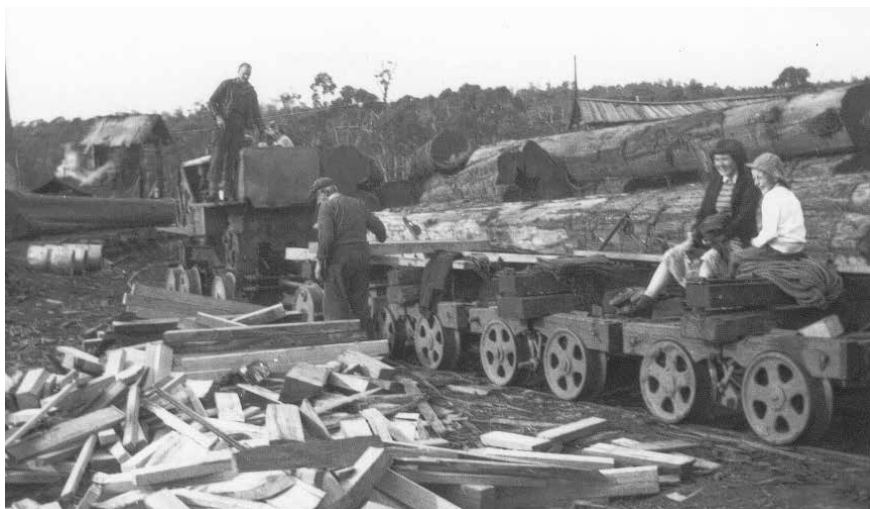
The Caterpillar had an unusual wheel arrangement, with a leading 4-wheeled bogie, a single rear wheelset, and a linked powered 4-wheeled log bogie. It is unclear which of the five axles were powered, but most likely all but the single rear wheelset. The two bogies were from the old Byers , but they had lost their rod linkages and gained chain linkages. The wheelsets on the following three log bogies were of a different pattern, and matched those of the background bogie shown in the colour photograph. Original unknown, from W Chenoweth collection
