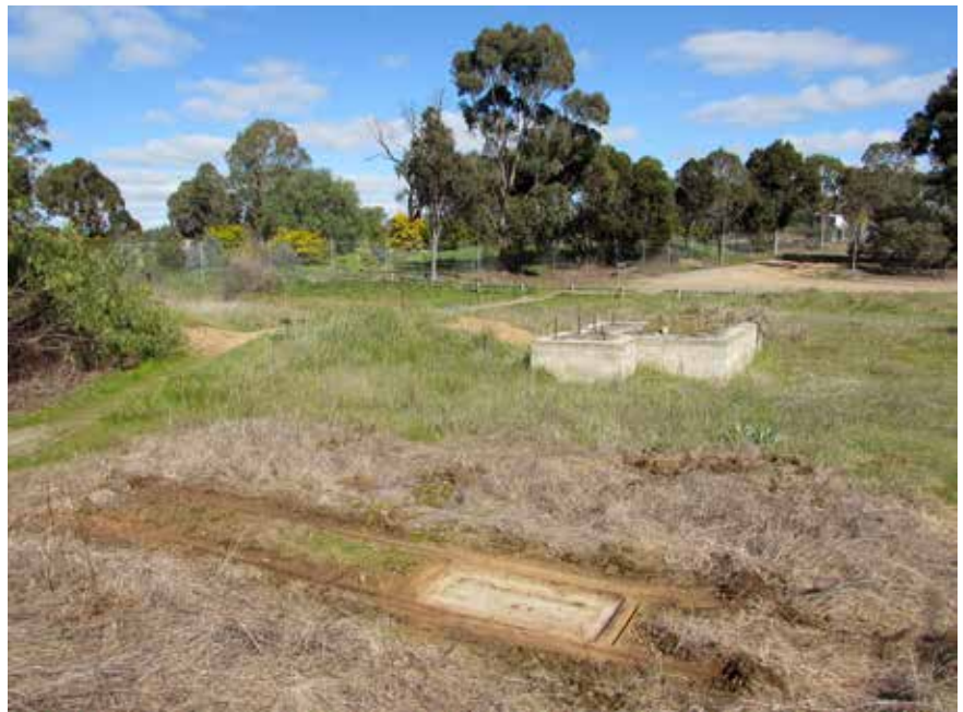
The extant track at the 'Old' Napoleon mine in the foreground with the winder foundations in the background.
