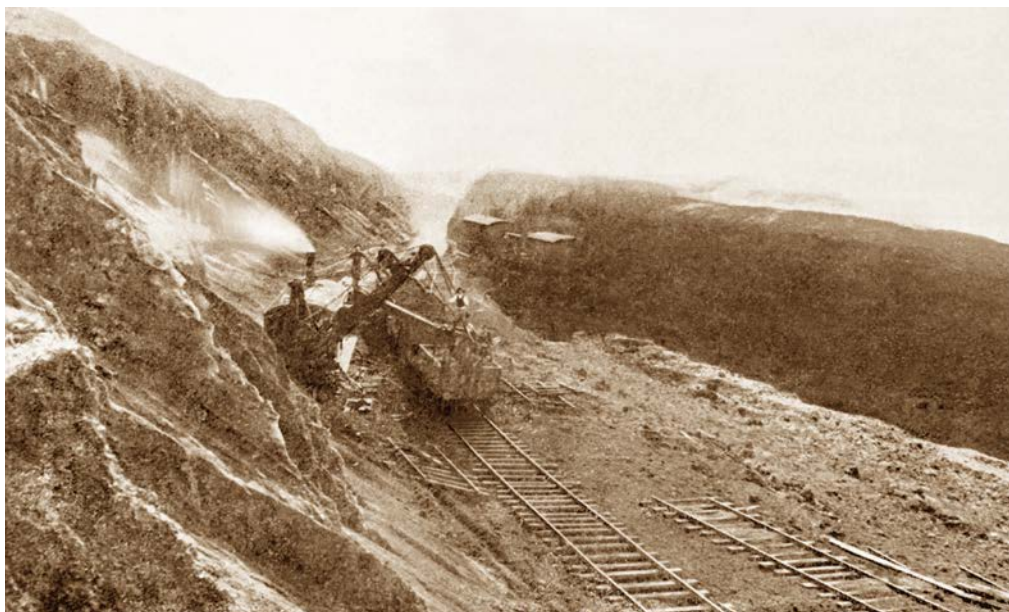
The Marion steam shovel at work in the pits loading rail trucks, circa 1910. The ballast line comes into the pit via the cutting in the background. The rails in the pit are in loose panels that are moved around as the cutting face advances. There is a short spur siding to the right and here are stabled three equipment and stores trucks for the shovel. Image courtesy John Thompson postcard collection.
