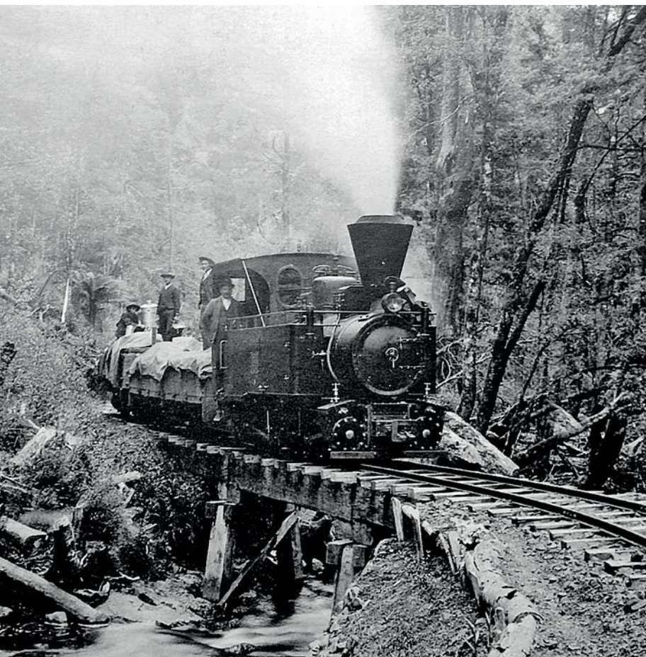
Above left: The Arthur River crossing at 3miles 25chains from the mine was a major structure on the line. It was from near there trains began the steep 5-mile "mountain section" of 142 curves, 71 of them under two chains radius, and with long gradients as steep as 1:25. Magnet No. 1, heading for Magnet Junction had come up the river gorge from the right to approach the bridge in a left-hand curve. It would then enter a right/left reverse curve to climb up the opposite side of the gorge before swinging away to the right after about a mile, and then running up to the summit through steep sideling country. Wikimedia Commons: Magnet tram (28416685446).jpg
