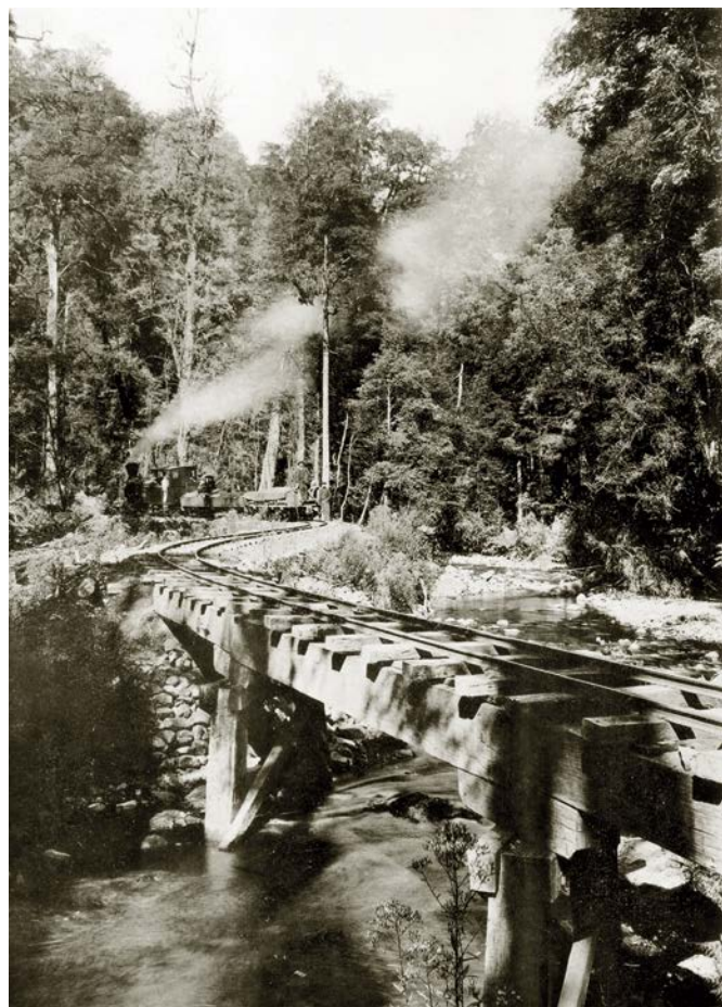
Above left: The Arthur River crossing at 3miles 25chains from the mine was a major structure on the line. It was from near there trains began the steep 5-mile "mountain section" of 142 curves, 71 of them under two chains radius, and with long gradients as steep as 1:25. Magnet No. 1, heading for Magnet Junction had come up the river gorge from the right to approach the bridge in a left-hand curve. It would then enter a right/left reverse curve to climb up the opposite side of the gorge before swinging away to the right after about a mile, and then running up to the summit through steep sideling country. Wikimedia Commons: Magnet tram (28416685446).jpg
