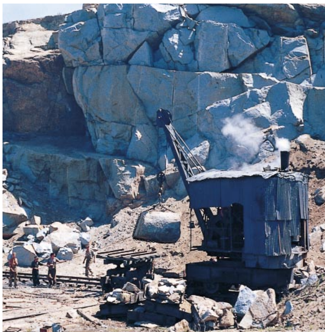
The Ruston steam crane loads a granite boulder onto a truck in the quarry. Photo: D.G. McKillop
