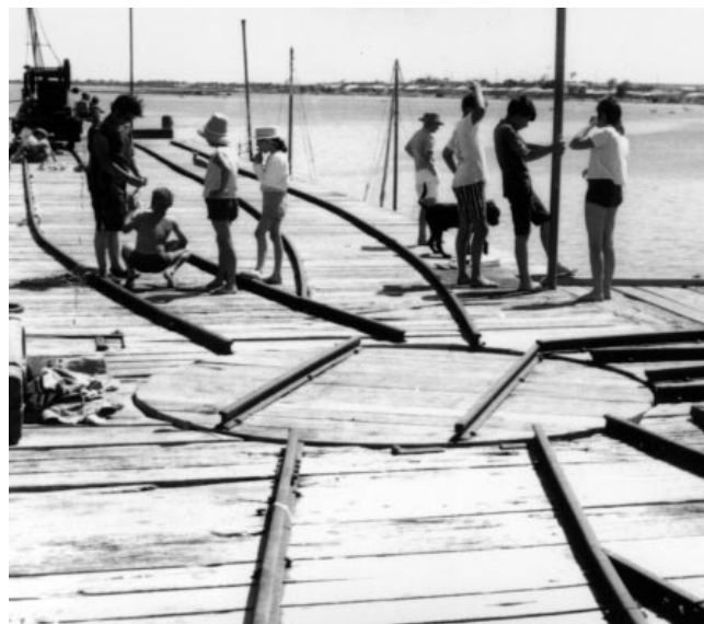
'T'-Head jetty at Port Broughton, showing trackwork, including turntable and moveable rails at the 'T'-Head, c.1964.
