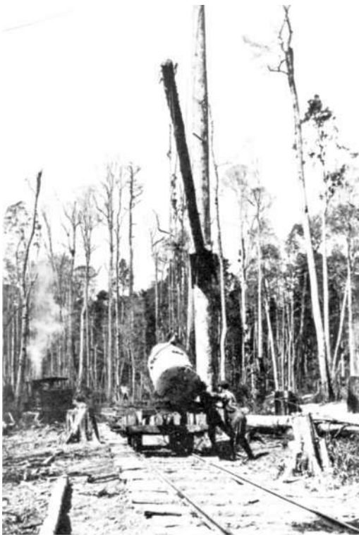
Loading logs onto a tramway truck at a logging depot on the Briggsvale tramway, September 1930. The loading jib is suspended from the spar tree which is used for "high lead" logging. Photo: FM Bailey, per NSW Forestry Commission
