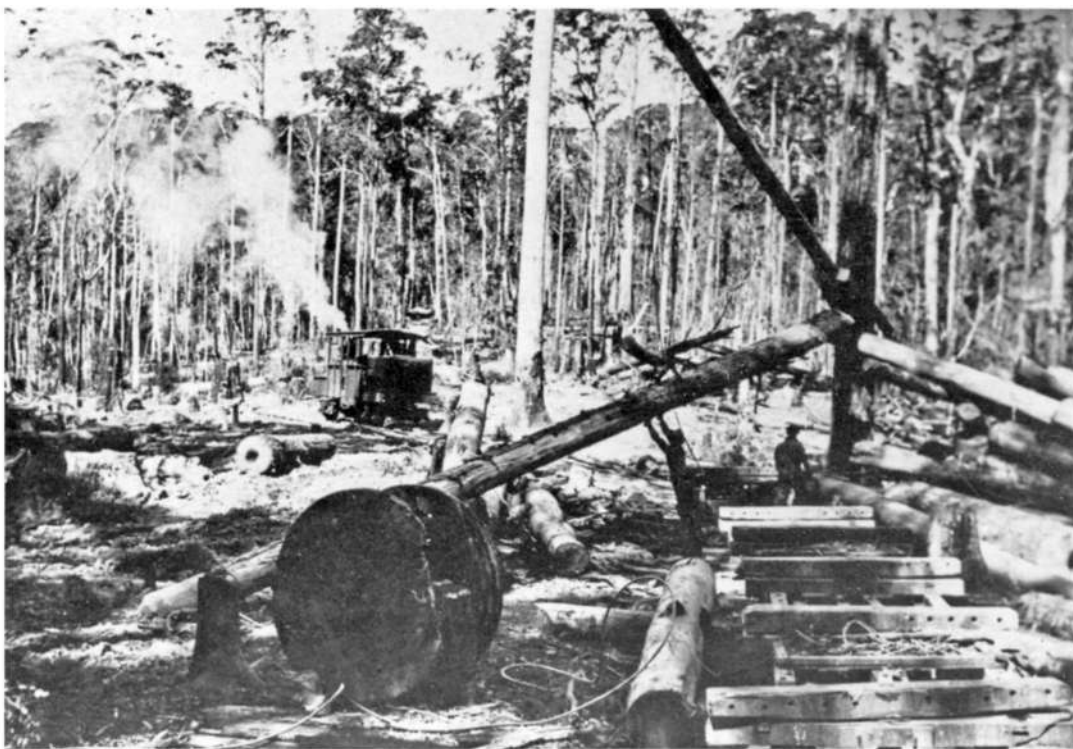
Log loading arrangements on the Briggsvale tramway. The "neutral" position of the loading job was over the centre of the tramway. Logs were lifted by a secondary steam winch driven off the main hauler. Photo: FM Bailey, per NSW Forestry Commission
