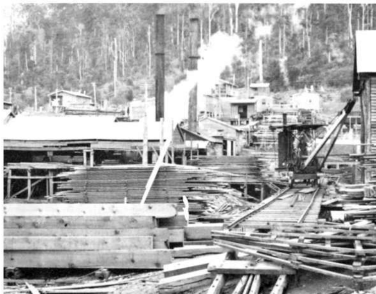
Briggsdale sawmill in September 1936, showing the small rail mounted steam crane. A NSWGR S-truck is on the mill siding behind.
