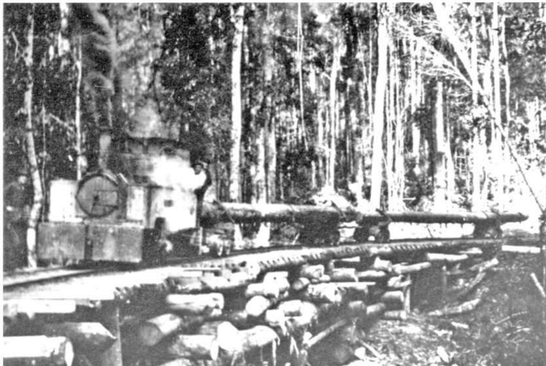
BEN BULLEN and a short logging train pose for the photographer on a small trestle bridge built "pig-sty" fashion on the Briggsvale tramway, circa 1927. Photo: NSW Forestry Commission
