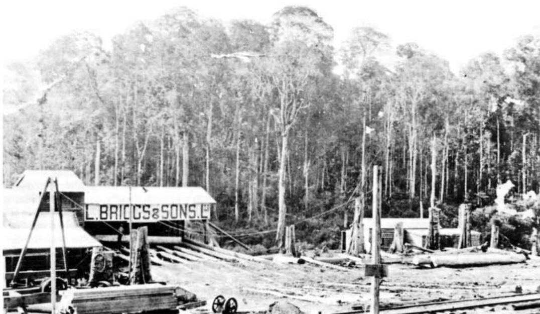
The Briggsvale mill and tramway in 1928. Logs were simply tipped off the tramway trucks and rolled to the mill.
