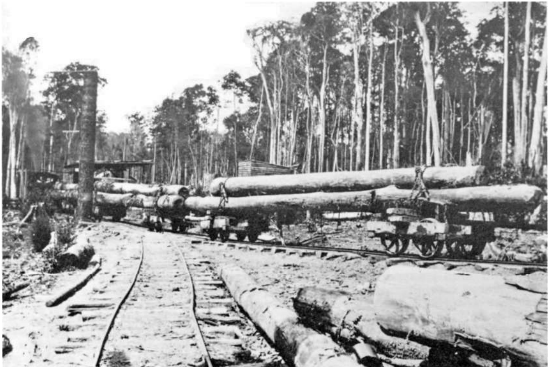
A log train on the Briggsvale tramway, September 1930. Note the light rails (approx 20 lbs/yd). Photo: FM Bailey, per NSW Forestry Commission
